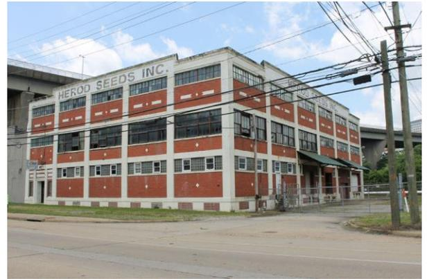
The Richmond complex also exemplifies the evolution of industrial buildings after the advent in the early 20<sup>th</sup> century of reinforced concrete. This development made possible construction of larger interior spaces, and more numerous and larger windows than the use of brick alone. The two types of construction methods are juxtaposed in the earlier warehouses and later portions of the complex and add to the interest of the building as a whole.
