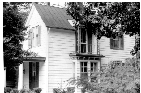
After application of synthetic siding.
