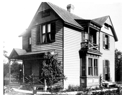
Before application of synthetic siding.
