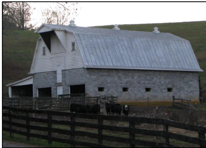
Figure 13- A gambrel-roofed barn (005-5075)
