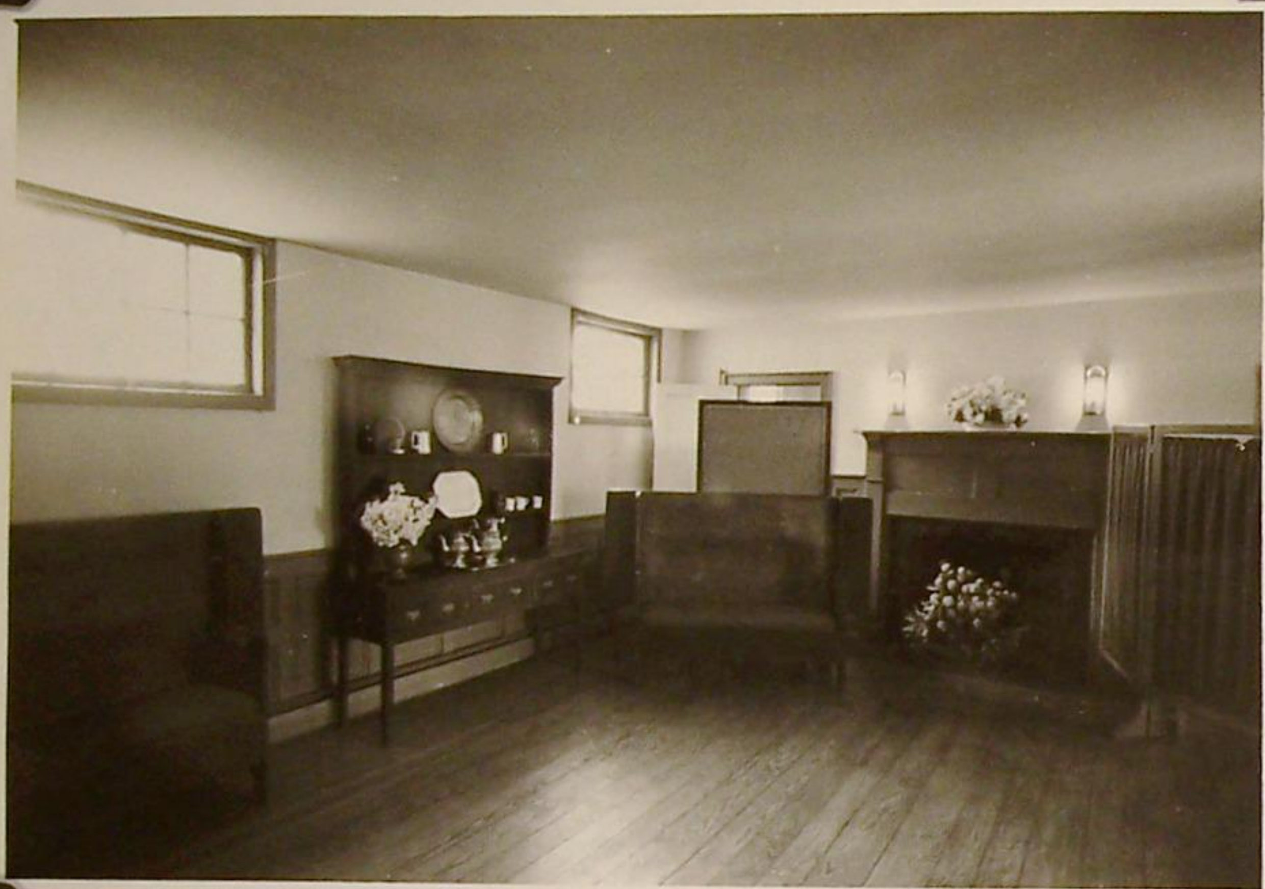
- Ground floor room -
