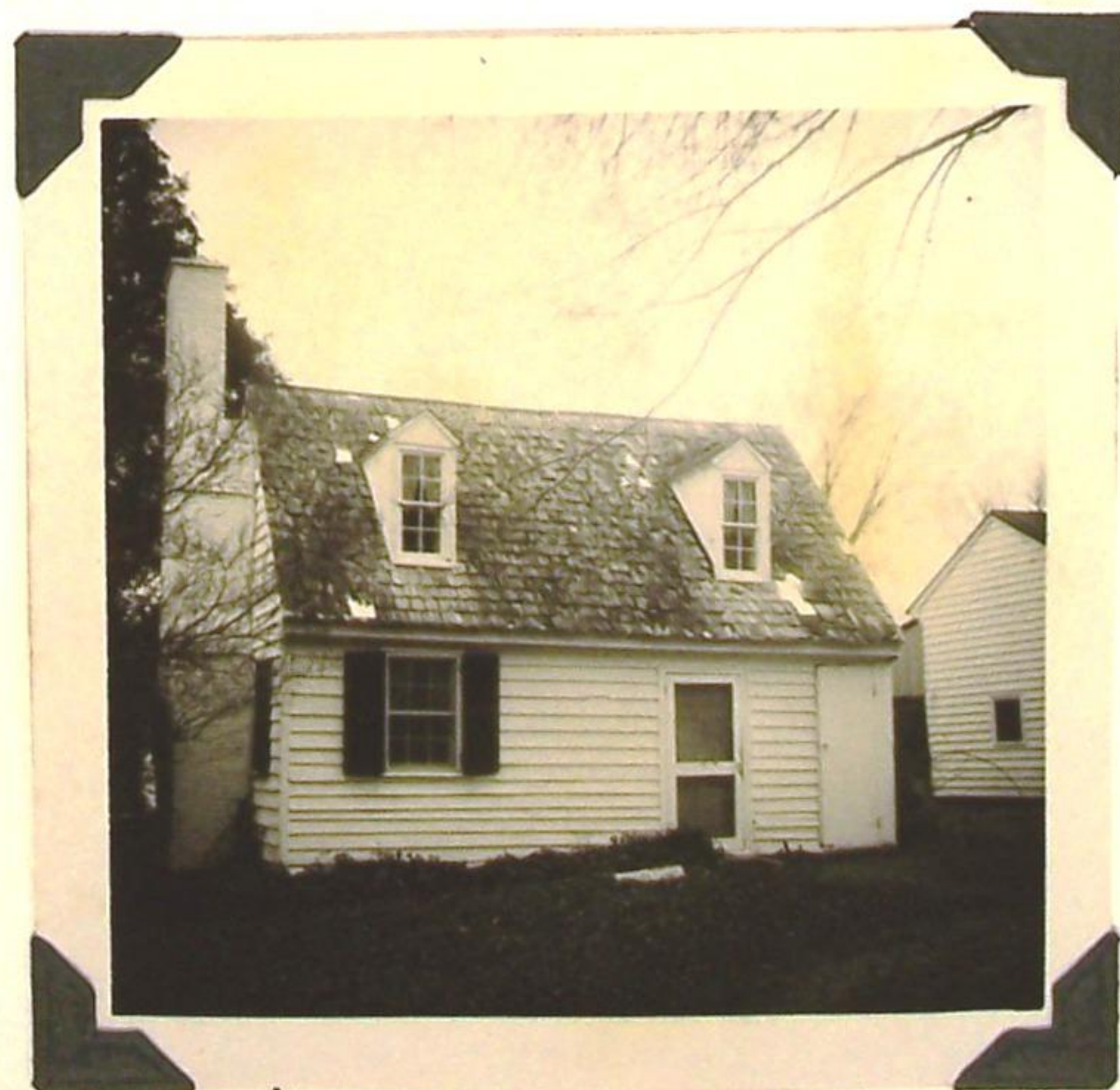
Kitchen - southeast facade the building appears to anti-date the house
