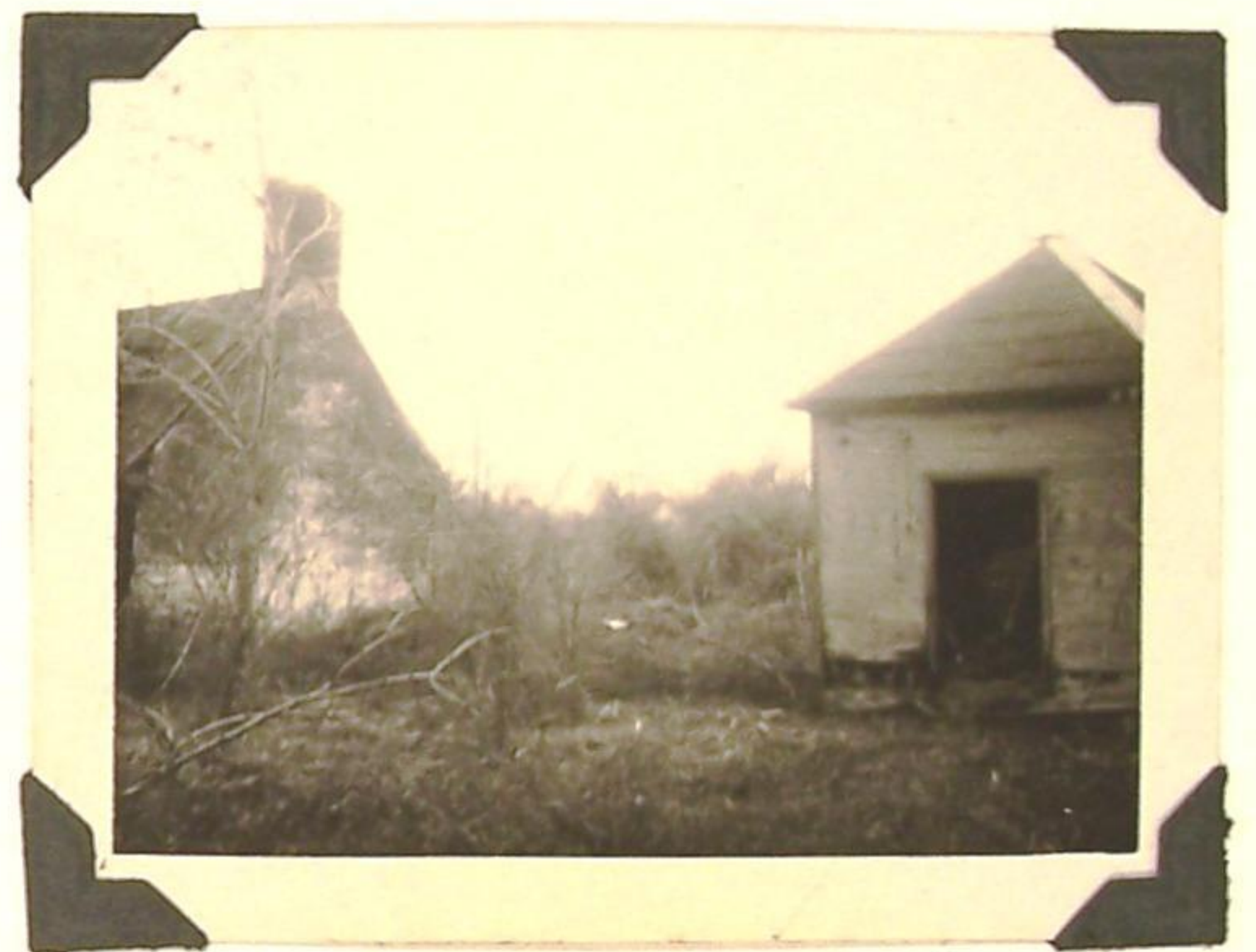
brick end of kitchen & Smokehouse
