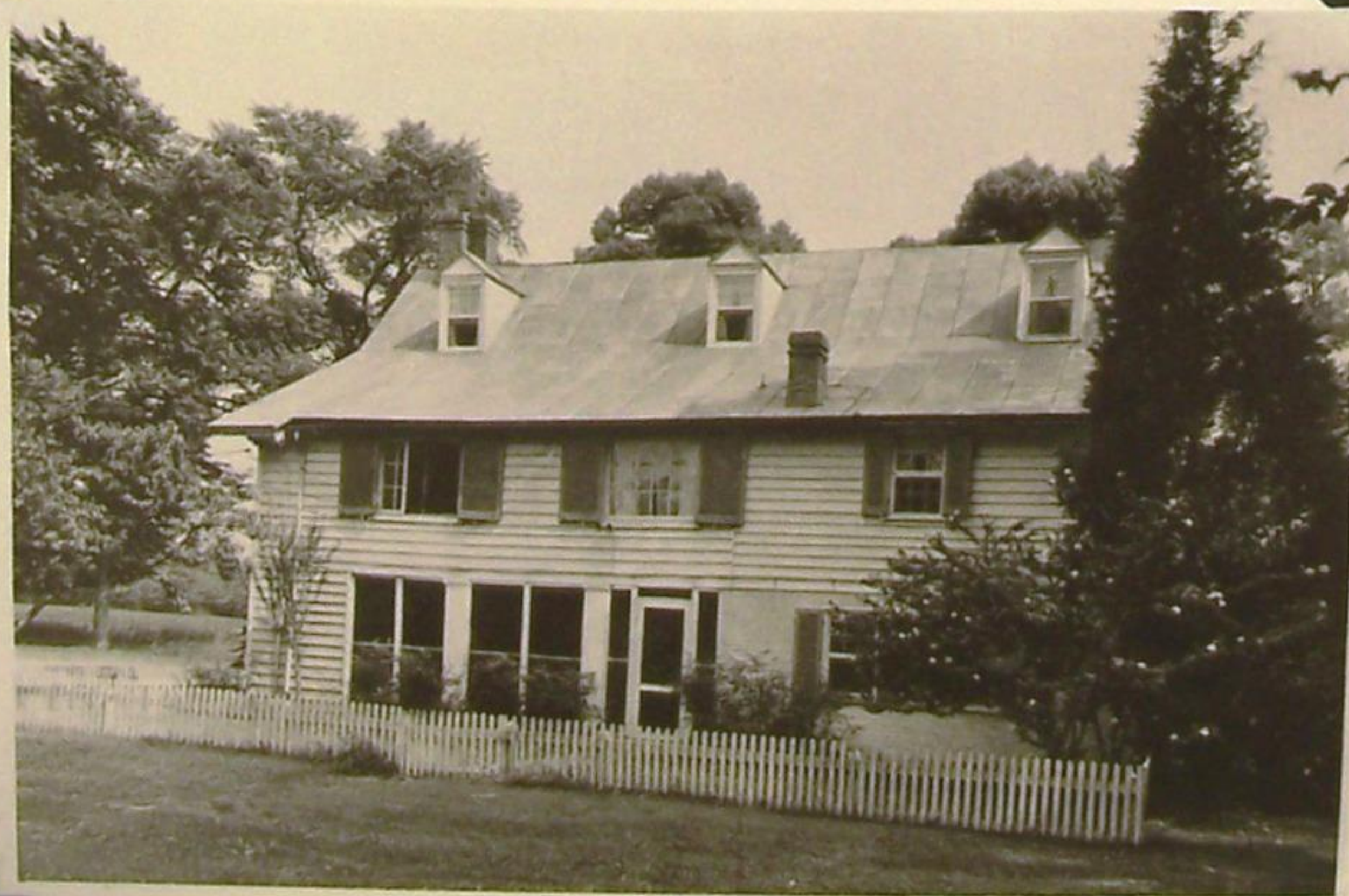
Northwest facade Photo 1950's This is the mid-18th century portion to which there has been a shed addition.
