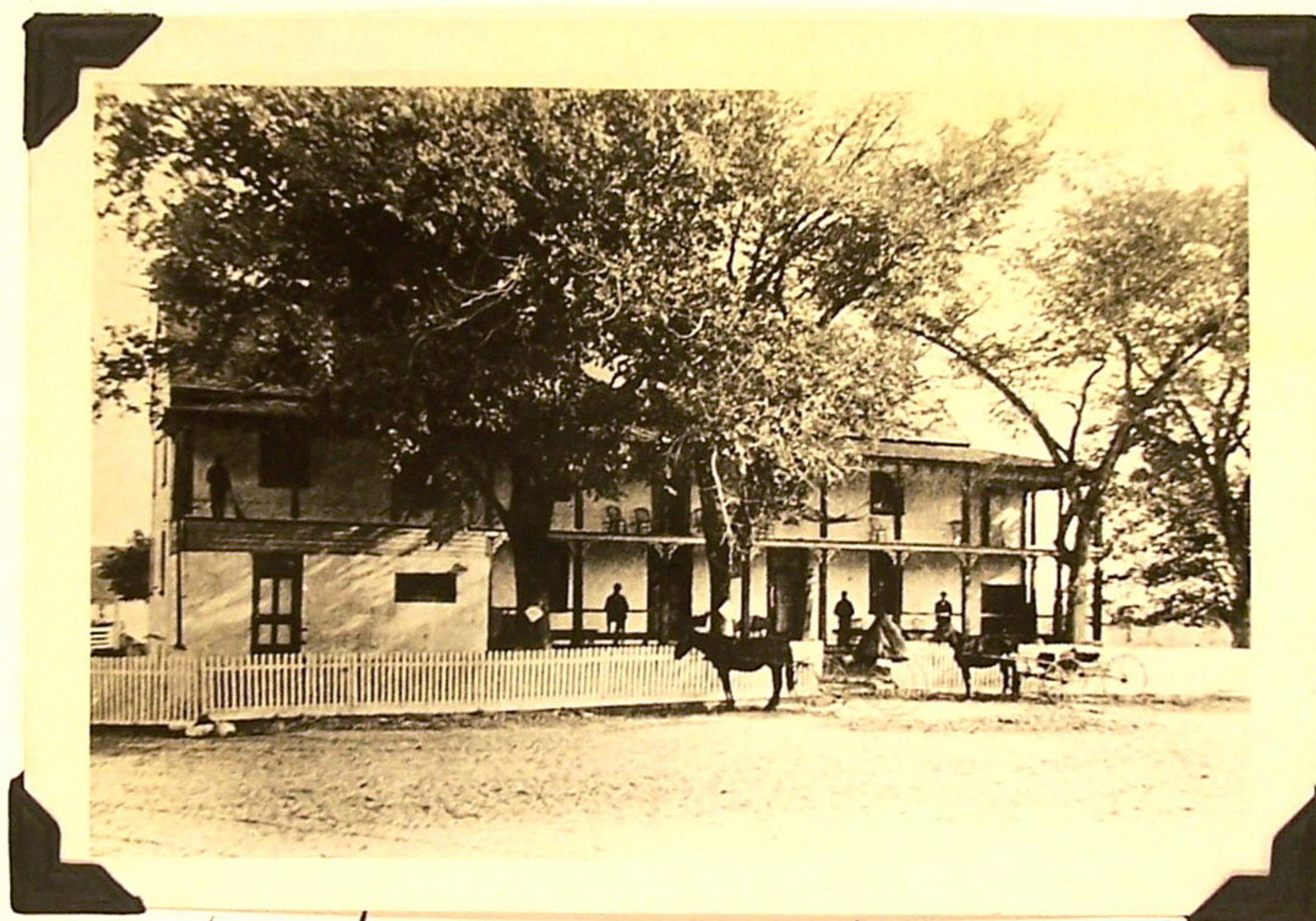
front facade - Photo c. 1900 by Robert A. Lancaster Jr.
