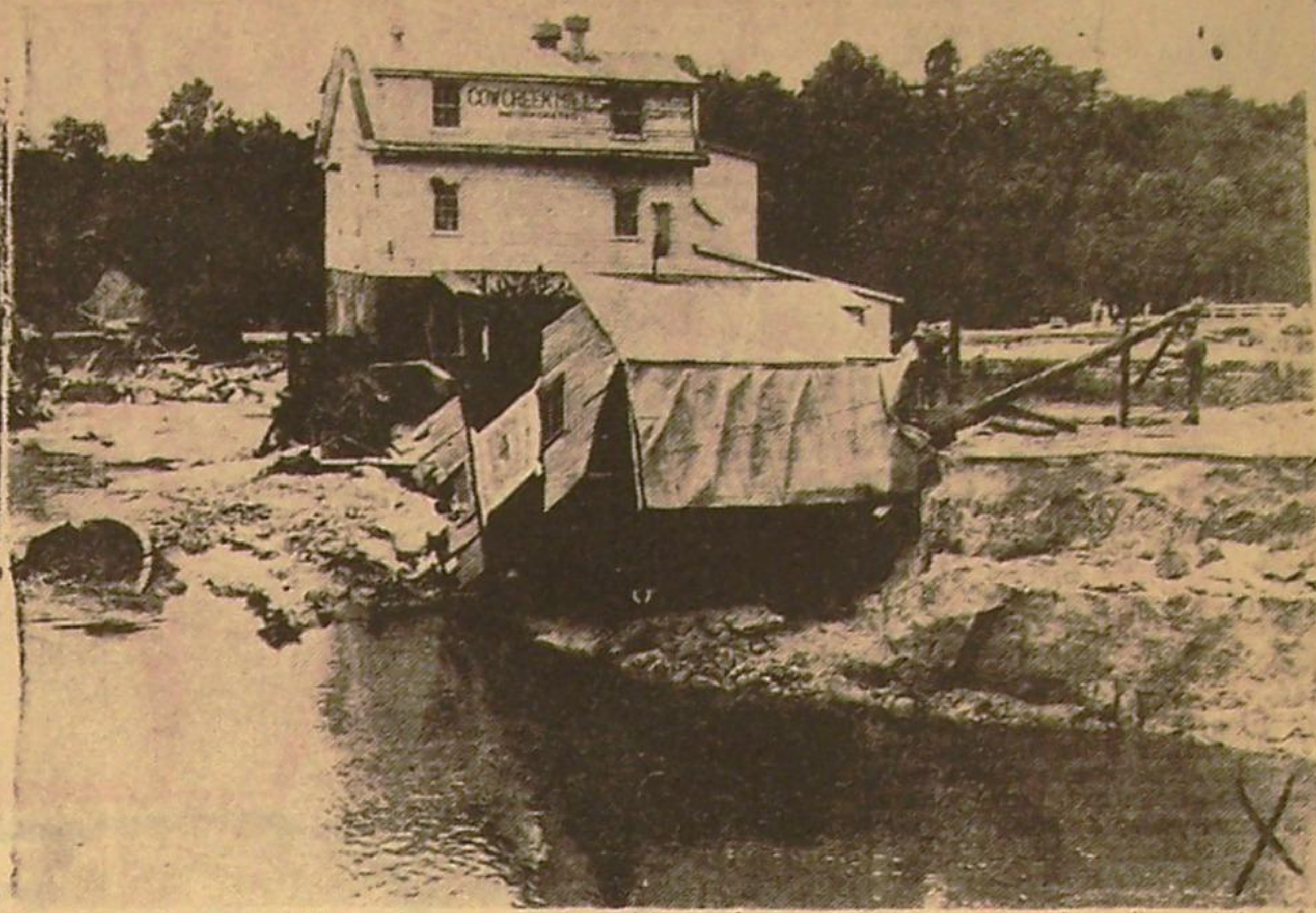
the nearby trees, and Mason jars were scattered in profusion near the scene as the mill pond, largest in the State, burst through the dam. Damages to the mill were estimated between $25,000 and $30,000. [Dementi photo.]
