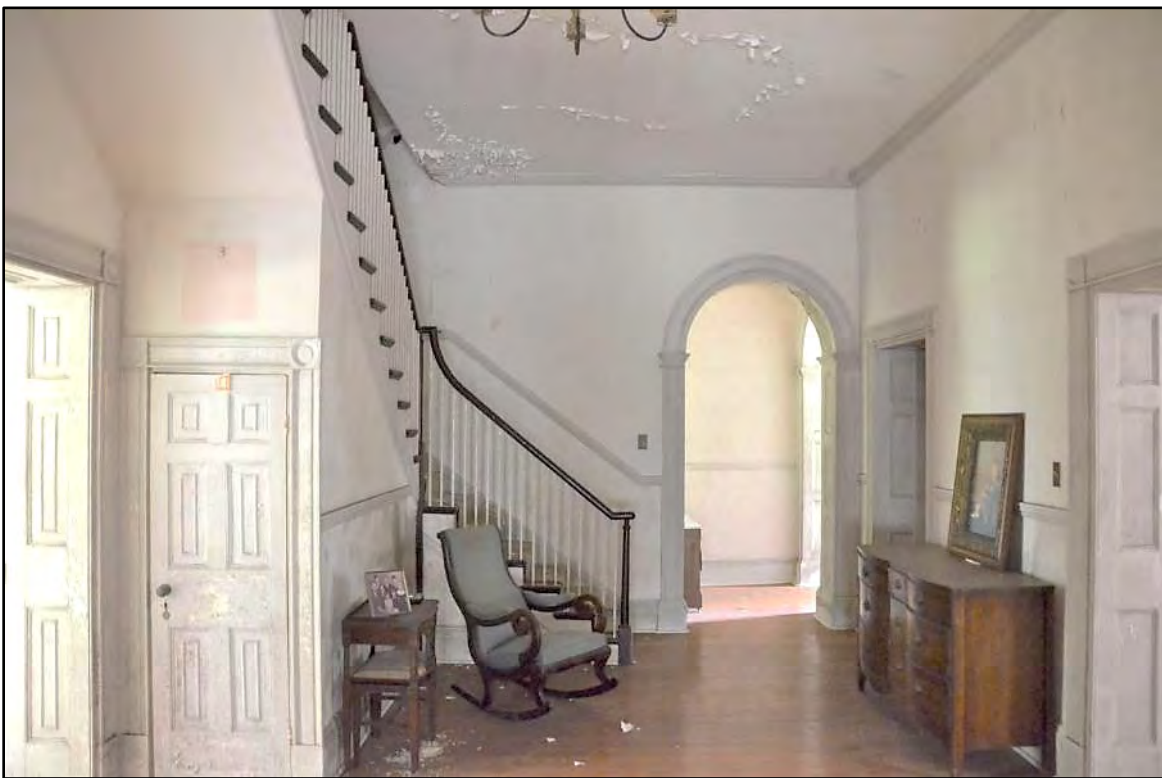
Figure 9. Looking South Through Center Hall on Second Floor. (DHR, 2018)
