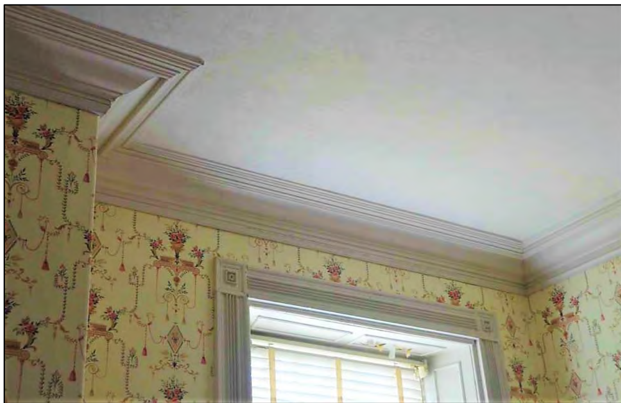
Figure 7. First Floor, East Room, Wall and Ceiling Molding (DHR, 2018)
