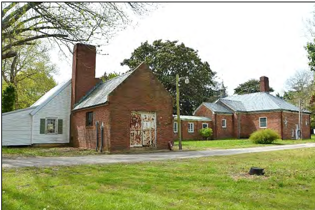
Figure 10. Looking Southwest at Row of Attached Dependencies of "Curtain" including (left to right) Ballroom, Furnace Room, Corridor, Plant Room, and Pool House.
