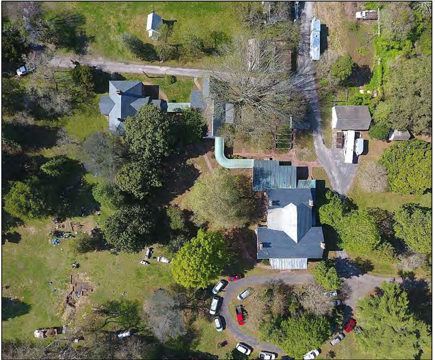
2. Eyreville, Aerial View, 2018. North is to the top of the photograph. Active archaeological investigation seen at left (west). Courtesy DHR.
