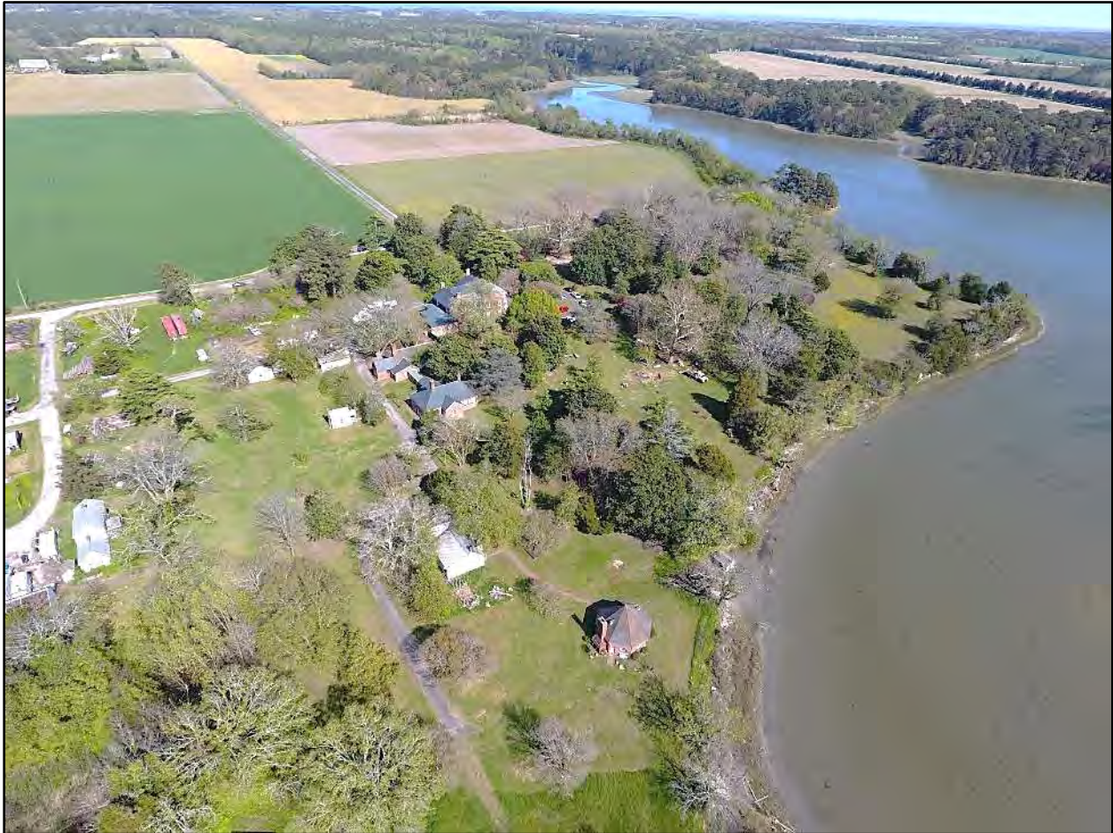
Figure 1. Aerial view of Eyreville Property Showing Main Dwelling and Associated Outbuildings within Wooded Yard, Looking Southeast. Eyre Hall lies on the south (right) side of Eyreville Creek and the long driveway (Eyreville Drive) near the center ground extends east towards U.S. Route 13. (DHR, 2019)
