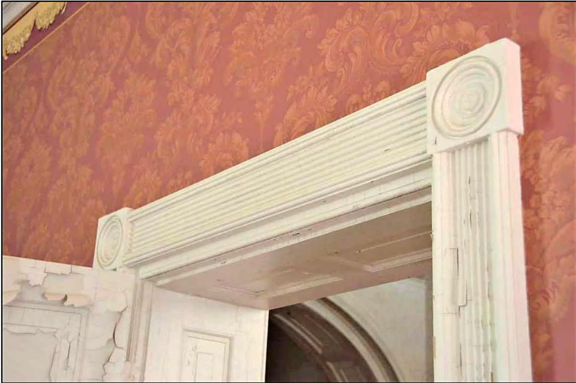
Figure 8. First Floor, West Room (library), Detail of Door Casing (DHR, 2018)
