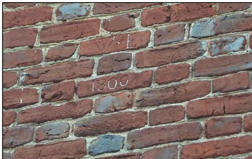
Figure 2. Detail, West Exterior Wall (Period I House) Showing Inscribed Bricks (DHR, 2018)
