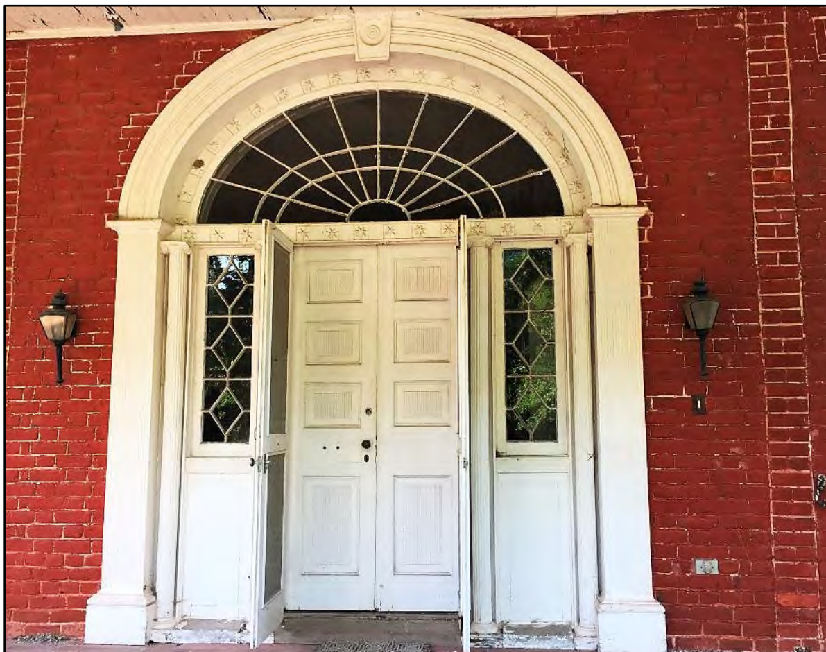
Figure 5. Detail of Entrance into Period III House Showing Elaborate Surround, Painted Brick, and Ghosting from Previous Porch Structure. (DHR, 2017)
