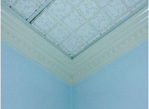
*Figure 13:* Third Floor at Intersection of Main Rectangular Section and Front Southeast Wing of Original c.1944 Section – Showing Detail of Intact Original/Historic Denticulated Crown Molding (CPG, 2022)
