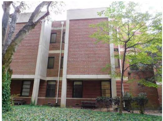
Figure 6: Northwest Elevation of Original c.1944 Front Southeast Wing – Modern Bathroom Build-Outs in Foreground, Note Historic Windows and Walls Exposed at the First-Floor Level (CPG, 2022)
