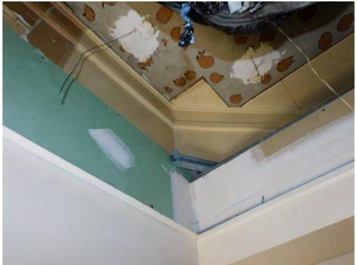
Figure 9: First Floor, Front Area of Original c.1944 Section at Intersection of Main Rectangular Section and Front Northwest Wing – Showing Intact Original/Historic Trim/Crown Molding and Metal Ceiling Tiles Above the Current Dropped Acoustical Tile Ceiling (CPG, 2022)
