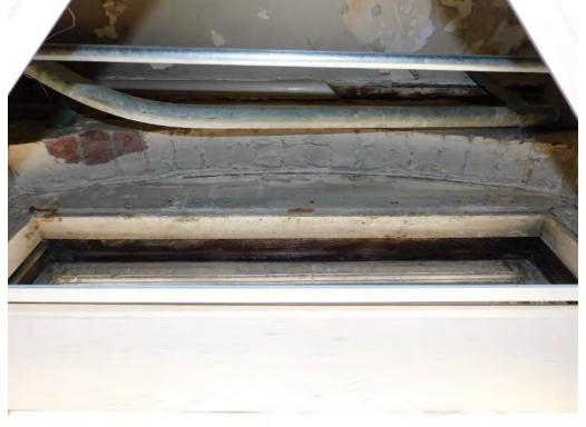
*Figure 8:* Historic Brick Arch Over First-Floor Historic Wood-sash Window, Intact Above Dropped ACT Ceiling, Original c.1944 Section (CPG, 2022)
