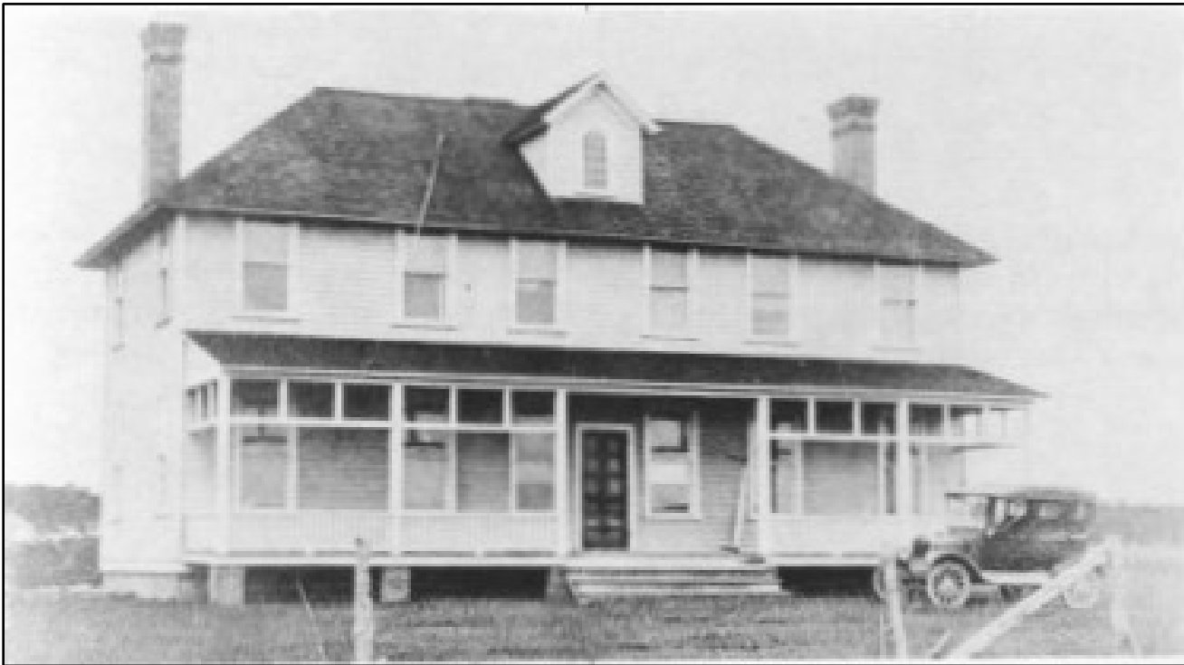
Drum Point Gunning Club (134-0219), c. 1915. Source: Johnson & Coppedge
