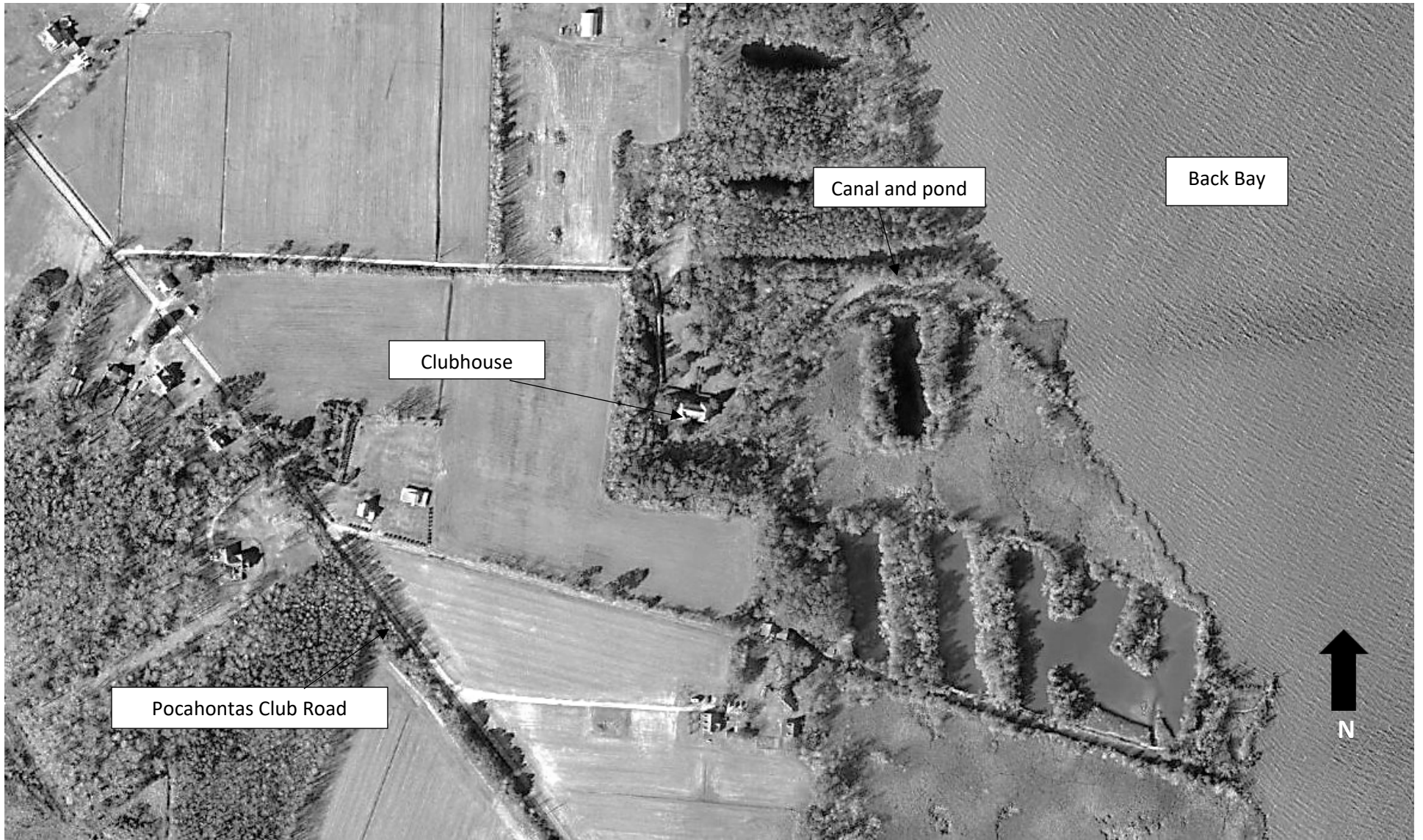
2021 Aerial Photograph of Pocahontas Fowling Club Property, City of Virginia Beach, VA 134-0171. Source: City of Virginia Beach GIS
