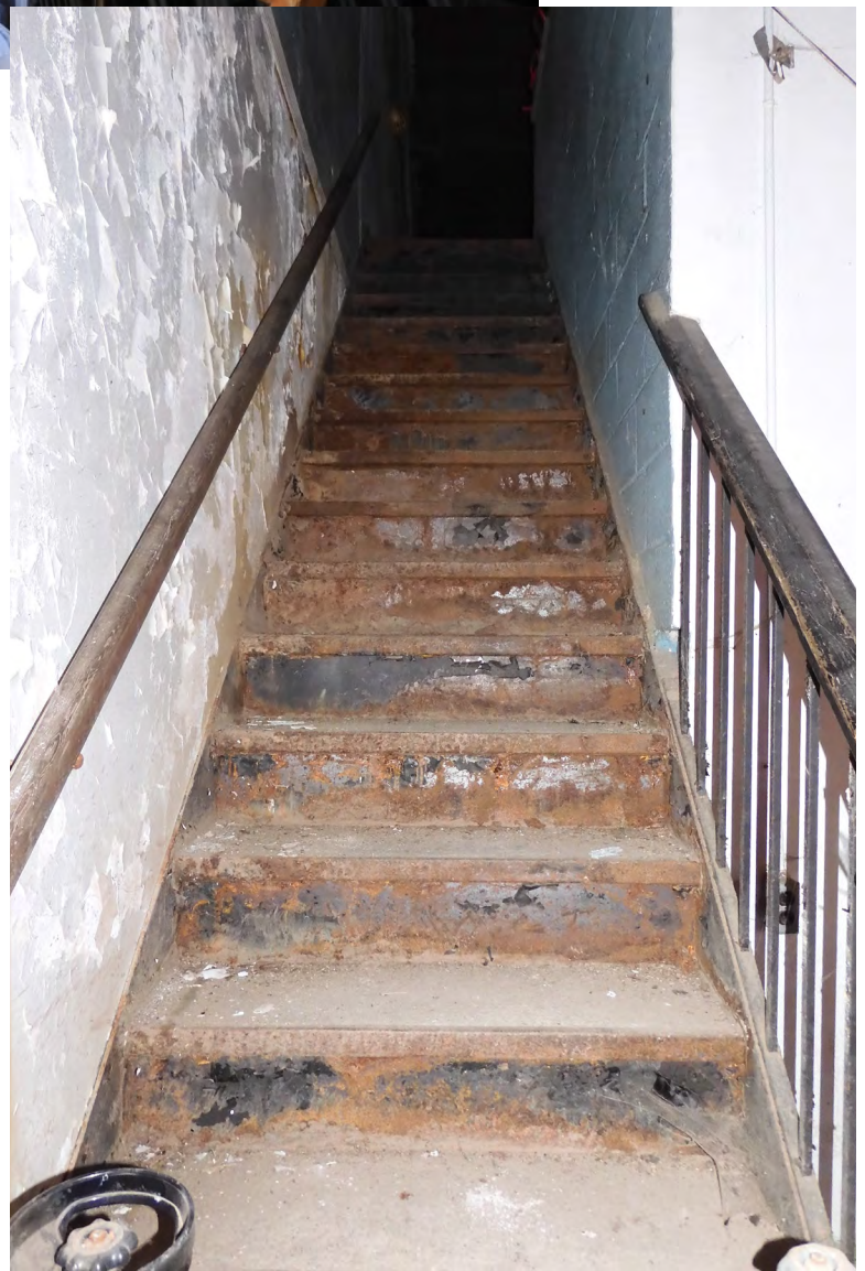
16. View of east stair to balcony.
