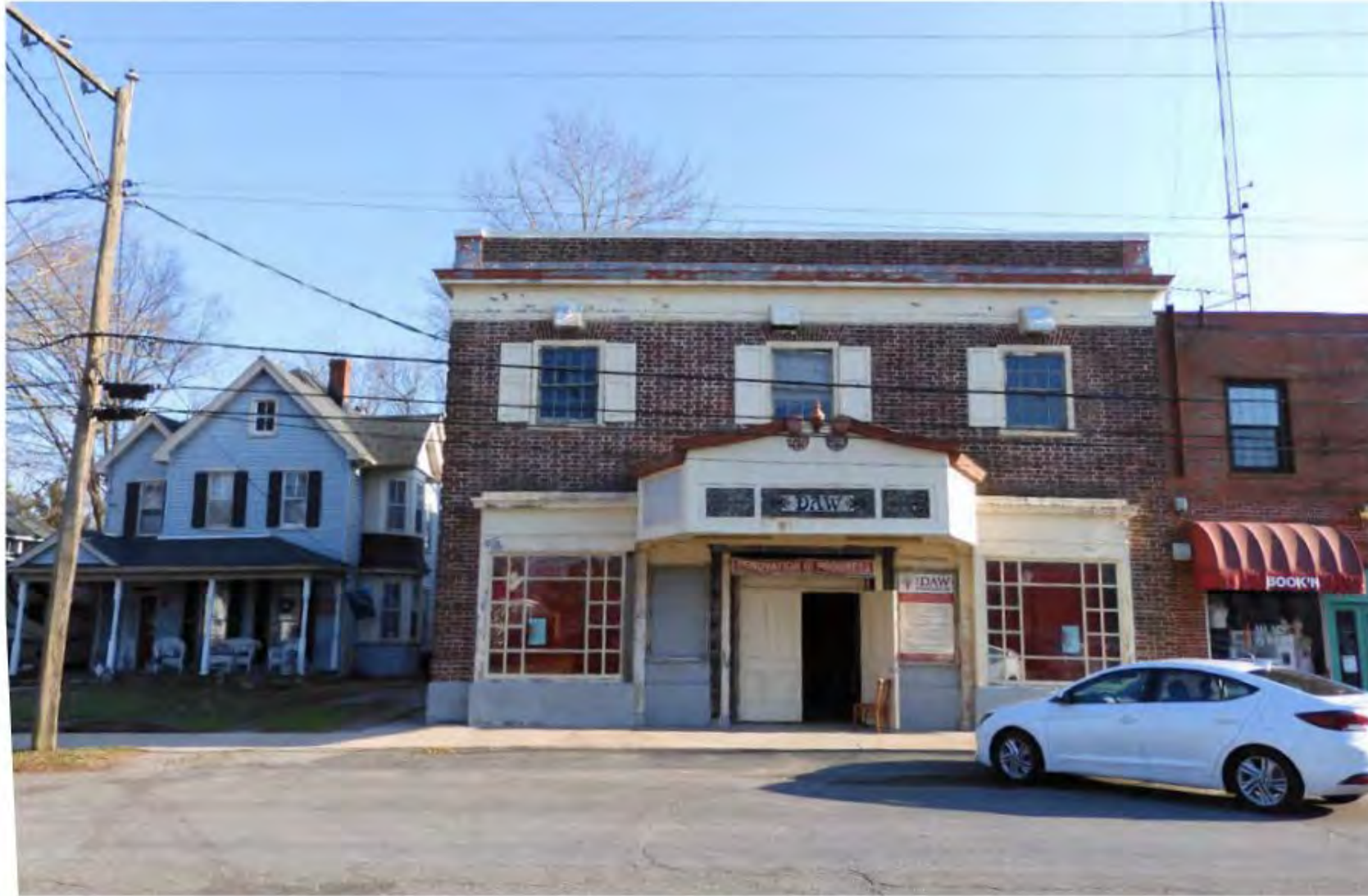
1. View of front facade of the DAW Theater.
