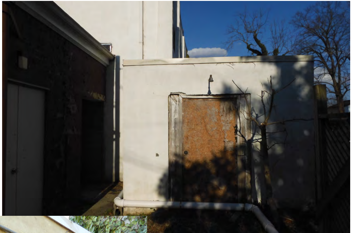
5. View of existing west entrance into rear addition.
