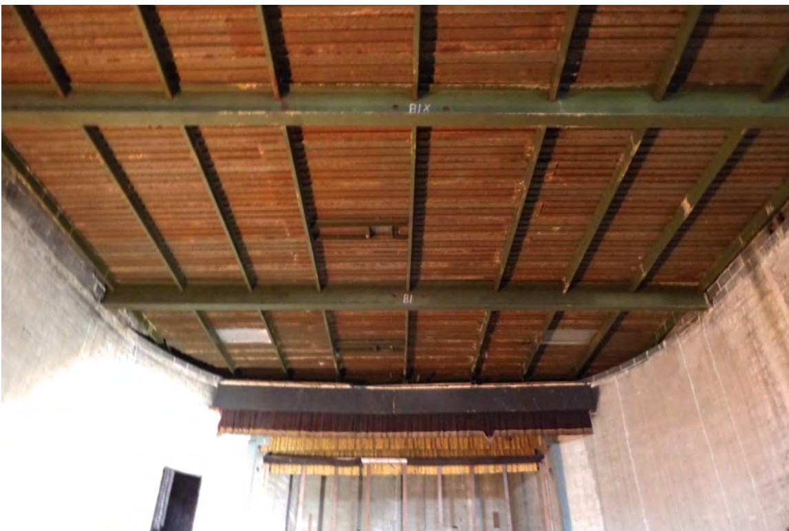
8. View of underside of roof deck.
