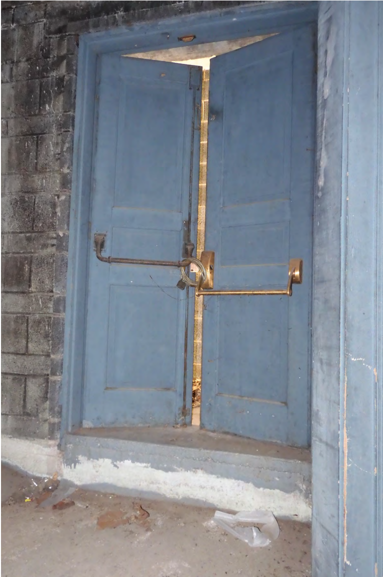
17. View of doors leading existing on west side of the building.
