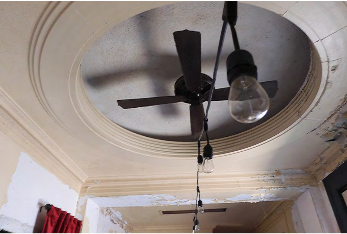
13. Detail view of ceiling medallion at the center of the lobby.
