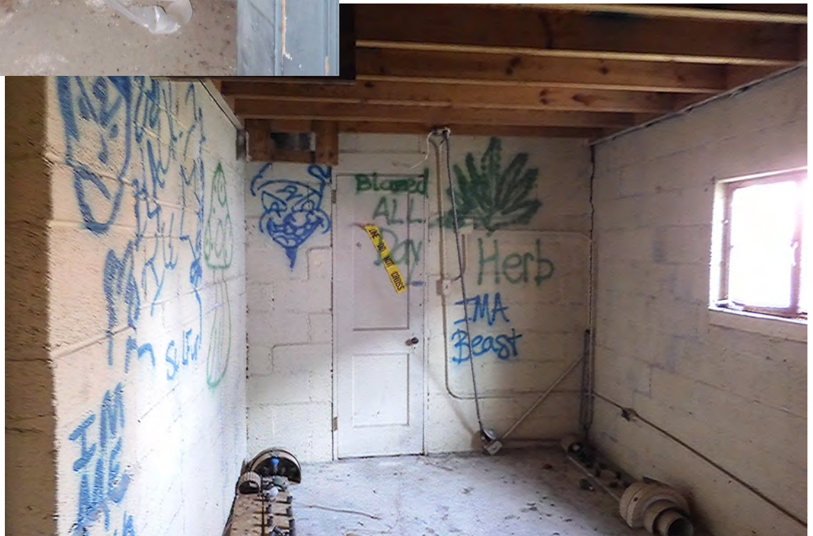
18. View of room in the rear addition.
