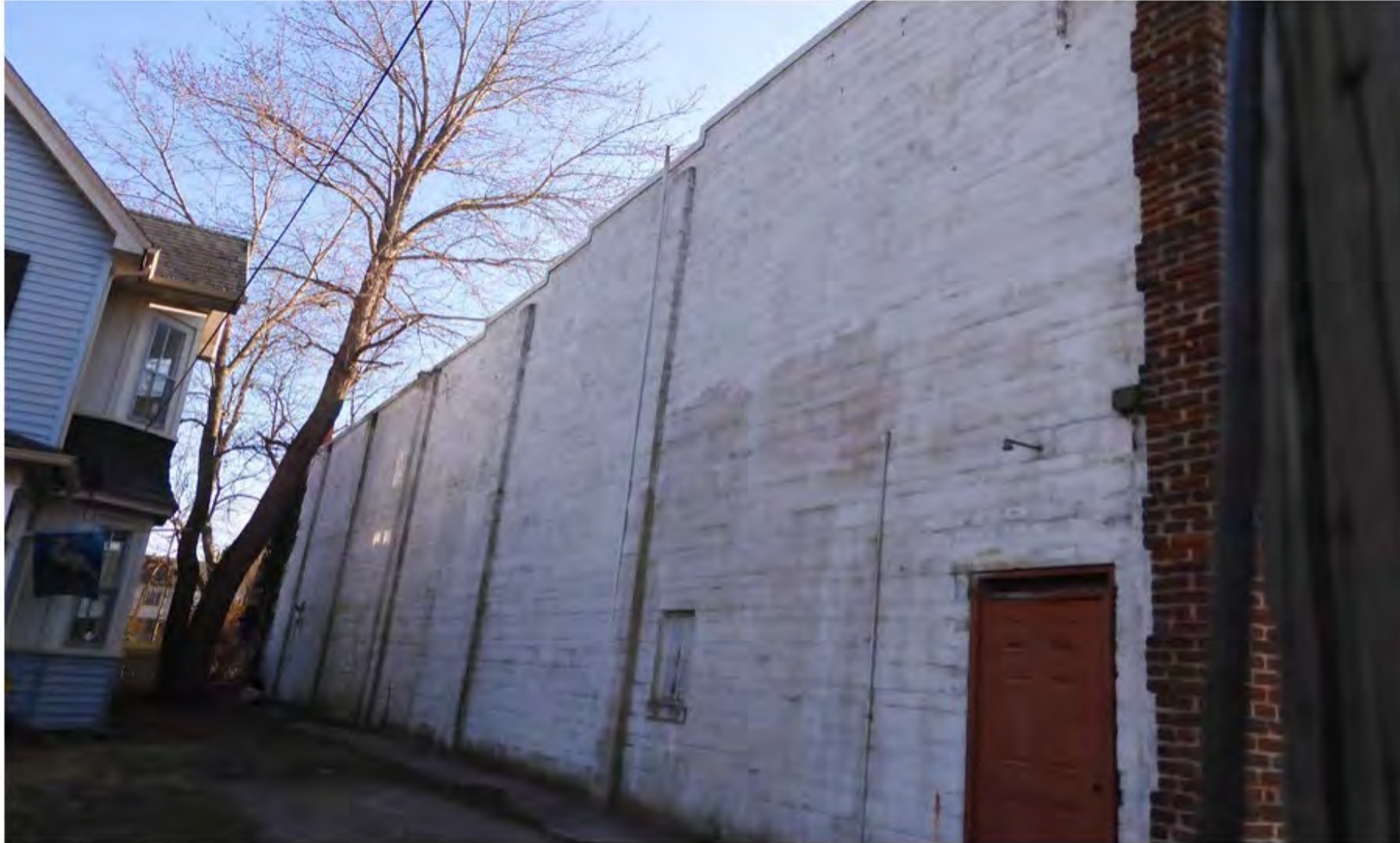
3. View of painted CMU on east side of building.
