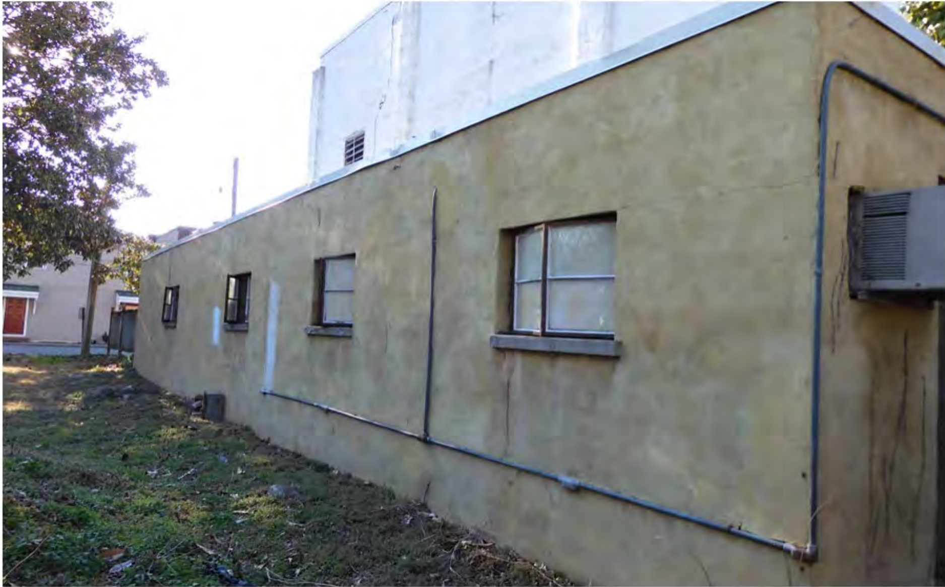
4. View of addition on rear of building.
