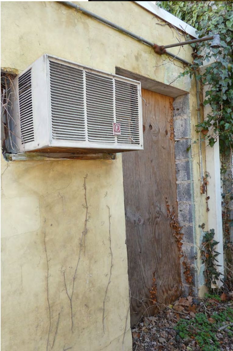
6. View of boarded up entrance on east end of rear addition.
