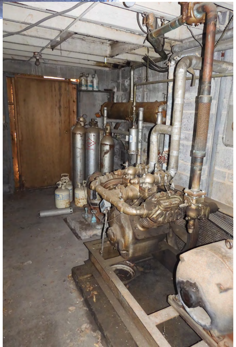
20. View of room on the west end of the rear addition.
