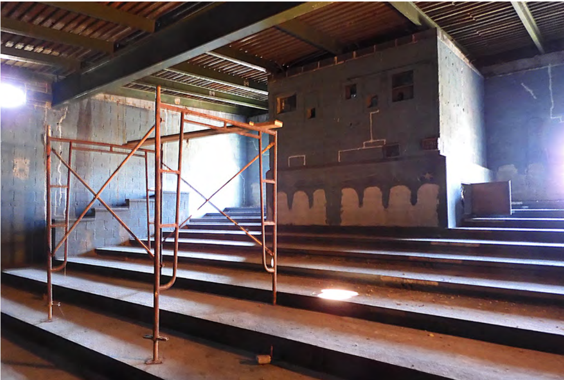
17. View of balcony space.
