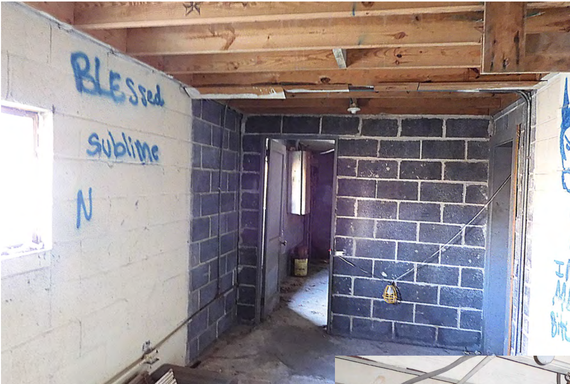
19. View of room in rear addition.
