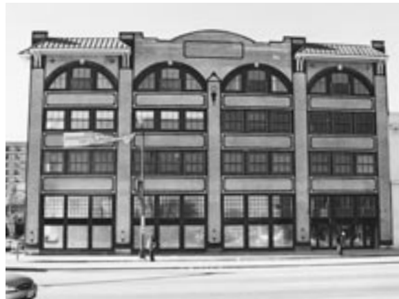
After rehabilitation as loft apartments
