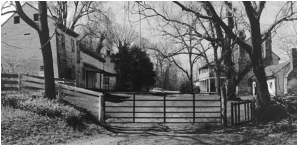
James City Historic District, Madison County
