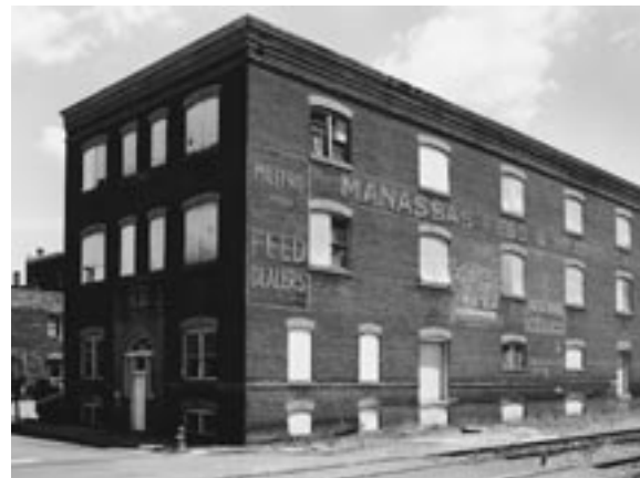
Hopkins Candy Factory Building
