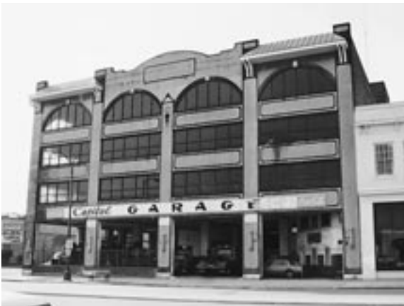
Capital Garage, Richmond, before rehabilitation
