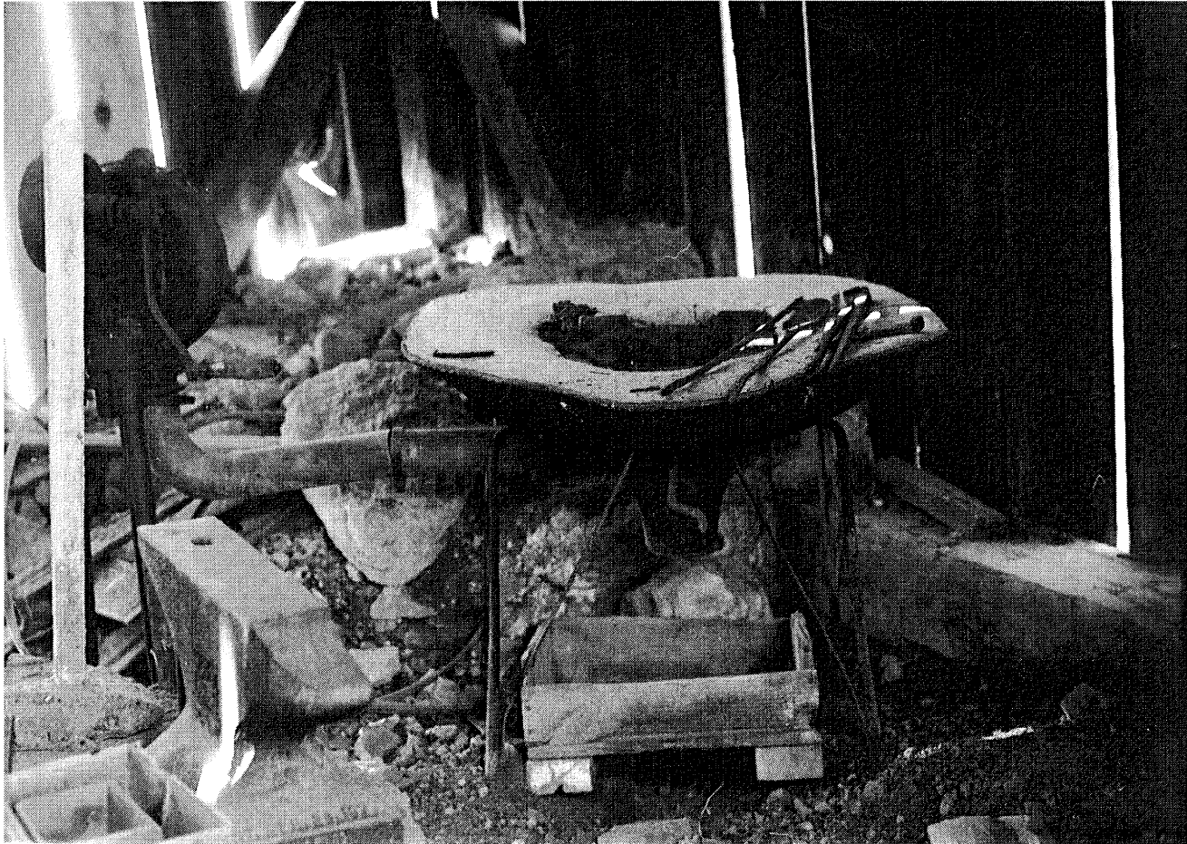
Plate 5. Portable forge, Spessard-Hylton Blacksmith Shop.
