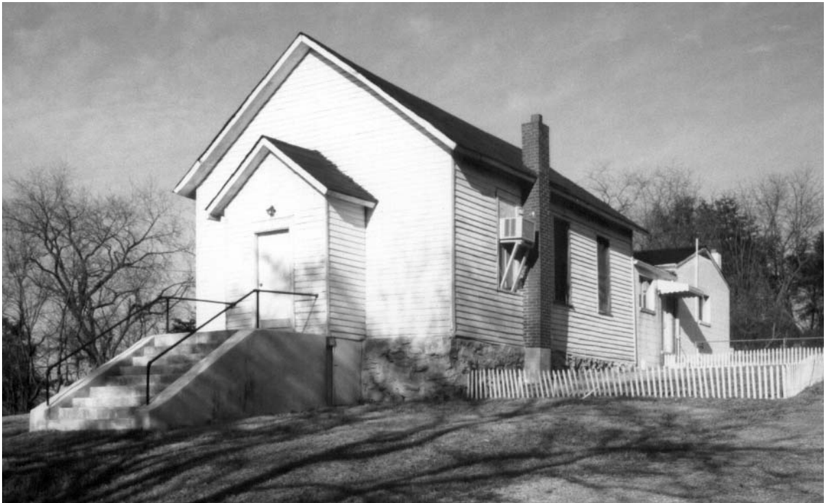
Mount Moriah Baptist Church, Roanoke: This simple country church overlooking the bustle of suburban Roanoke was built in 1908 by a congregation organized in the mid 1800s as a Sunday school for slaves.
