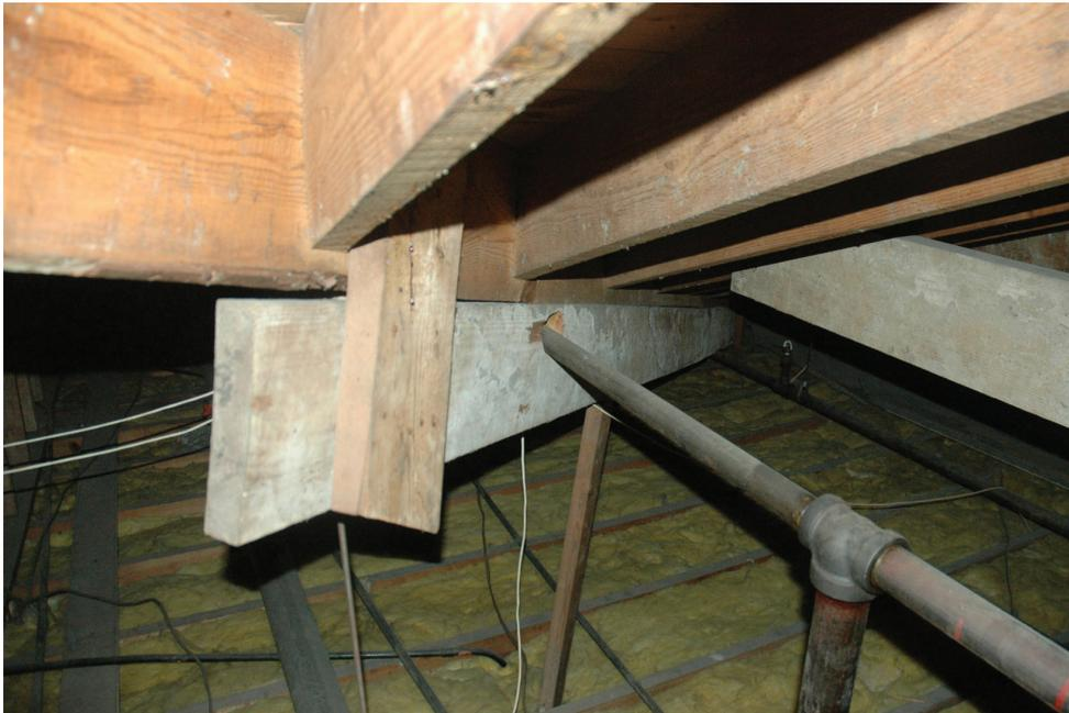
*Figure 51. Supplemental framing at valley rafters – 1939 attic.*
