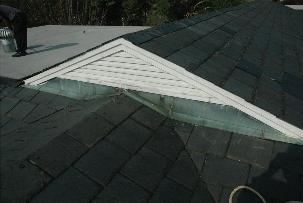
*Figure 36. Small gable – east end of 1854 roof.*
