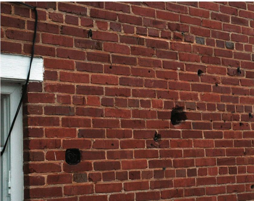
*Figure 37. Penetrations in east facade of 1939 wing.*
