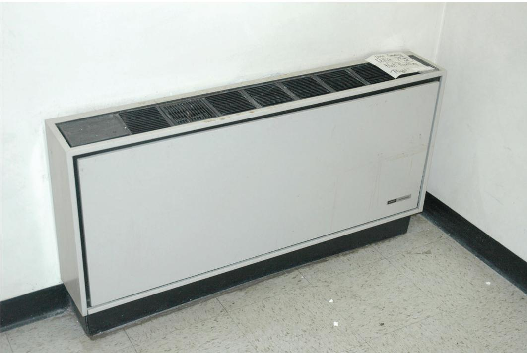
*Figure 58. Typical fan coil unit.*
