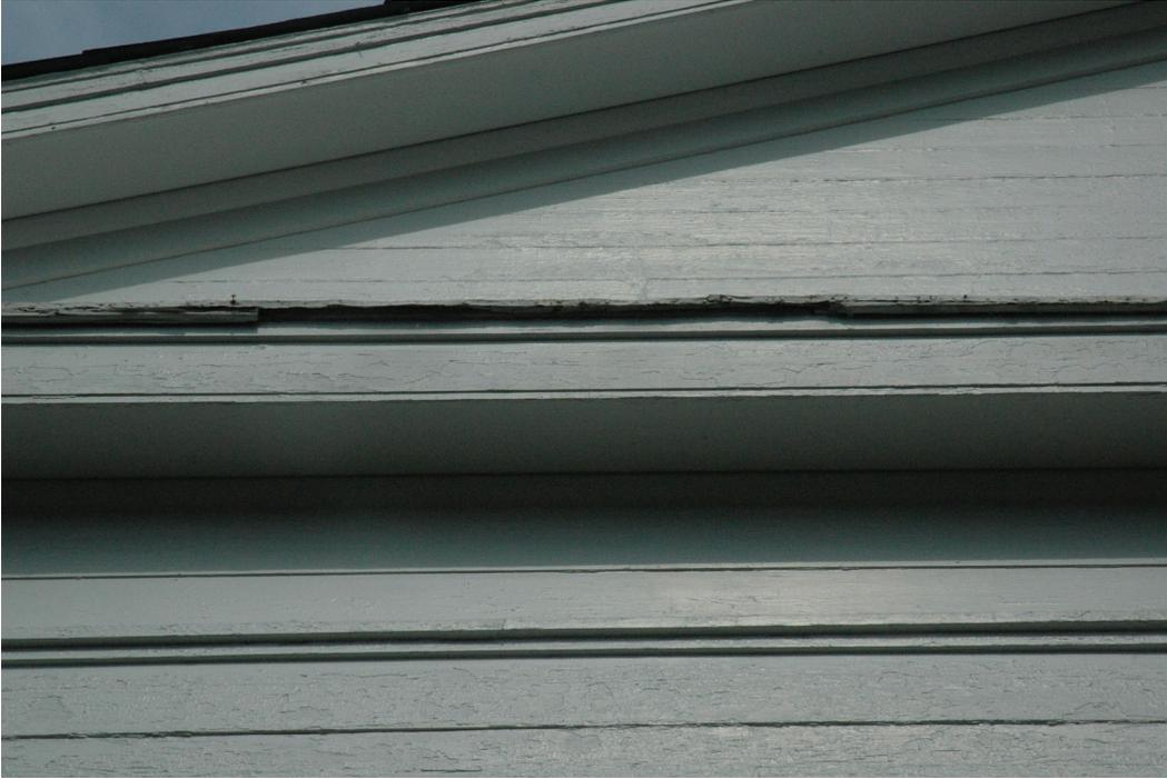
*Figure 18. Coping on horizontal cornice of portico.*
