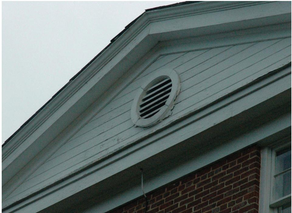
*Figure 33. North gable and louvered vent – 1939 wing.*
