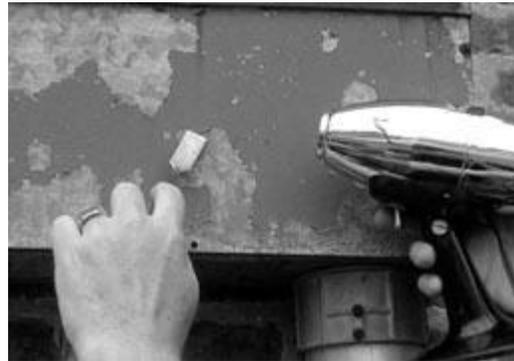
*Heat guns can soften paint on solid surfaces before it is scraped. Use extreme caution.*
