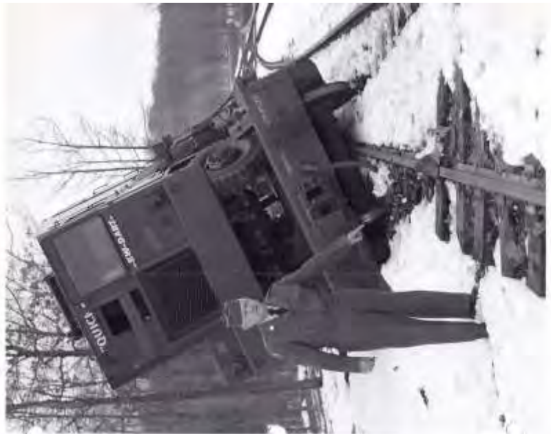
Figure 52: c. 1958 image of overturned crane north of Facility No. 2486 (Cinder Bed Road Bridge). The derail the gentleman is pointing to was used as a safety measure. Because the track is on a hill/incline, the derail was positioned so that if a cars brakes failed or tampered with, it would derail the car, versus going all the way to the main post; picture looking south; ©Daniel and Clarence Alton Seymour Collection.
