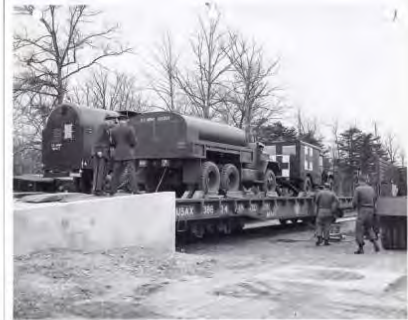
Figure 47: c. 1958; taken at Fort Belvoir, loading/unloading ramp, Facility No. 1465, while in use. The flatcar is a DoD 6-axle, heavy duty (not standard). Included in the freight (bottom right side of the cargo) is a fuel truck. ©Daniel and Clarence Alton Seymour Collection
