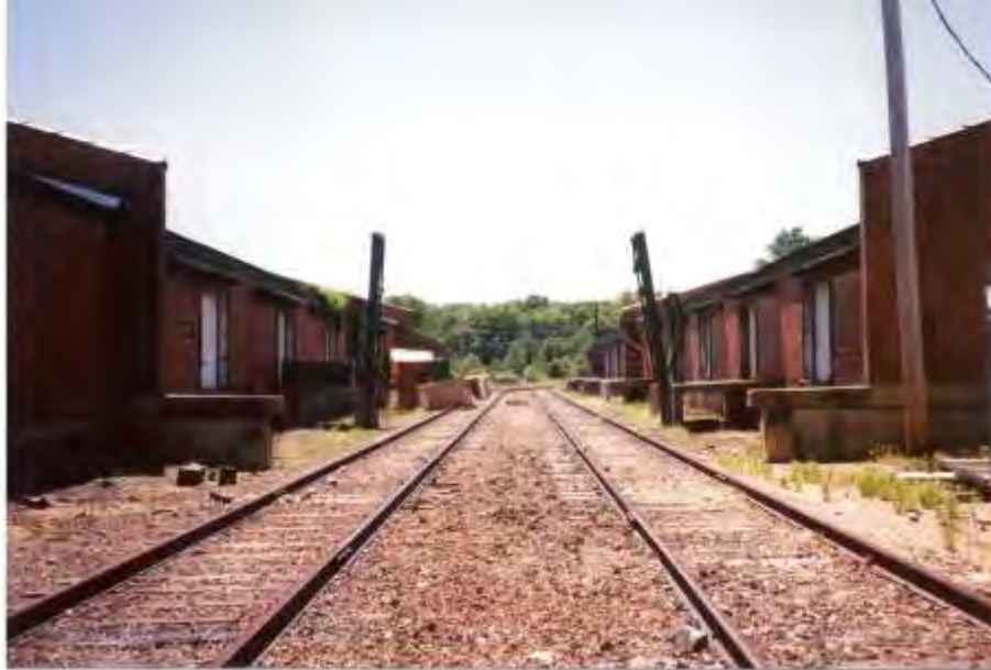
Figure 21: c. 1988; taken at Fort Belvoir of the Area 1900 warehouses and central siding, looking north. The green, metal bridges allowed personnel to walk from one row of warehouses to another (when connected). The bridges operated via electric jacks. The typical concrete platforms were used for unloading/loading boxcars. ©Daniel and Clarence Alton Seymour Collection
