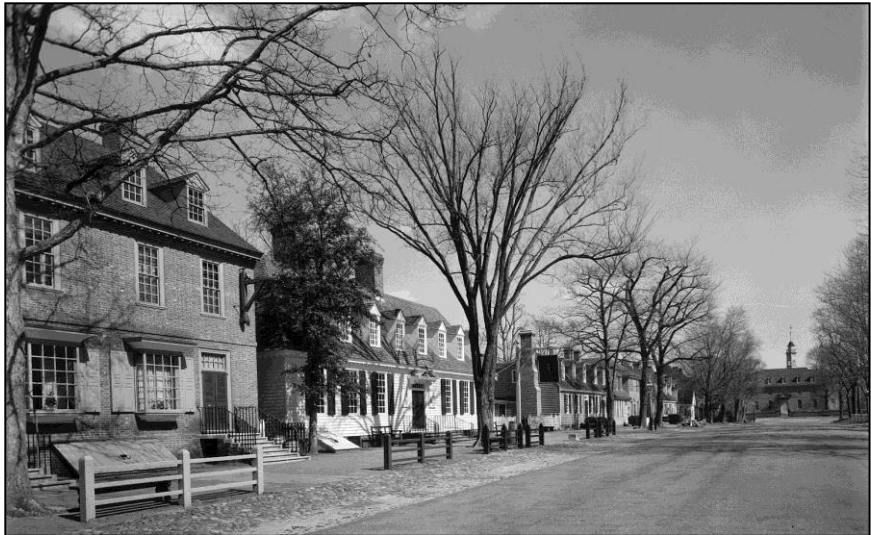
2. Colonial Williamsburg in Williamsburg, Virginia.
