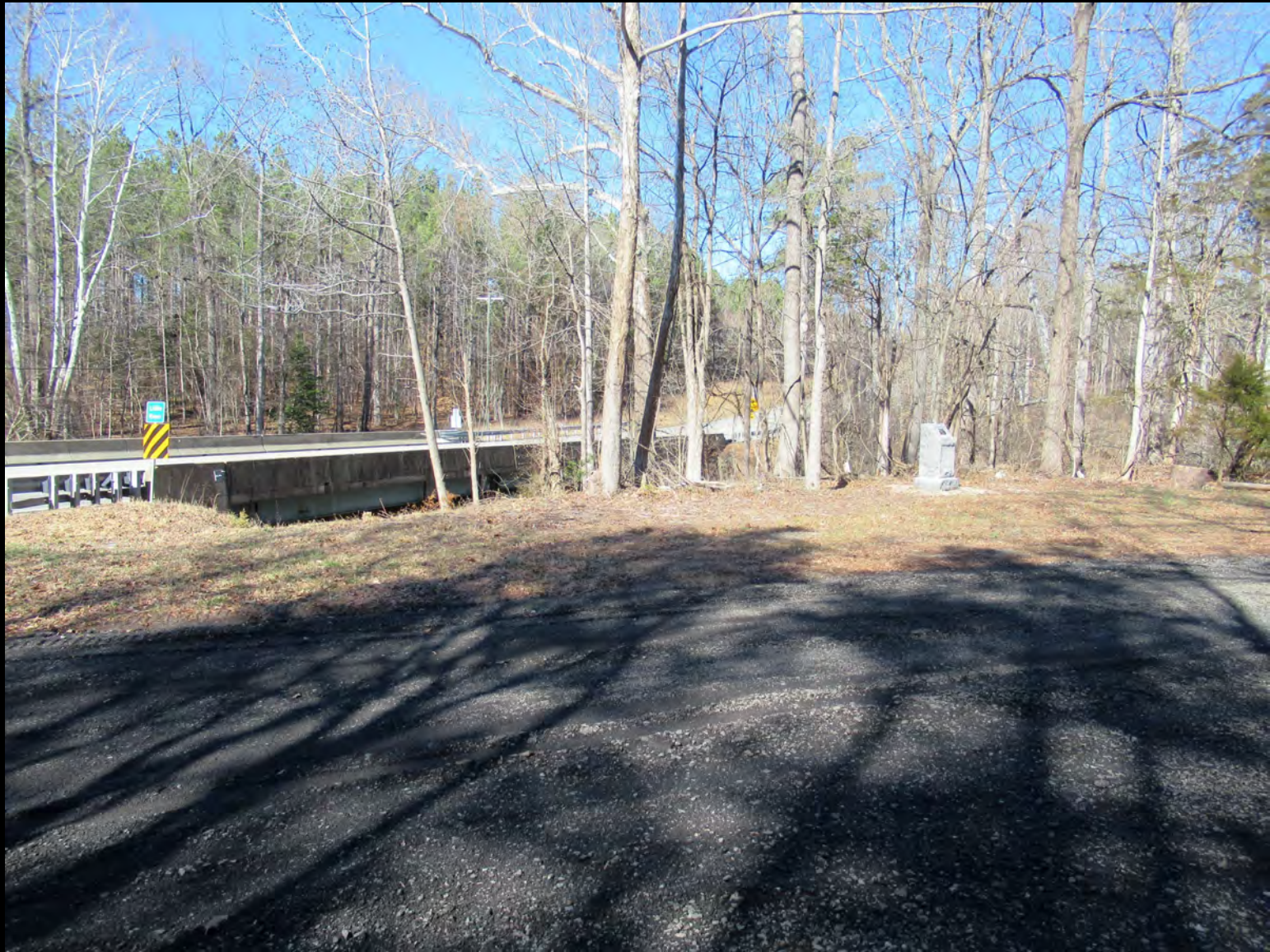
Little River relocated marker southeast of Little River Bridge, camera facing North
