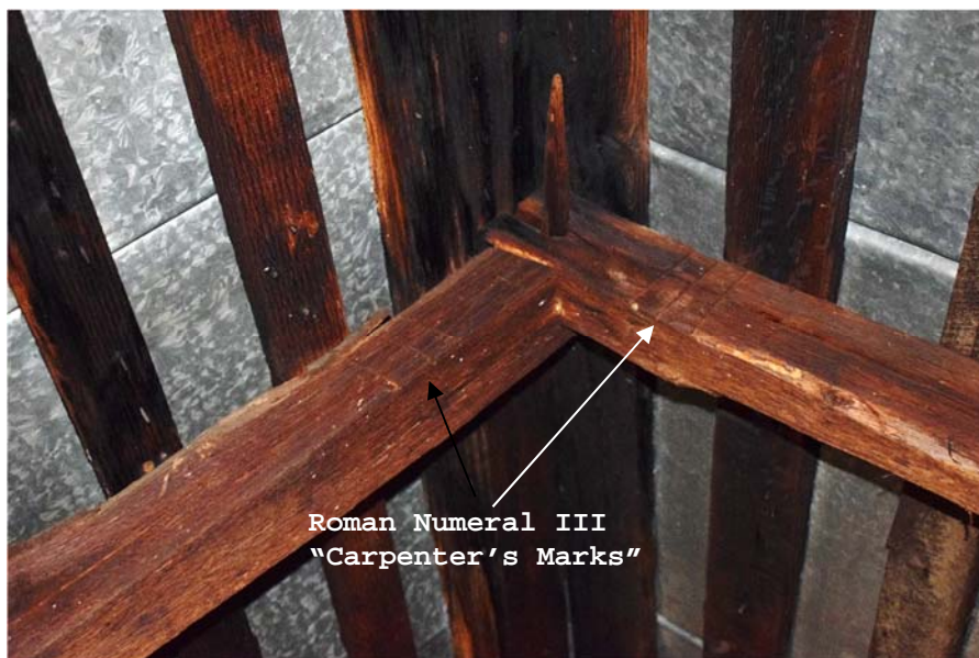
Figure 3: Attic Carpenter's Marks
