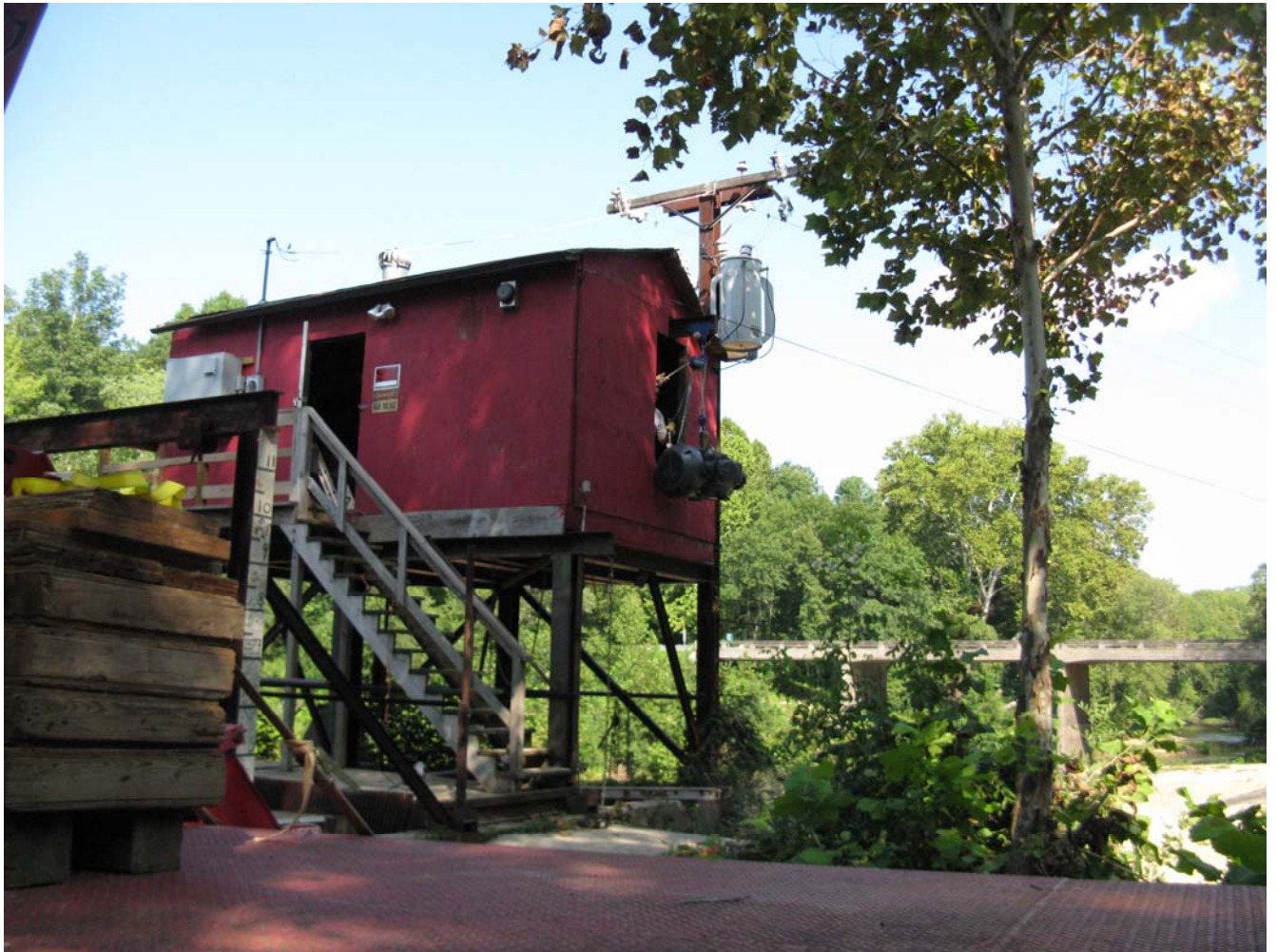
Generator being Hoisted into 1975 Powerhouse during 2010 Renovation
