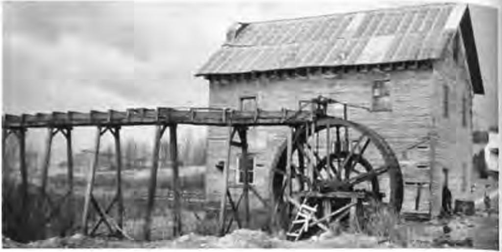
The Fitz steel wheel was installed in 1956, replacing the last wooden water wheel in use at a commercial mill in Floyd County. The race collapsed soon after this picture was taken in 1972 but the mill ran until around 1984, grinding buckwheat part-time using electric power. (Courtesy Floyd County Historical Society)
