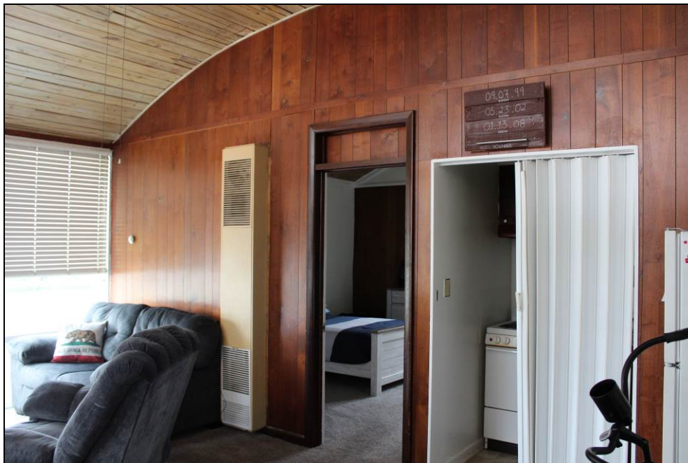
Figure 2. Current interior view of the south end, second floor unit. This unit has an original window on the south side wall that the other units lack, as shown in the historic image above.
