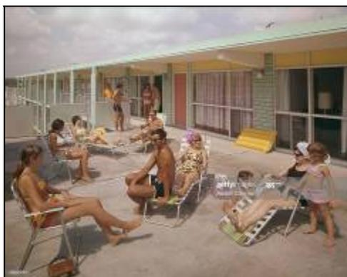
Figure 16. The Beach Carousel (above), 13<sup>th</sup> Street and Pacific Avenue, and the Mardi Gras Motel and Apartments (below), at 28<sup>th</sup> Street and Atlantic Avenue, both opened in 1968. The buildings are excellent examples of the two-story modern concrete motel covered by a flat roof with cantilevered walkways and stairs and exposed structural elements. The Mardi Gras included an on-site pool and a rooftop sun deck. Courtesy VBPL, Edgar T. Brown Collection.
