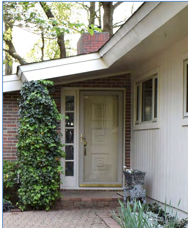
Figure 3. Detail original door (relocated) (134-5874-0080, 1305 Graham Road)
