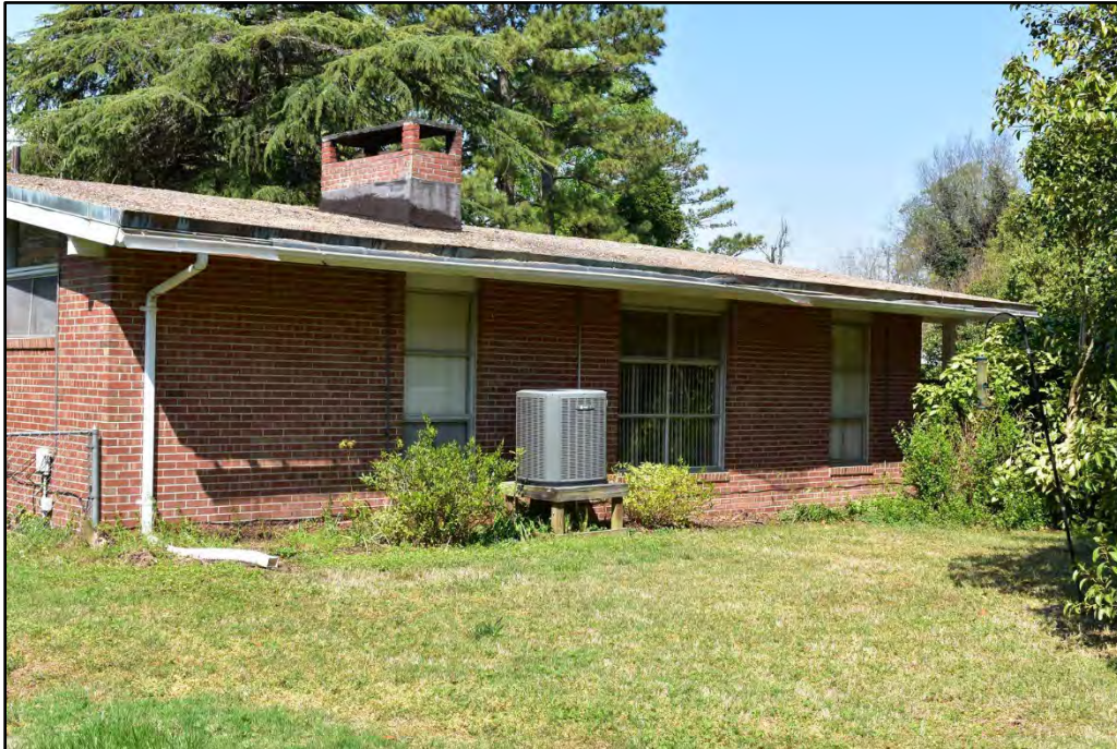
Figure 2. House retaining metal-frame windows on side elevation (134-5874-0068, 1340 Graham Road)
