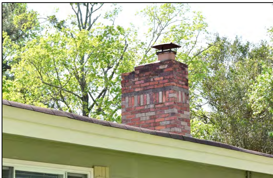
Figure 4. Chimney constructed with salvaged bricks (134-5874-0046, 1329 Woodhurst Drive)
