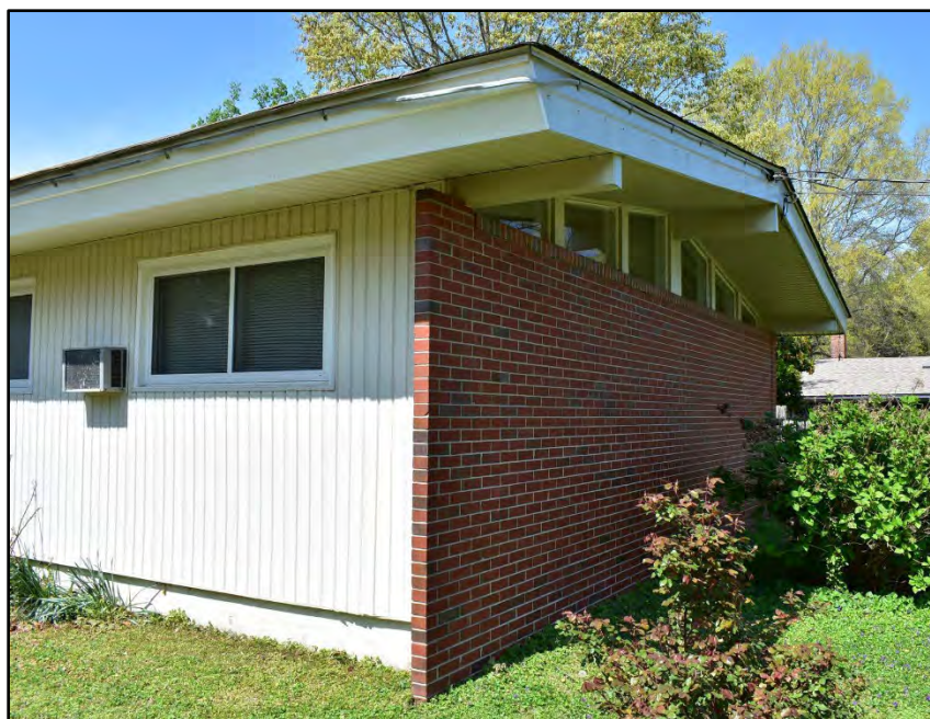
Figure 5. Detail of Model #1 brick end wall 9134-5874-0044, 1337 Woodhurst Drive)
