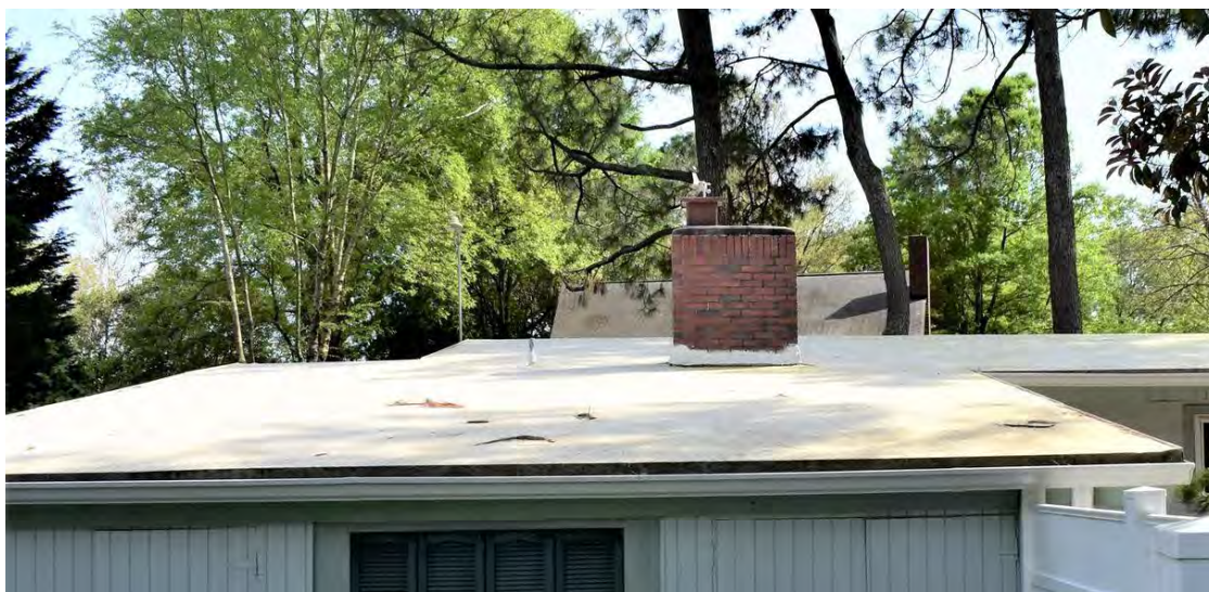
Figure 1. Roof clad with single-ply membrane (134-5874-0064, 1312 Graham Road)
