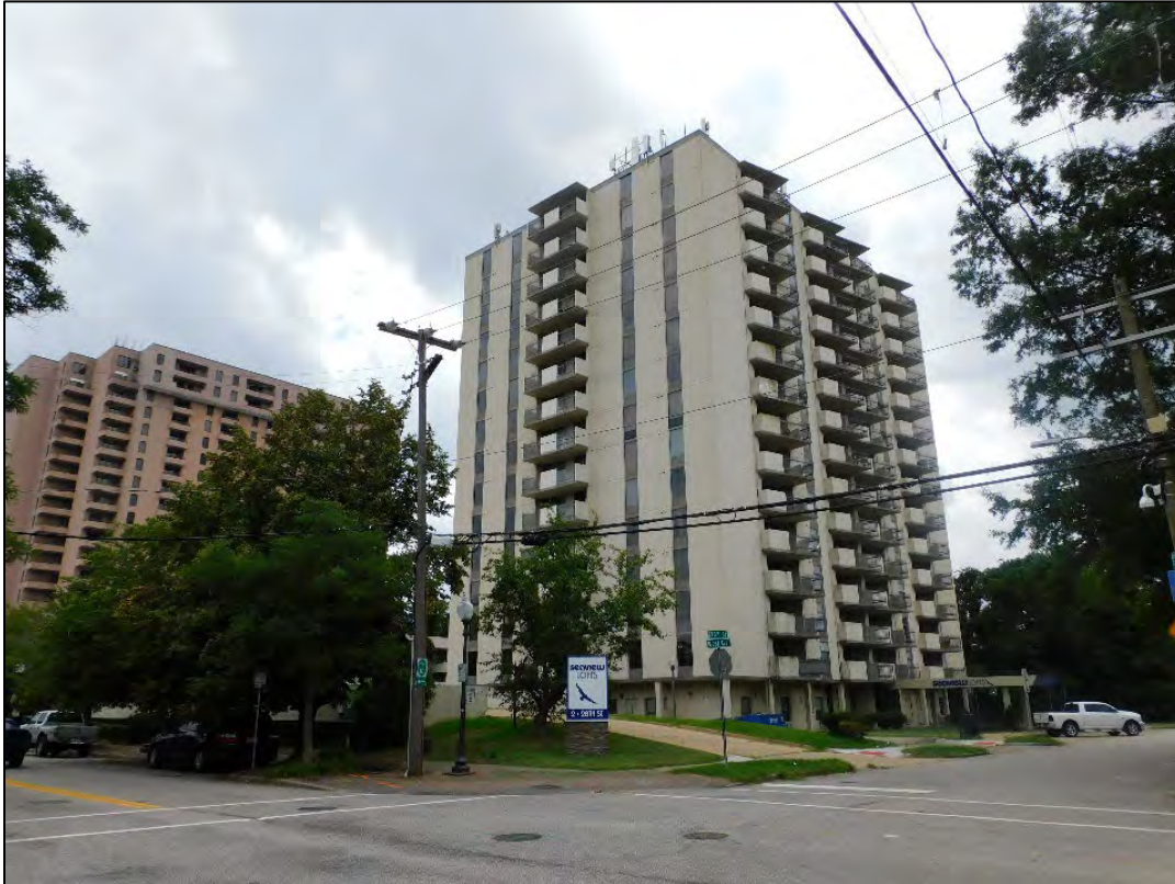
Figure 6: 90 28th Street, Seaview Lofts (DHR# 121-5621-0029)
