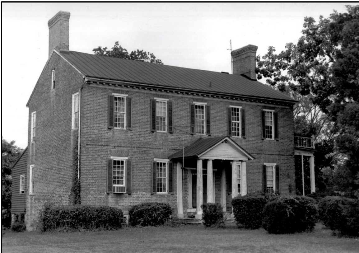
Figure 1: Pleasant Hall, 1972 Survey photo showing the Greek Revival porch, the rear lean-to addition, and the side porch, as well as other modern alterations such as the shutters and the roofing material. (Image courtesy of VDHR Archives, Resource ID #134-0027)
