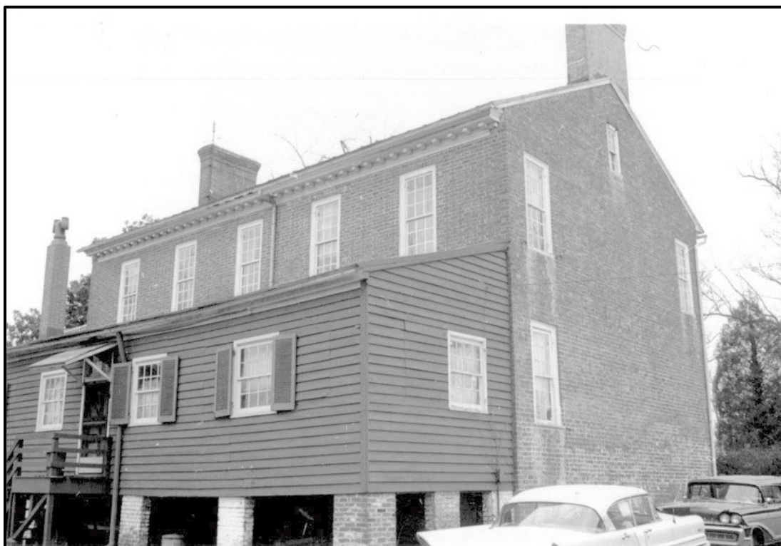
Figure 2: Rear, c.1890 lean-to addition to Pleasant Hall, c.1968 (Image courtesy of VDHR Archives, Resource ID #134-0027)
