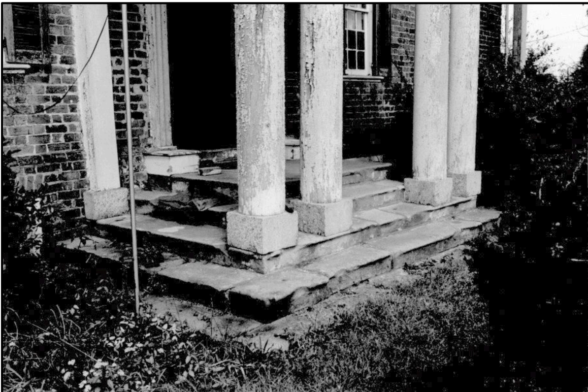
Figure 4: 1972 photo showing the granite blocks used as the column bases on the Greek Revival Porch, 1972 Survey and NRN (Image courtesy of VDHR Archives, Resource ID #134-0027)
