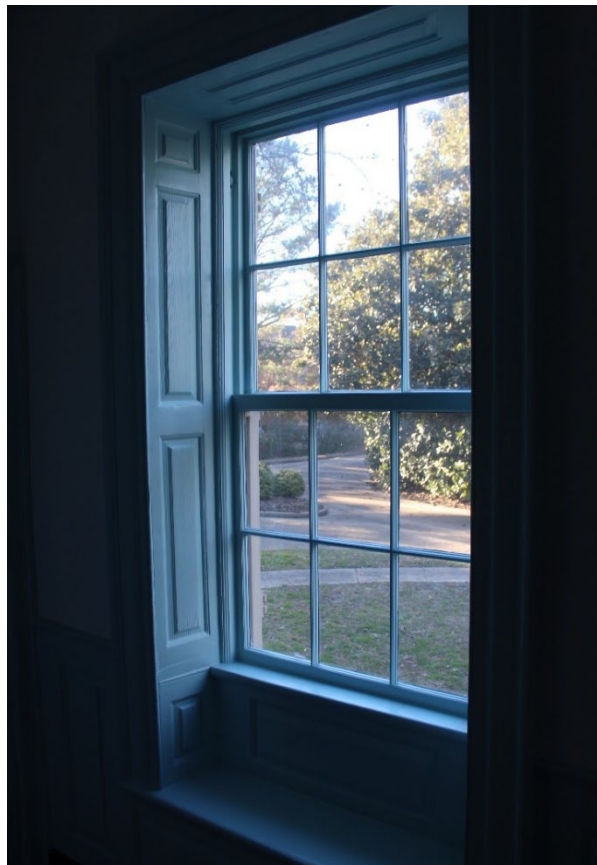
Figure 13: Detail of window shutter paneling in dining room
