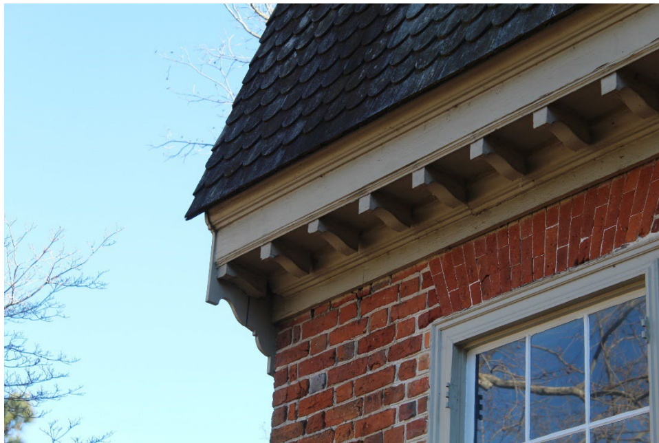
Figure 5: Detail of roof cornice on facade
