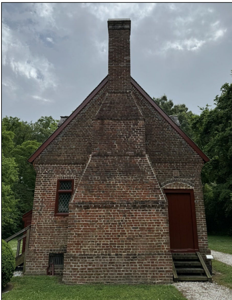
North side elevation, May 2024. Original window opening on the first story and original cellar window opening to the left of the chimney. Original doorway to the right of the chimney. Note glazed headers following the rake of the roof.
