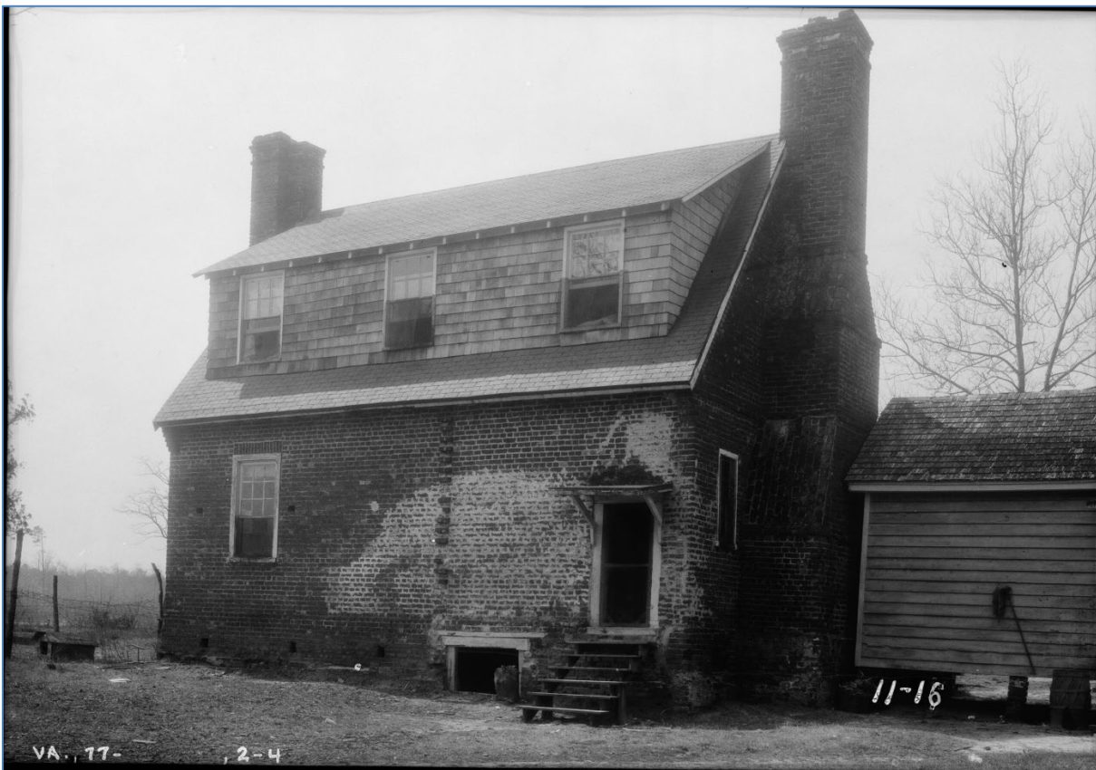
Rear elevation of Lynnhaven House, ca. 1936, showing the same brick racking illustrated by the photo above, along with surviving plaster on the rear wall. Image courtesy of HABS/Library of Congress.
