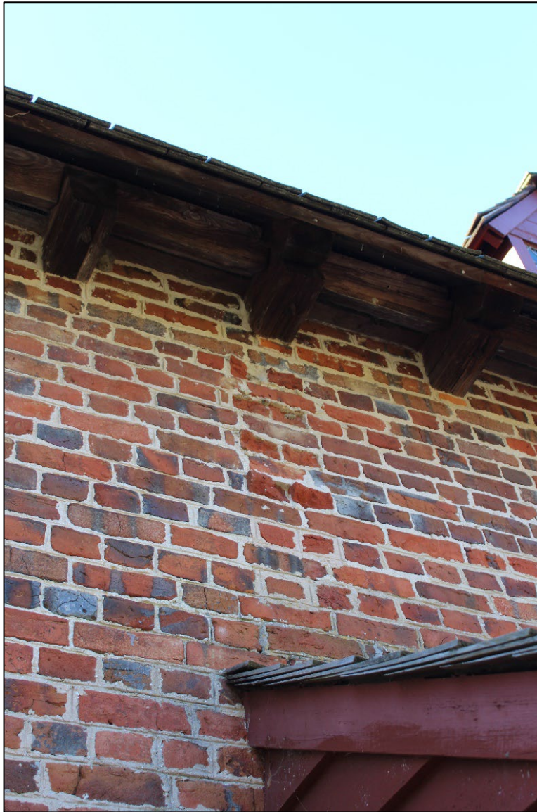
Evidence of missing rear wing. Note broken bricks in the middle of the photo. December 2023.
