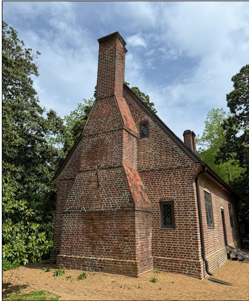
Thoroughgood House, Virginia Beach, Virginia, May 2024. Compare the chimney, the brick corbels at the corners, and the glazed headers following the rake with Lynnhaven.
