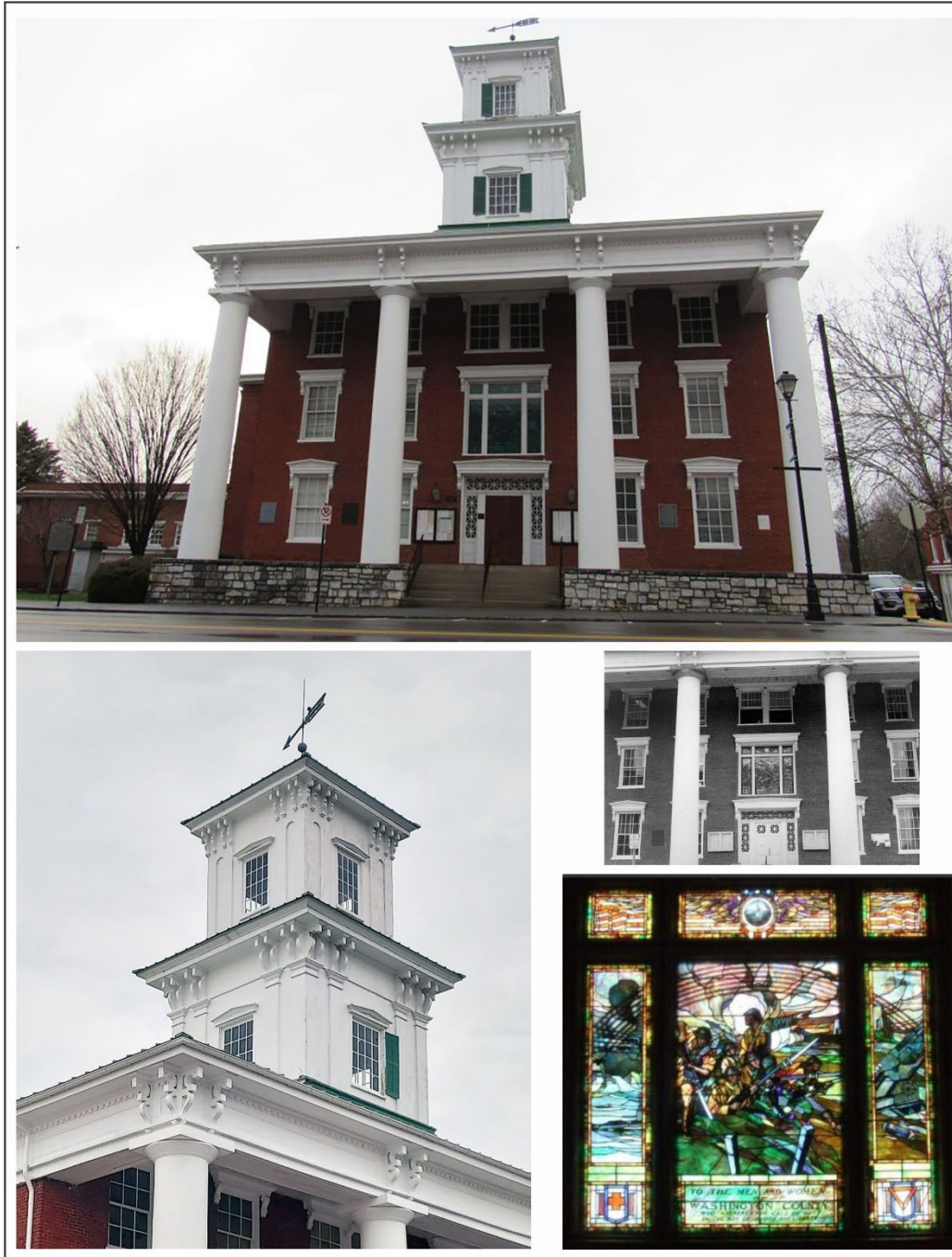
Figure 3. Washington County Courthouse (140-0037-0064; 189-191 East Main Street) (clockwise from top: Façade [V-CRIS 2020]; Detail of façade showing location of 1919 stained glass memorial window by Louis Comfort Tiffany above main entrance [V-CRIS 1978]; memorial window [Garrett Jackson 2025]; Detail of cornice and cupola [David Lewes 2025]).
