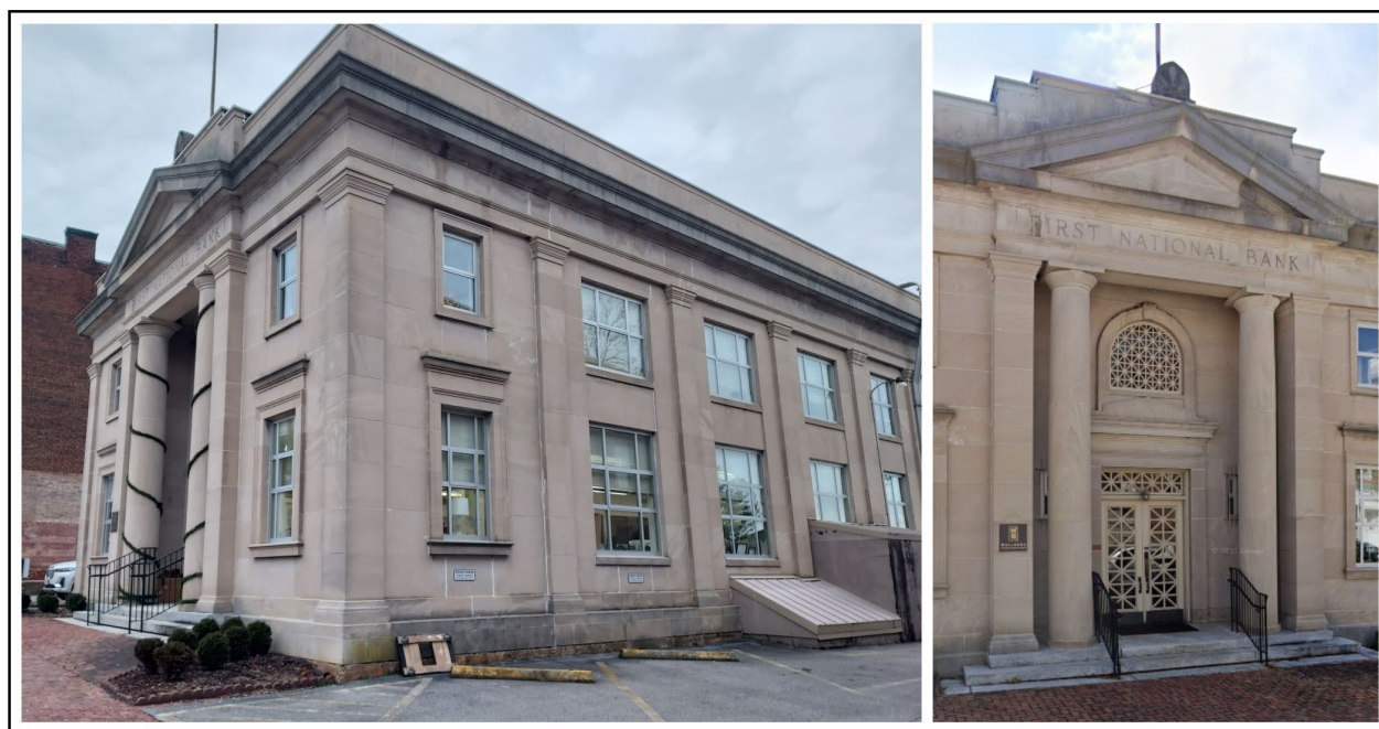
Figure 5. First National Bank (140-0037-0022, 174 East Main Street), west corner and entrance detail (David Lewes 2025; GoogleEarth).
