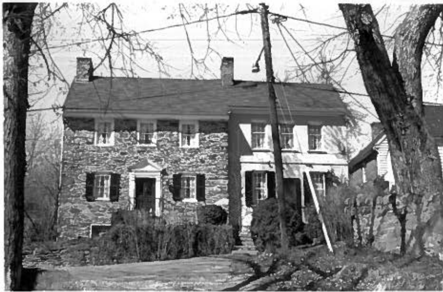
401-74 "The Moore-Means House" 3552 Two Storey, Six Bay Rubble Stone and Brick dwelling. Original stone house to the left of the existing one is now gone. Existing stone house built circa 1760 by Mahlon Janney. Brick addition built in the early 1800's by Asa Moore.
