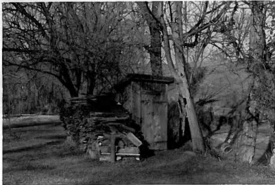
401-85 2606 Frame Outhouse on the "Mahlon Myers House" property.
