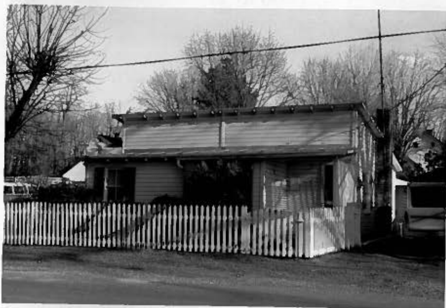
401-44 2606 One Storey, Shed Roofed, Commercial building of frame construction. Now used as a residence. Built circa 1920 as a Store.
