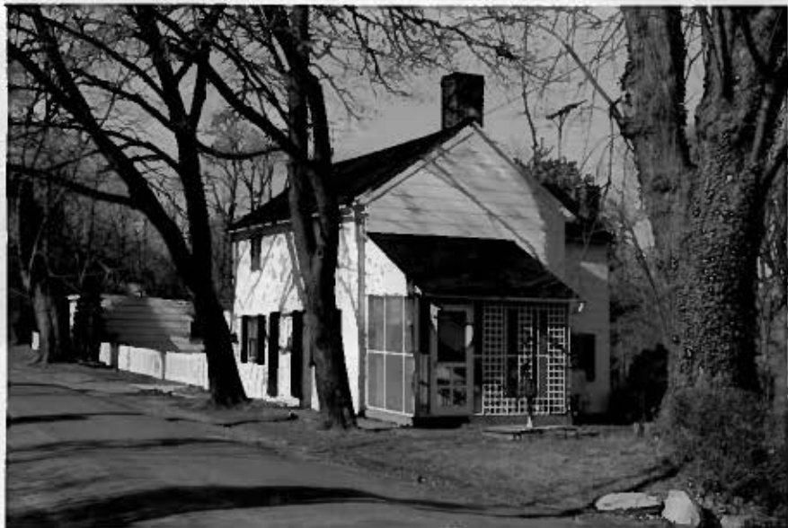
401-86 2606 Two and Three Bay Frame, Two Storey small house with Two Storey Frame rear wing. Garage shown in the background is built on the site of the Slaughter House for which Butchers Row (Street) was named. House built in the last quarter of the 1800's.
