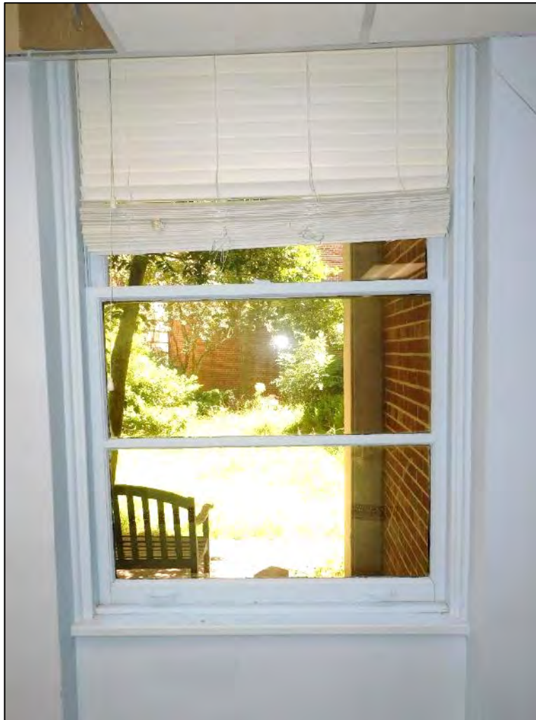
Figure 7: Historic First-Floor Wood-Sash Window, 1944 Building (CPG, 2022)
