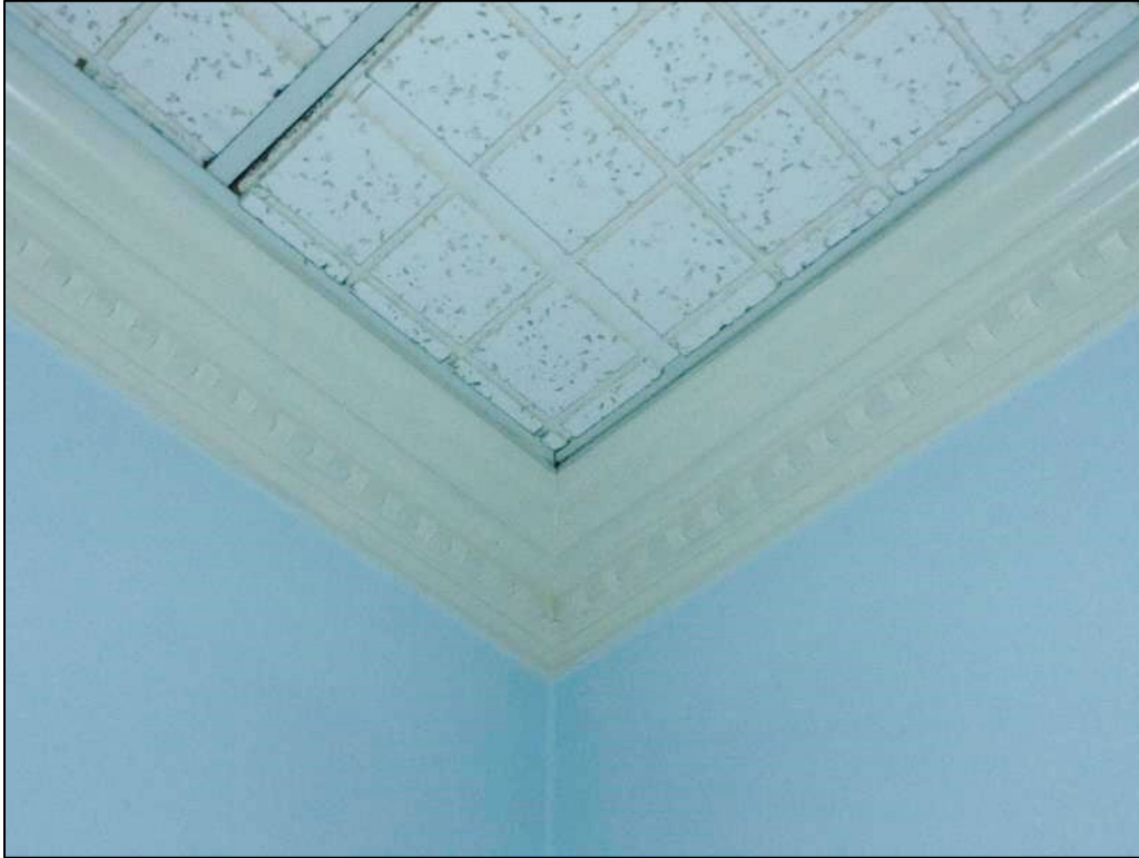
Figure 13: Third Floor at Intersection of Main Rectangular Section and Front Southeast Wing of 1944 Building – Showing Detail of Intact Original/Historic Denticulated Crown Molding (CPG, 2022)
