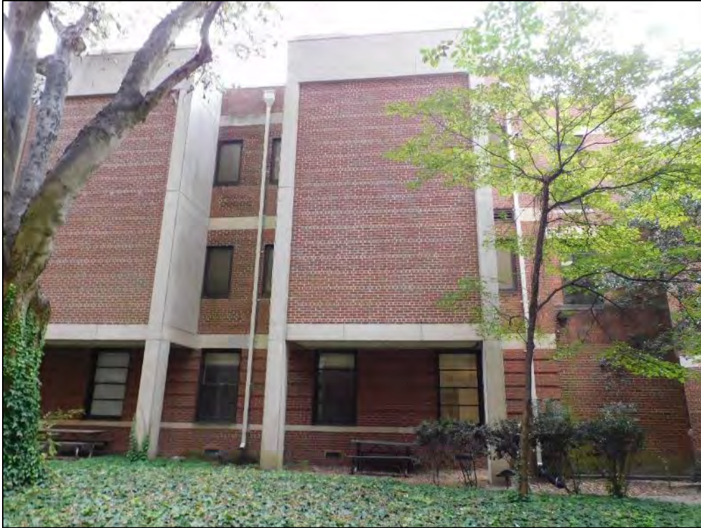
Figure 6: Northwest Elevation of Original 1944 Front Southeast Wing – Modern c. 1979 Bathroom Build-Outs in Foreground, Note Historic Windows and Walls Exposed at the First-Floor Level (CPG, 2022)
