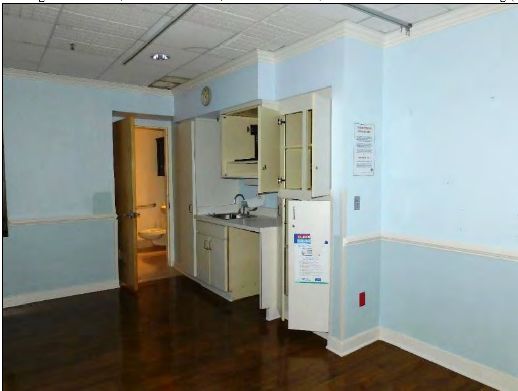
Figure 12: Third Floor, Front Southeast Wing of 1944 Building – Showing Intact Original/Historic Features Including Wood Floors, Wood Base Trim, Wood Chair Rail, and Denticulated Crown Molding (CPG, 2022)
