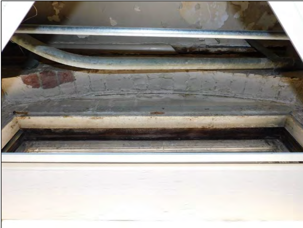
Figure 8: Historic Brick Arch Over First-Floor Historic Wood-sash Window, Intact Above Dropped ACT Ceiling, 1944 Building (CPG, 2022)
