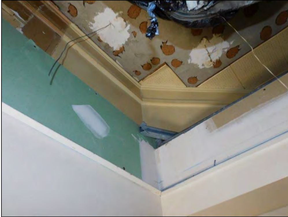
Figure 9: First Floor, Front Area of 1944 Building at Intersection of Main Rectangular Section and Front Northwest Wing – Showing Intact Original/Historic Trim/Crown Molding and Metal Ceiling Tiles Above the Current Dropped Acoustical Tile Ceiling (CPG, 2022)
