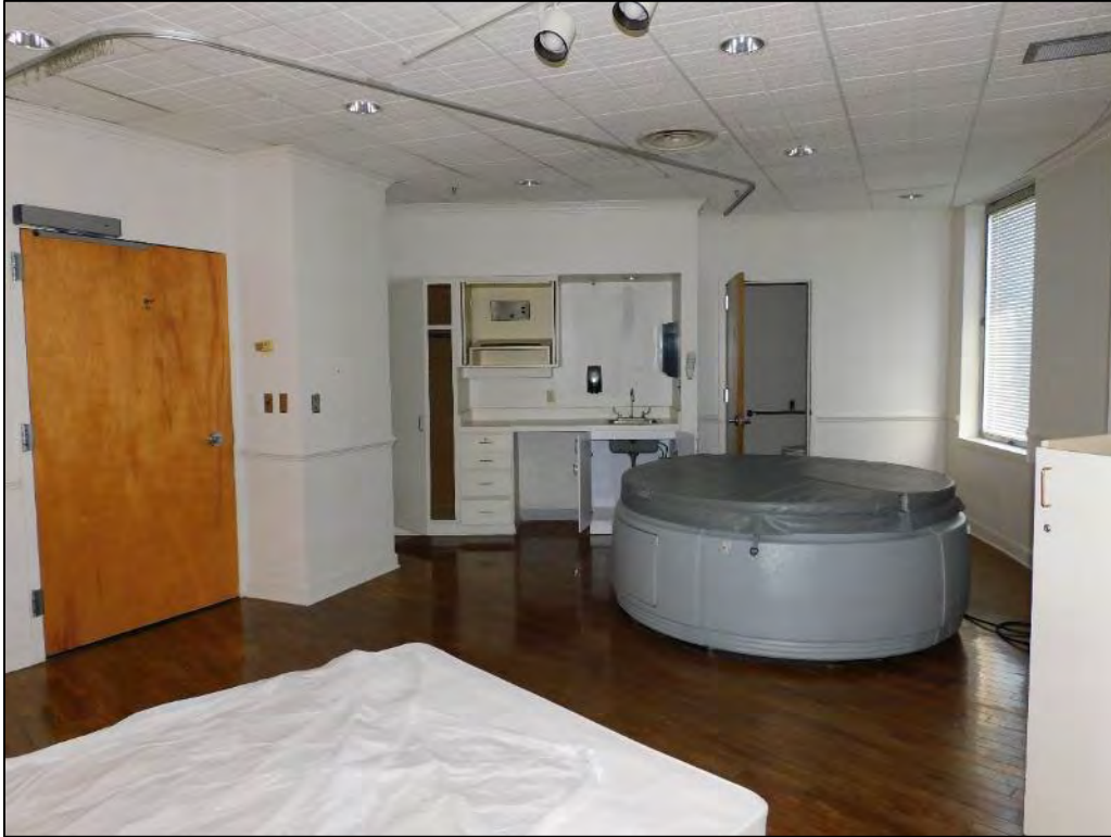
Figure 21: Third Floor, Maternity Ward – Showing Intact Original/Historic Features Including Wood Floors, Wood Base Trim, Wood Chair Rail, and Denticulated Crown Molding (CPG, 2022)
