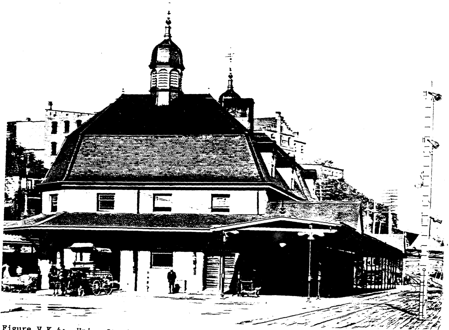
Figure V.K.4: Union Station (demolished), Lynchburg. Source: Lynchburg- An Architectural History.
