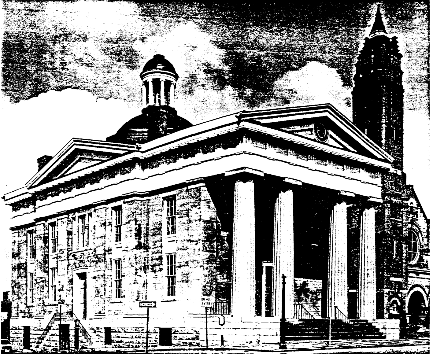
Figure V.D.1: City Courthouse (built 1851-1855), Lynchburg. Source: Lynchburg - An Architectural History.
