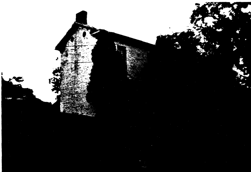
Figure V.C.4: A typical I-House located in the Diamond Hill neighborhood. Source: Greenhorne & O'Mara, Inc.
