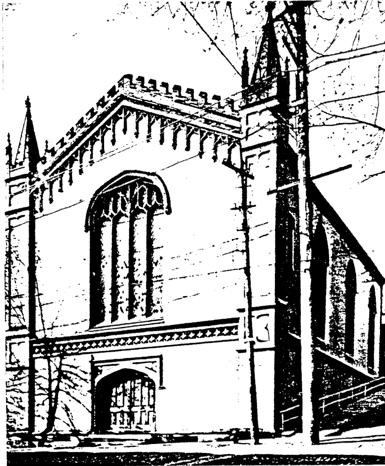
Figure V.H.1: Former St. Paul's Episcopal Church (demolished). Source: Lynchburg - An Architectural History.
