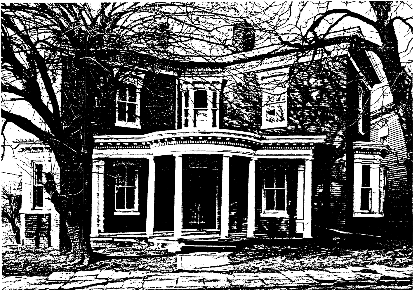
Figure V.R.3: Robert C. Burkholder House (1875). Source: Lynchburg-An Architectural History.
