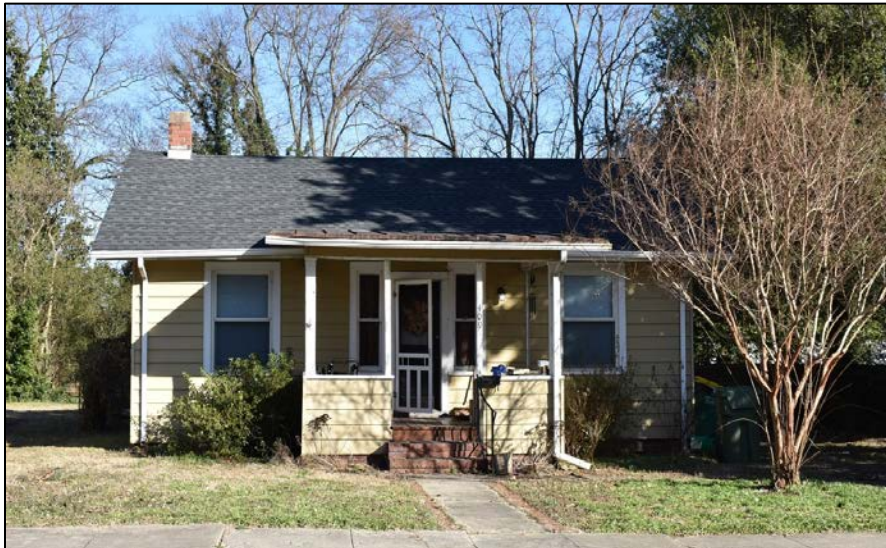
Figure 16. “The Forsyth” in “A Village” at 409 Brown Avenue (116-5133). Note the modified porch. March 2019.
