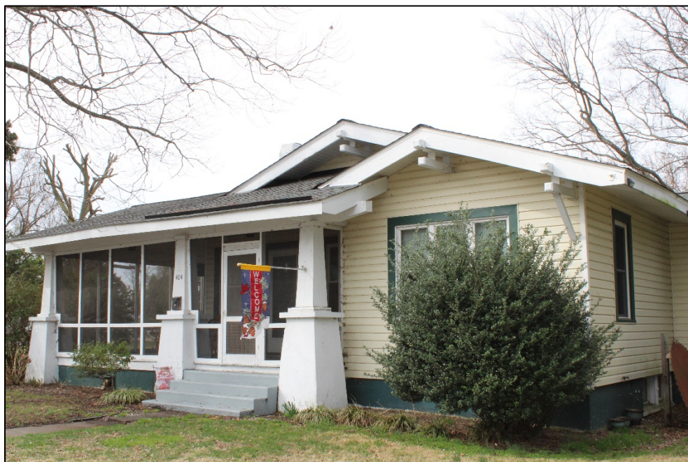
Figure 23. House at 404 Ramsey Avenue (116-5147), an example of the Plaza model of Aladdin kit houses. Note that the installation of vinyl siding has not obscured the distinctive eave brackets. March 2019.
