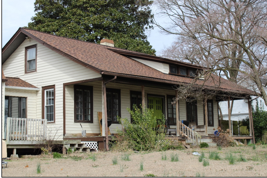
Figure 24. House at 401 Ramsey Avenue (116-5144). This example of the Kentucky model of Aladdin kit houses retains its original wooden casement windows on the original façade (which faces the river, on the opposite side of the house from Ramsey Avenue), but has replacement vinyl windows on the side and rear elevations. March 2019.
