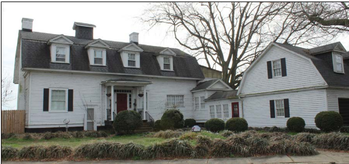
Figure 20. House at 403 Ramsey Avenue (116-5146). March 2019.
