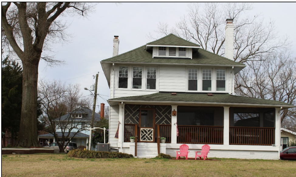
Figure 22. House at 405 Ramsey Avenue (not surveyed) and 402 Ramsey Avenue (in the background, 116-5145). Ramsey Avenue runs between these two houses; this is the modern-day rear of 405 Ramsey, the original front, facing towards the James River. Both houses are examples of the Wenonah model of Aladdin kit houses. March 2019.
