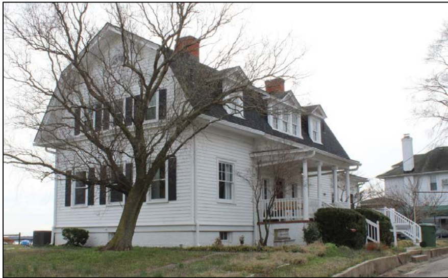
Figure 19. House at 407 Ramsey Avenue (116-5148). March 2019.
