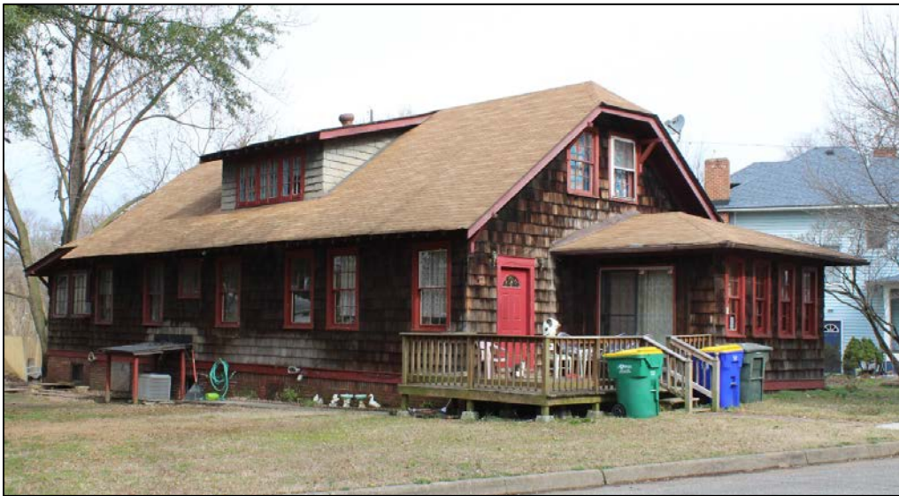
Figure 21. House at 400 Ramsey Avenue (116-5143). March 2019.
