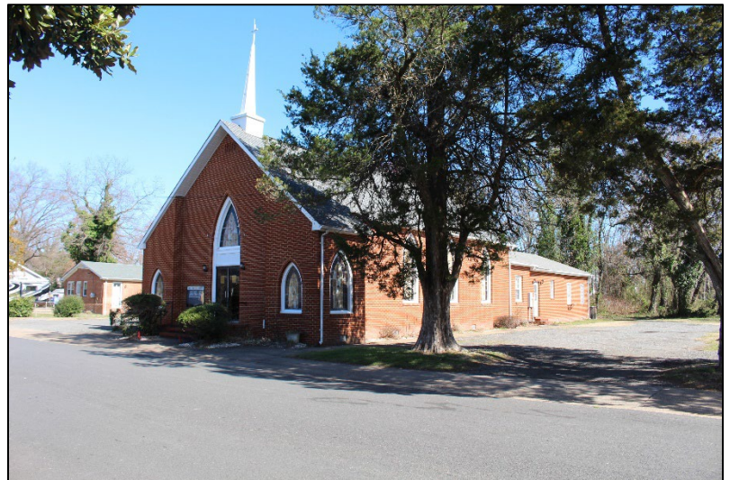
Photo 27. First Baptist Church of Colonial Beach (DHR ID #199-5138), looking northeast. (Robinson & Associates, 2023)
