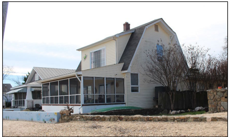
Photo 22. Circa 1930 house at 606 Potomac River Avenue (DHR ID #199-5145), looking southwest. (Robinson & Associates, 2023)
