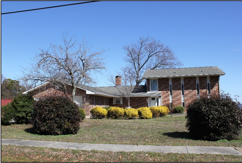
Photo 26. The 1968 house at 919 Bryant Avenue (DHR ID #199-5116), looking east. (Robinson & Associates, 2023)
