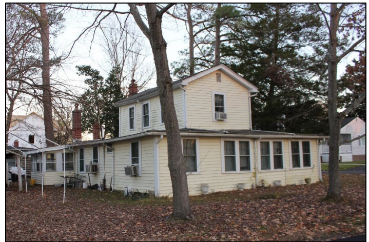
Photo 2. West elevation of 21 Chamberlayne Street (DHR ID #199-5063), looking southeast. (Robinson & Associates, 2022)
