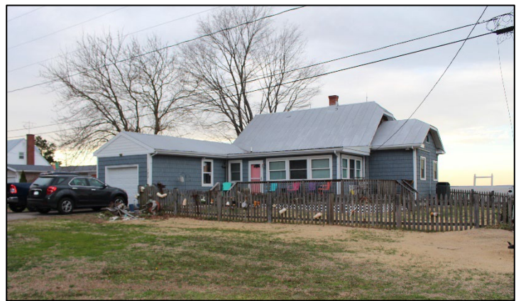
Photo 40. The former fishing shack at 123 Riverview Circle (DHR ID #199-5163). (Robinson & Associates, 2023)
