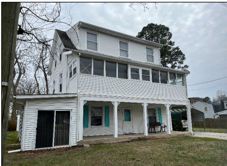
Photo 32. The two-and-a-half-story house at 20 9 th Street (DHR ID #199-5156, looking northwest. (Robinson & Associates, 2023)
