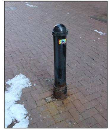
Figure 20. Nonhistoric bollard 2 nd Street SE, looking northeast. (Robinson & Associates, 2022)
