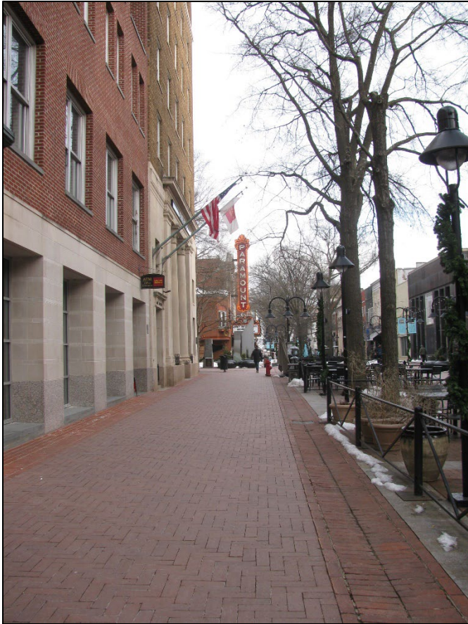
Figure 14. The LHA drainage runnels run east to west where the Main Street gutters and curbs had been located. Looking east. (Robinson & Associates, 2022)
