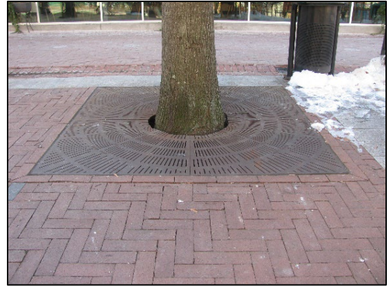
Figure 15. Tree grates were installed in the original portions of the Mall in 2009. Looking south. (Robinson & Associates, 2022)
