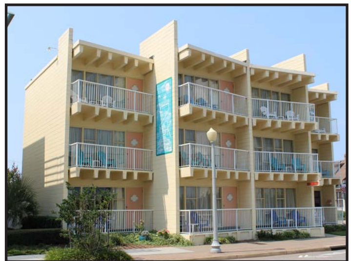
Figure 5.17 - Mid-20th Century hotels in the resort area offer an opportunity to promote heritage tourism, especially among younger generations interested in the aesthetics of mid-century modern.
