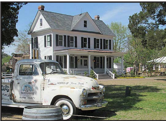
Figure 5.6 - Back Bay's Farmhouse Brewing Co. integrated a historic resource into new development
