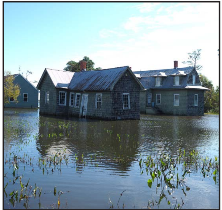
Figure 4.13 - Sunny day flooding at Horn Point Club in 2019.
