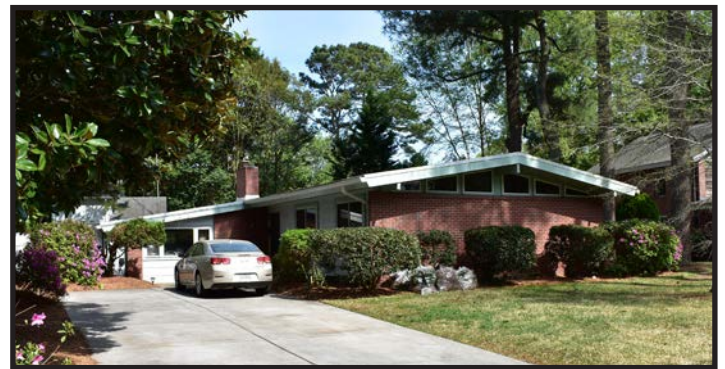
Figure 2.1 - 1312 Graham Road is located in the Woodhurst Historic District, which is listed in the Virginia Landmarks Register (VLR) and has been recommended eligible for listing in the National Register of Historic Places (NRHP) by the Virginia Department of Historic Resources (DHR).
