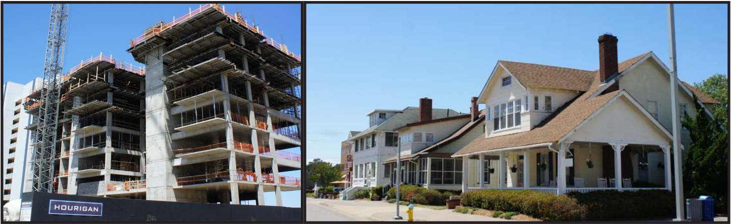
Figures 5.14 & 5.15 - At the left is a high-rise hotel being built on the former Belvedere Hotel location along the beach on Atlantic Avenue. Not far away is a group of cottages (at right) still intact and part of the Cutty Sark Motel. The cottages face development pressures due to the high value of land at the oceanfront.
