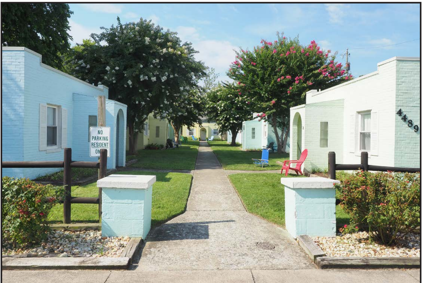
Figure 1.5 - Cottage Court, 4489 Lookout Road is located in the potential Chesapeake Beach Historic District, which has been determined potentially eligible for listing in the National Register of Historic Places (NRHP) and Virginia Landmarks Register (VLR) by the Virginia Department of Historic Resources (DHR).
