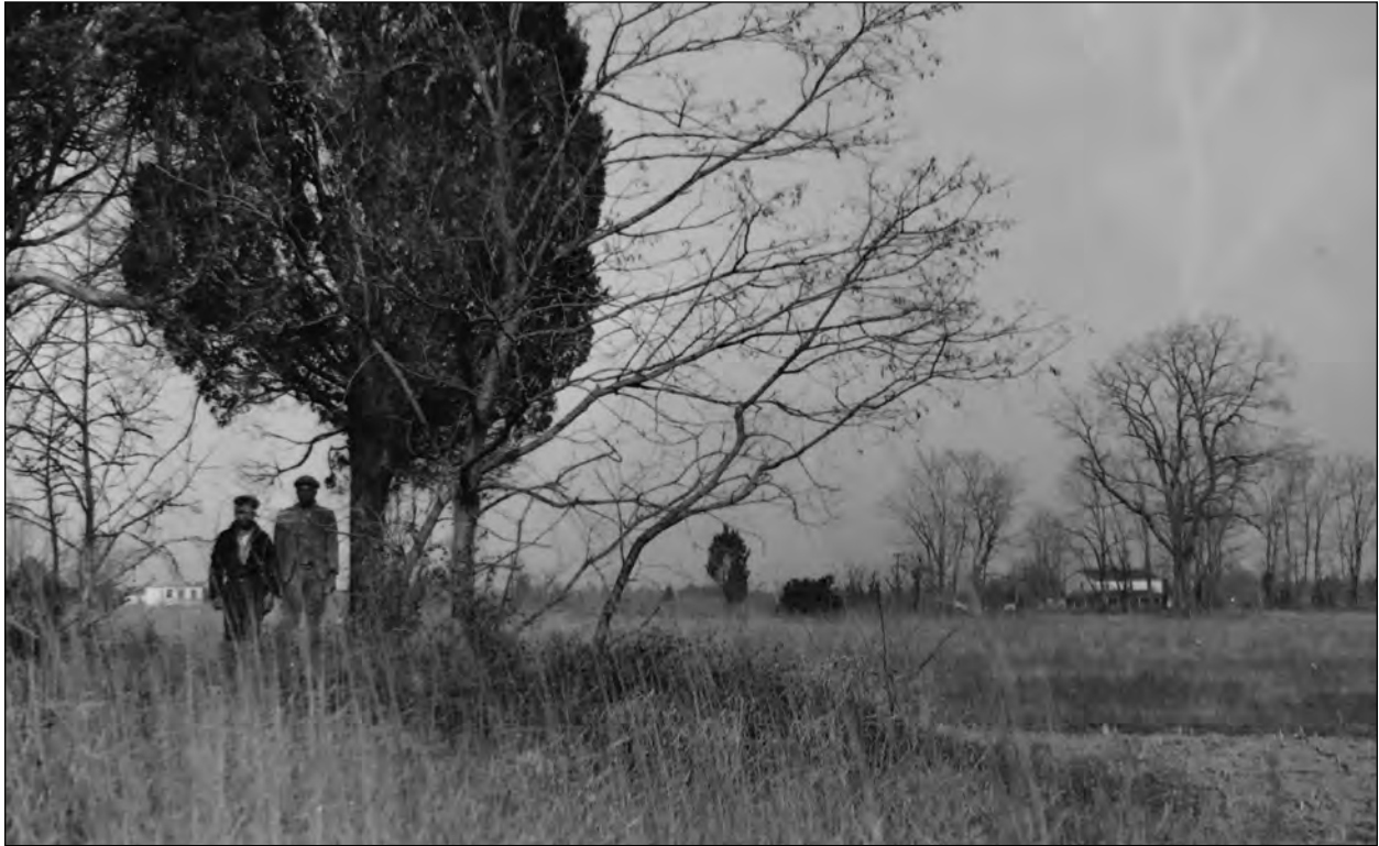
Figure 5.4 Two African American men standing near an old well, cedar trees, and an orchard in the foreground. A locust tree near the birthplace and a house are in the background. Stewart fields had yet to be reforested. Originally captioned "Negro Boys Standing by the Old Well. Locust Tree on the Right" (Porter 1937).
