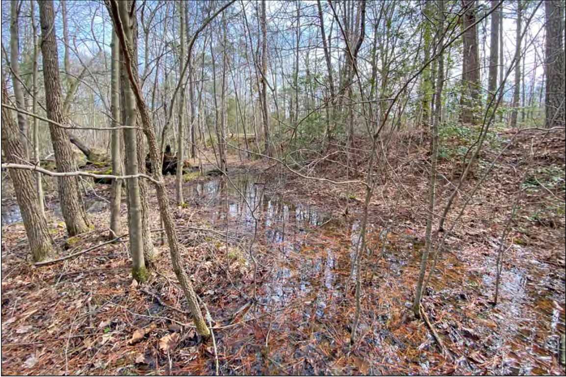
Figure 4.13 Abandoned mine excavation wall and pooling southwest of Watts Cemetery, view southeast.
