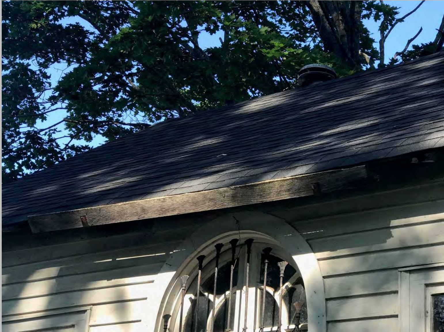
007-0128_Mint_Spring_Tavern_2022_Outbuilding_Post_Office_Wooden_Gutter
