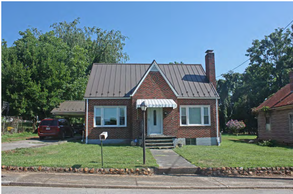
Figure 73. DHR # 033-5053. House at 255 Patterson Avenue, associated with the potential Patterson Avenue Historic District.
