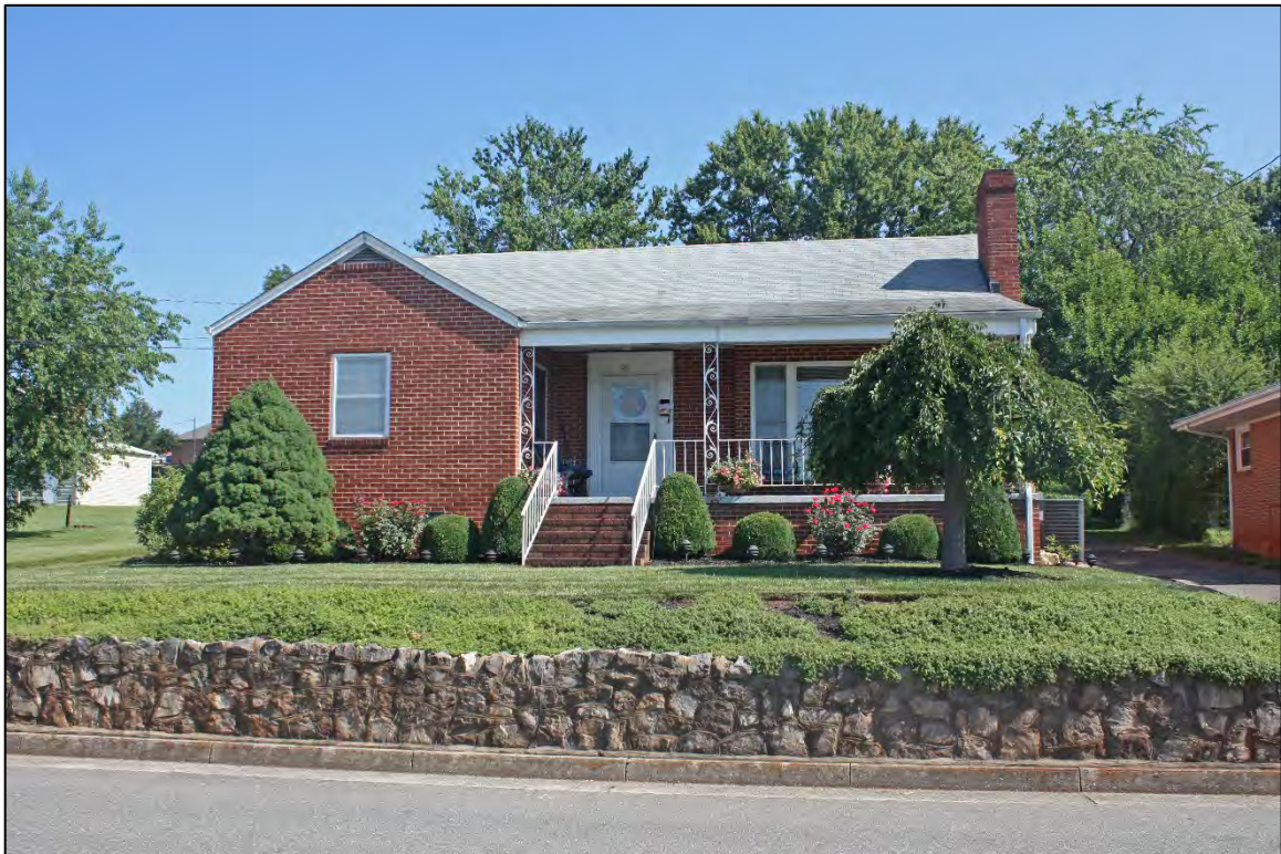
Figure 33. DHR # 157-5051. First Baptist Church Parsonage, 95 Patterson Avenue.
