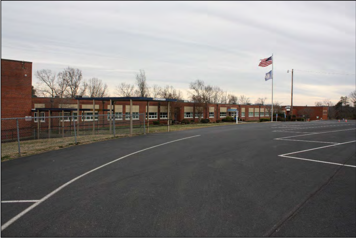
Figure 36. DHR # 157-5062. Lee M. Waid School, 540 East Court Street.
