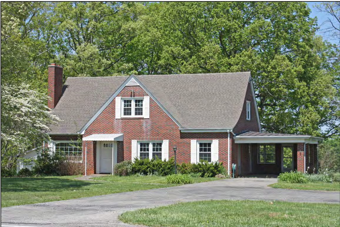
Figure 50. DHR # 033-5619. Beulah Baptist Church Parsonage.
