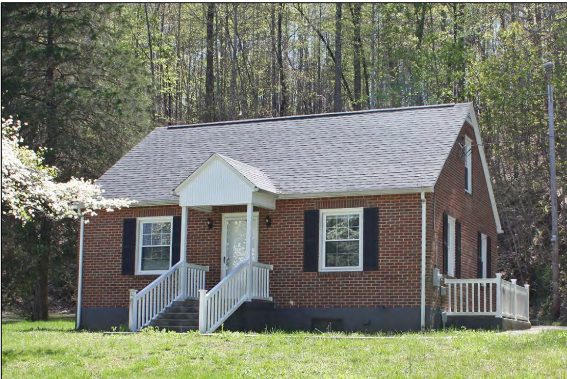
Figure 22. DHR # 033-5613. Minimal Traditional house, 10095 Franklin Street.
