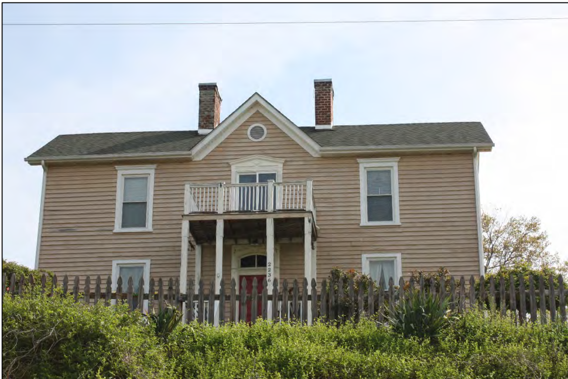
Figure 12. DHR # 033-5657. I-house, 2236 Dillons Mill Road.
