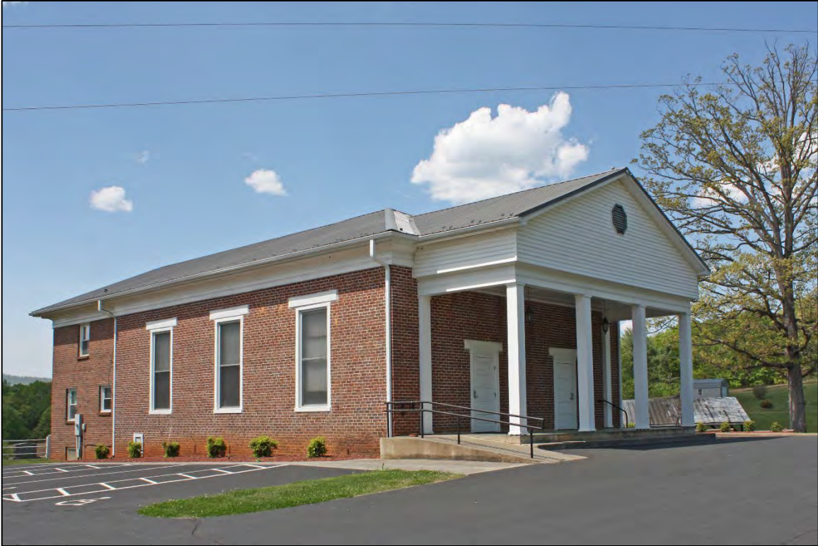
Figure 41. DHR # 033-0233. Fairmont Baptist Church.
