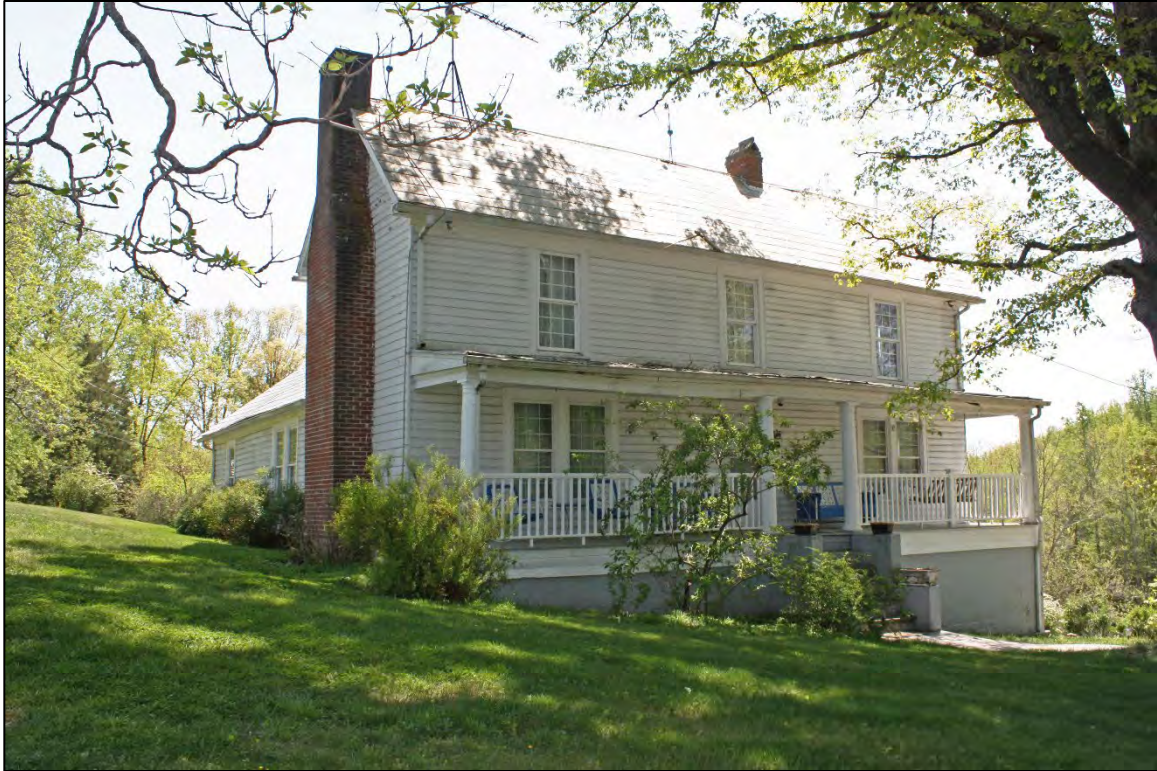
Figure 11. DHR # 033-5664. I-house, 1276 Knob Church Road.
