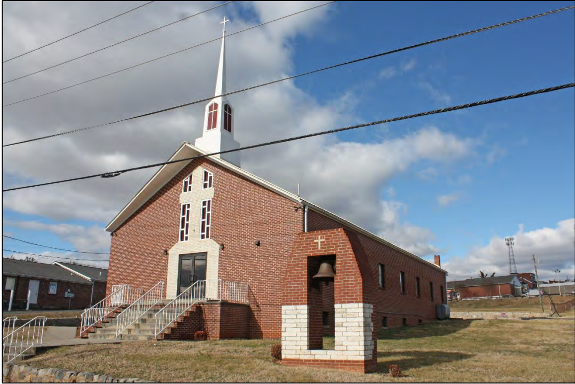
Figure 32. DHR # 157-5050. First Baptist Church, 45 Patterson Avenue.
