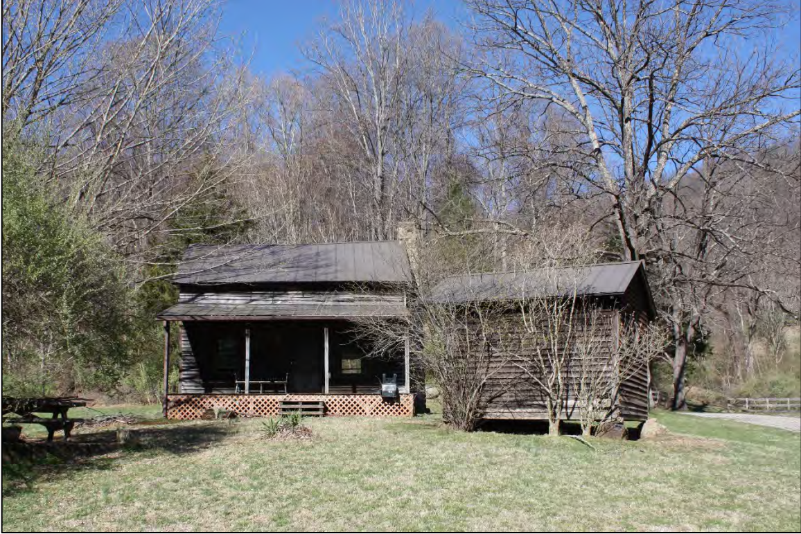
Figure 9. DHR # 033-5591. Log house, 1004 Webb Mountain Road.
