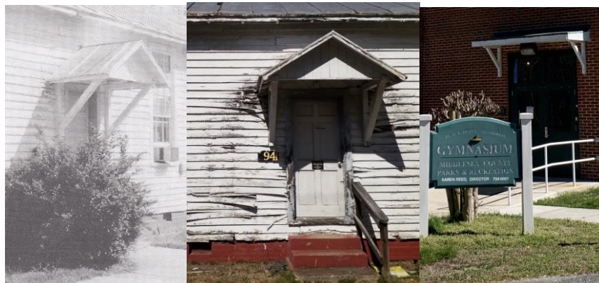
Figs. 4, 5, 6. Stick brackets on the front stoop of the c. 1941 Agricultural Shop and c. 1953 Gymnasium.
