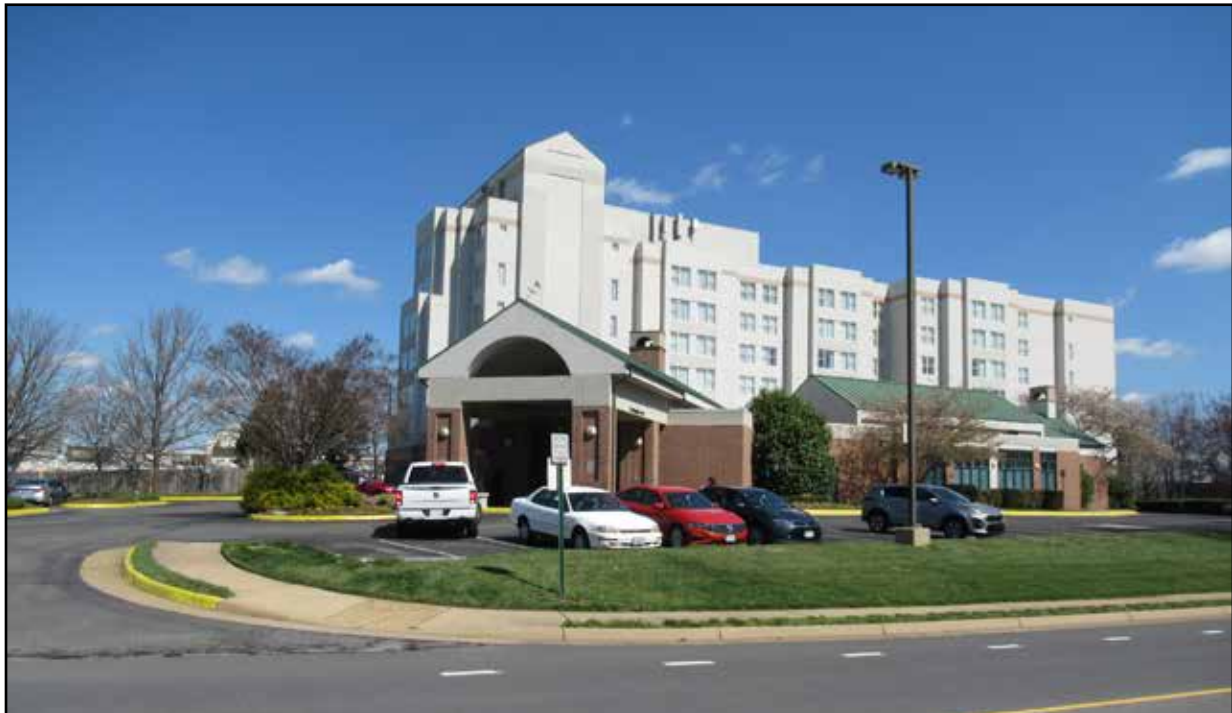
Figure 3.86. Merrifield area (029-6944), Porter Road, view to north.
