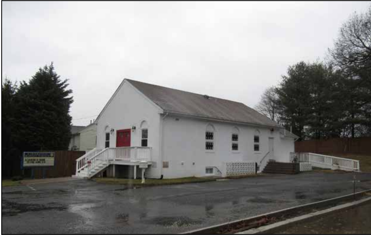
Figure 3.13. Cartersville Baptist Church (029-6015), southwest corner.
