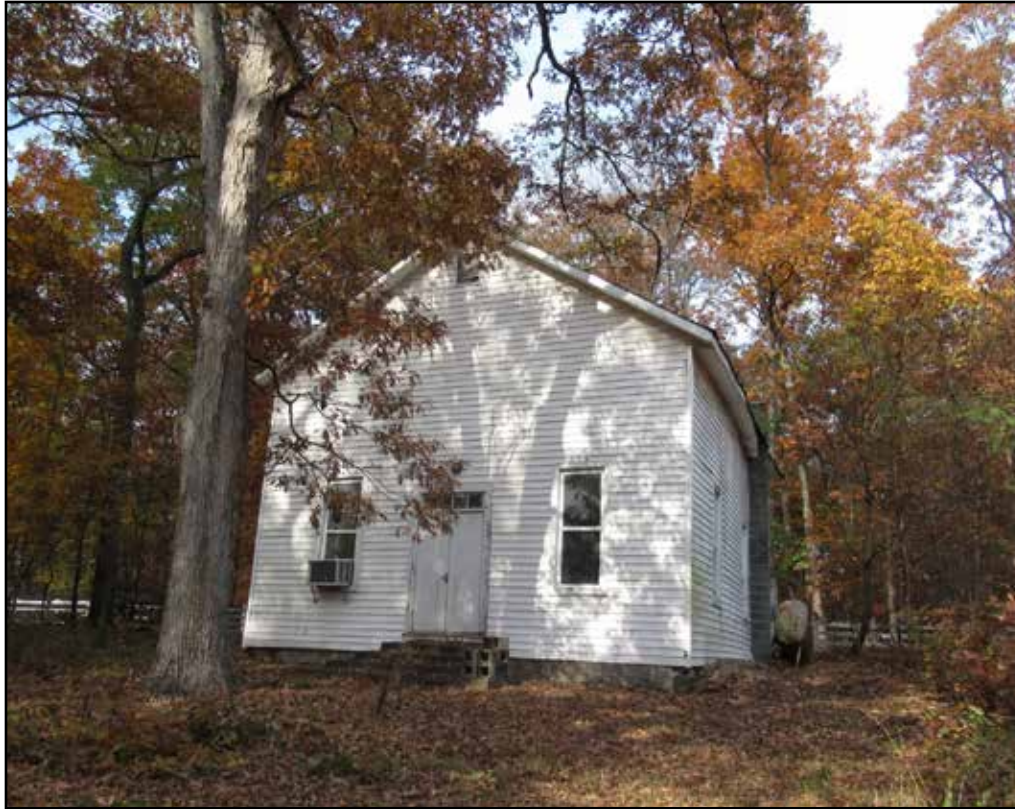
Figure 3.40. Cub Run Primitive Baptist Church (029-5321), facade.
