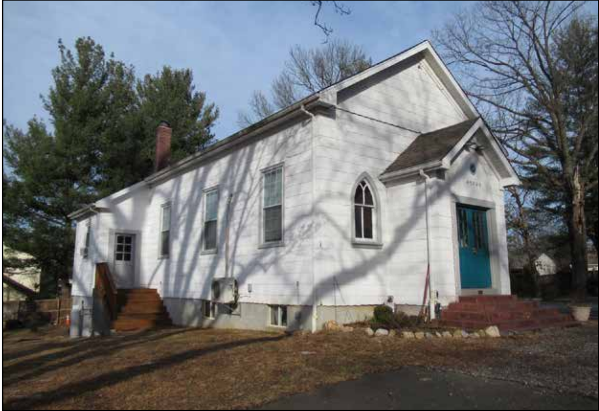
Figure 3.77. Little Zion Baptist Church (029-0376), southwest corner.
