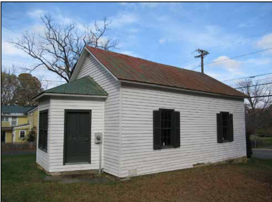
Figure 3.30. Clifton Primitive Baptist Church (194-0003-0024), south corner.
