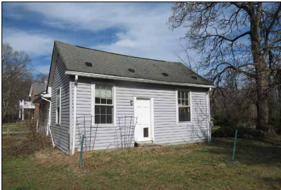
Figure 3.52. Gunston Hall area (029-6937), house on Harley Road.
