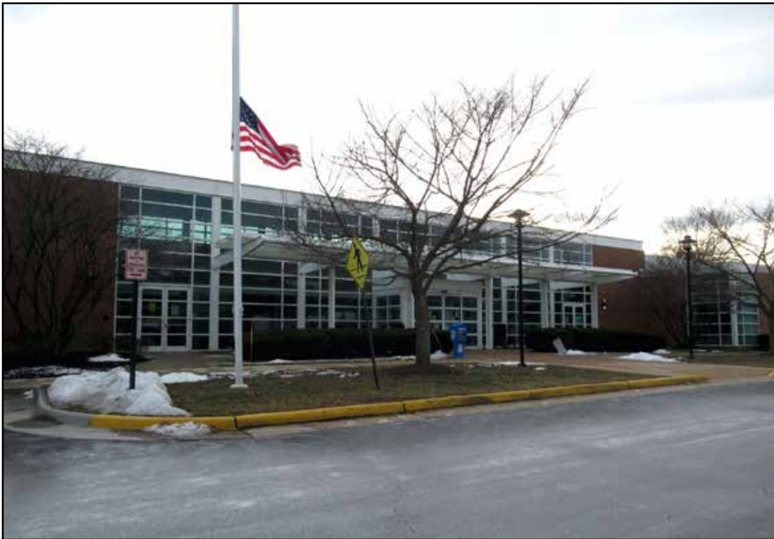
Figure 3.65. James Lee Community Center (029-6030), north entrance.
