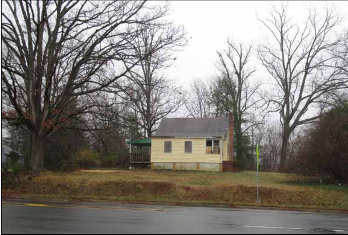
Figure 3.62. Ilda area ( 029-6932), Guinea Road at Walker Street, view to east.
