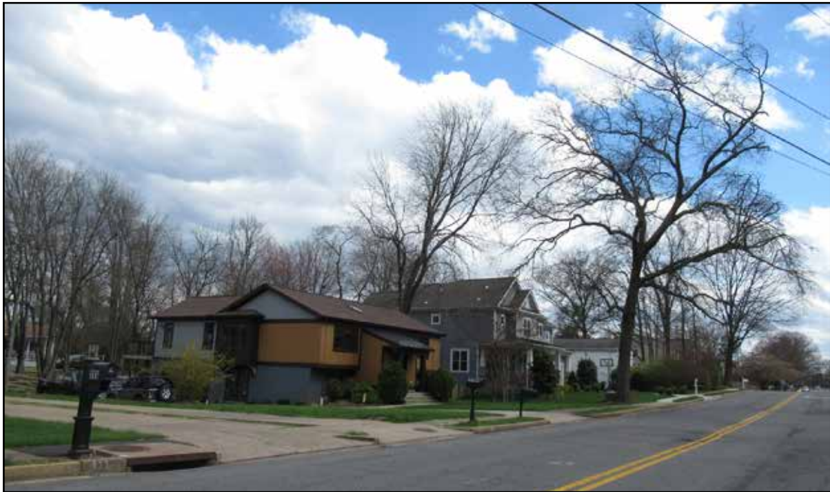
Figure 3.136. West End district (029-6942), 400 block of Nutley Street, view to the southeast.
