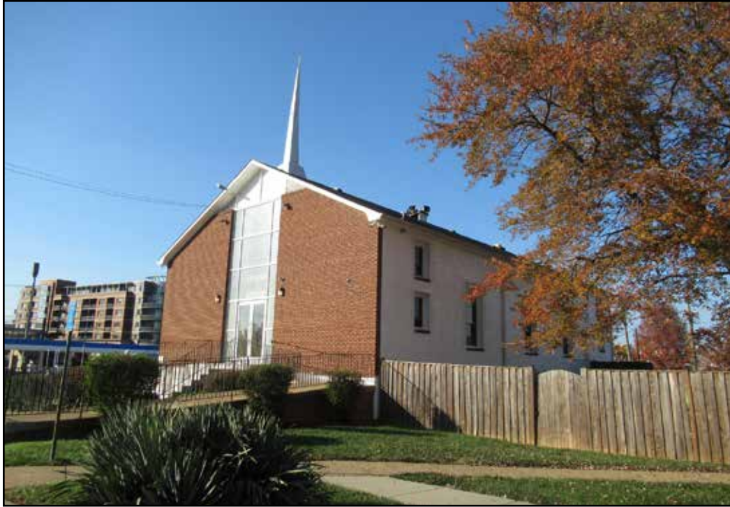
Figure 3.43. First Baptist Church of Merrifield (029-6888), southeast corner.
