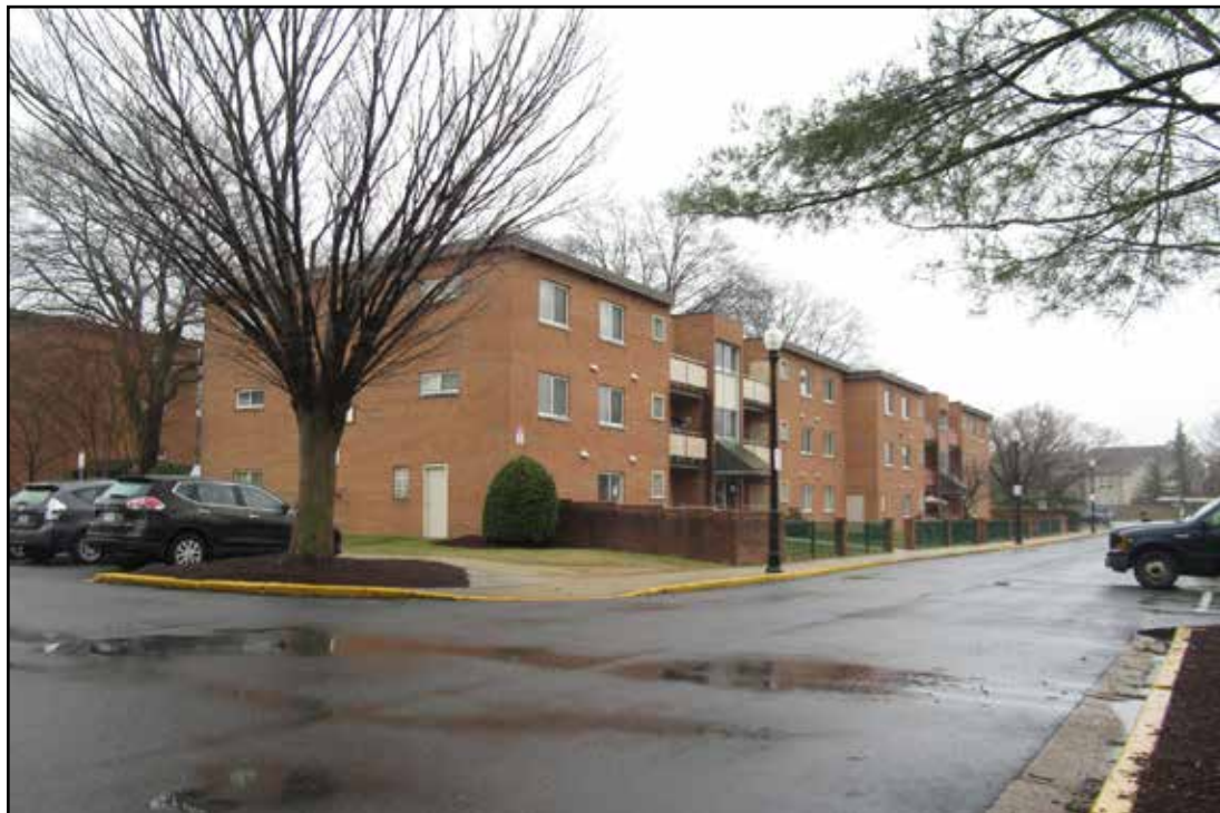
Figure 3.6. Bailey's Crossroads (029-6925), Oakview Apartments.
