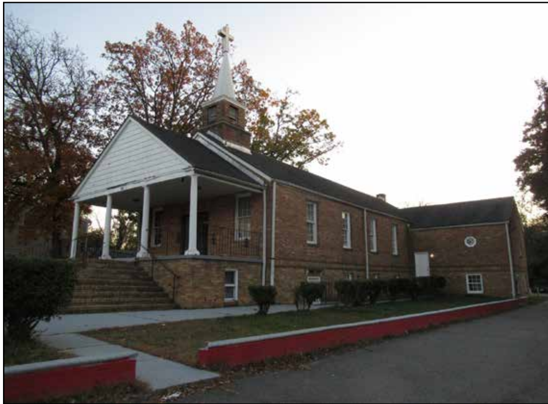
Figure 3.105. Scripture Church of Christ (029-6924), north corner.
