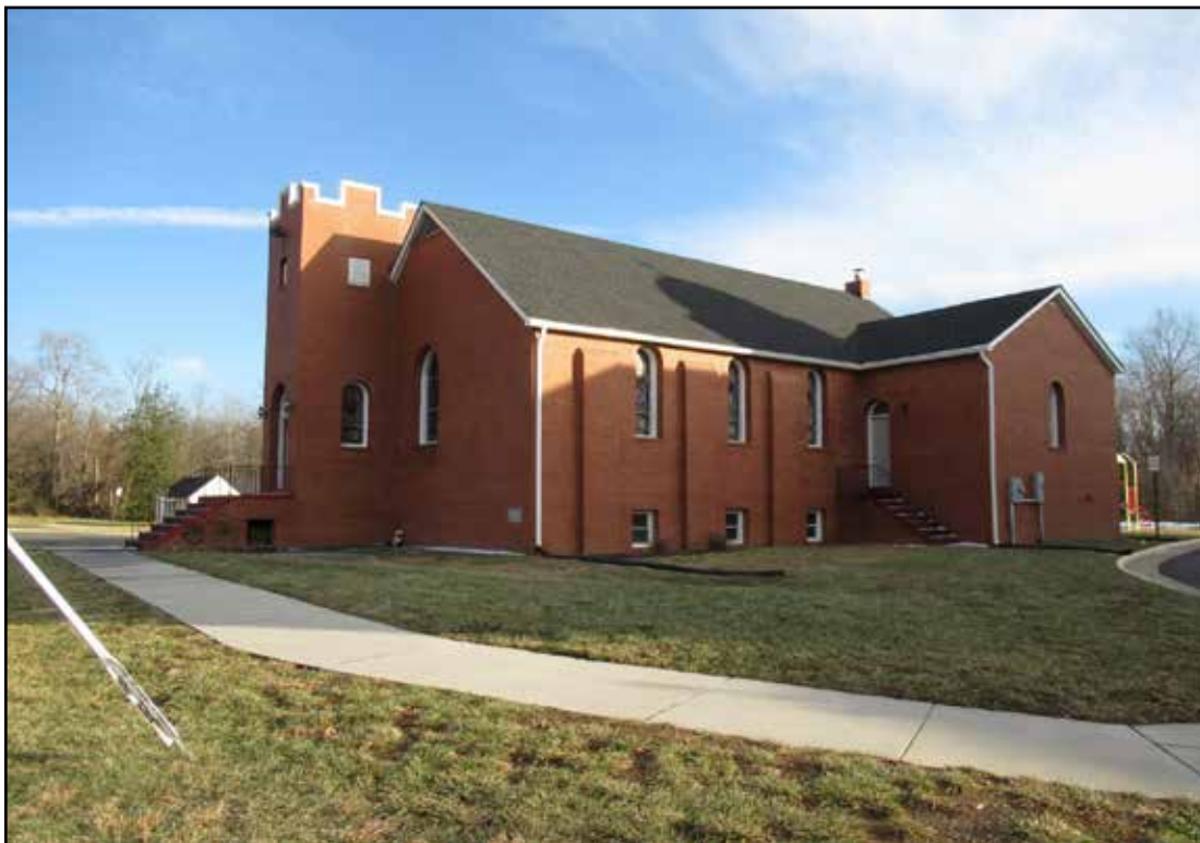
Figure 3.96. New Mount Zoar Baptist Church (029-6907), northwest corner.
