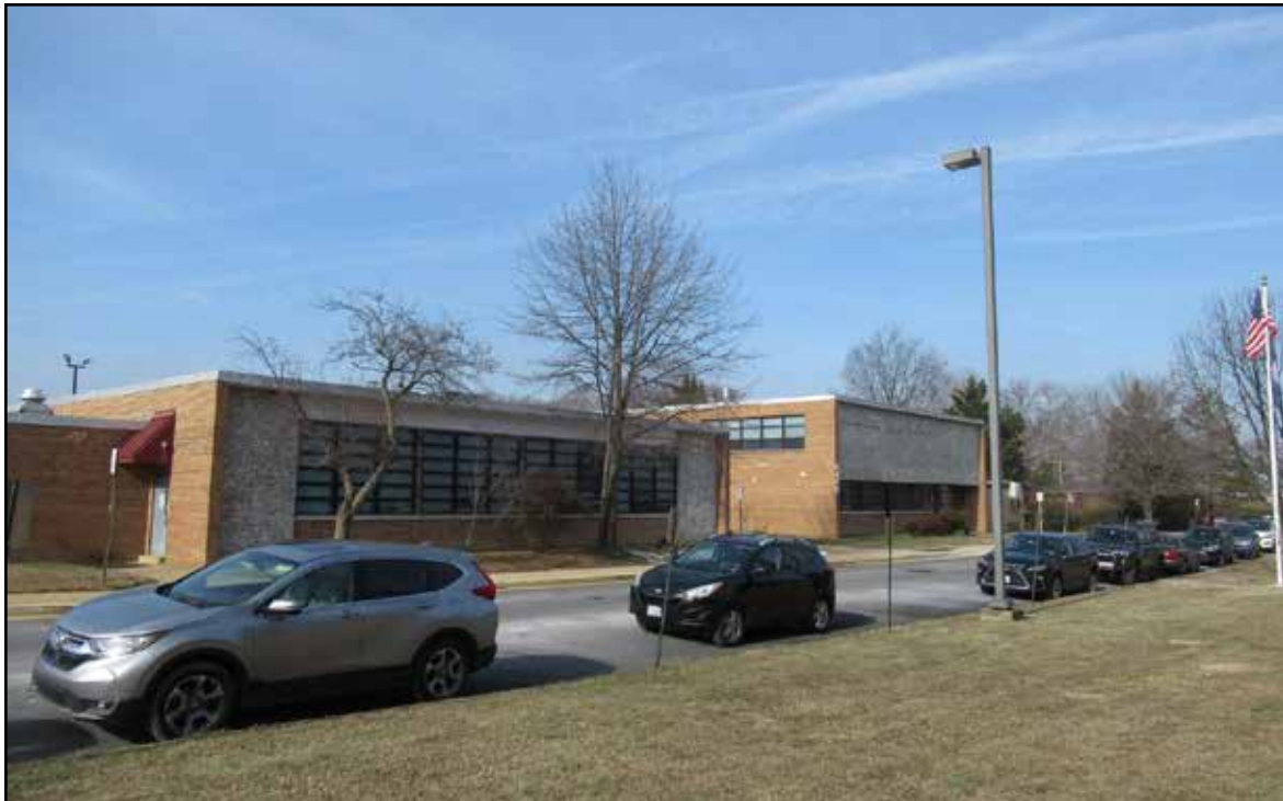
Figure 3.103. Quander Road School (029-6908), facade.
