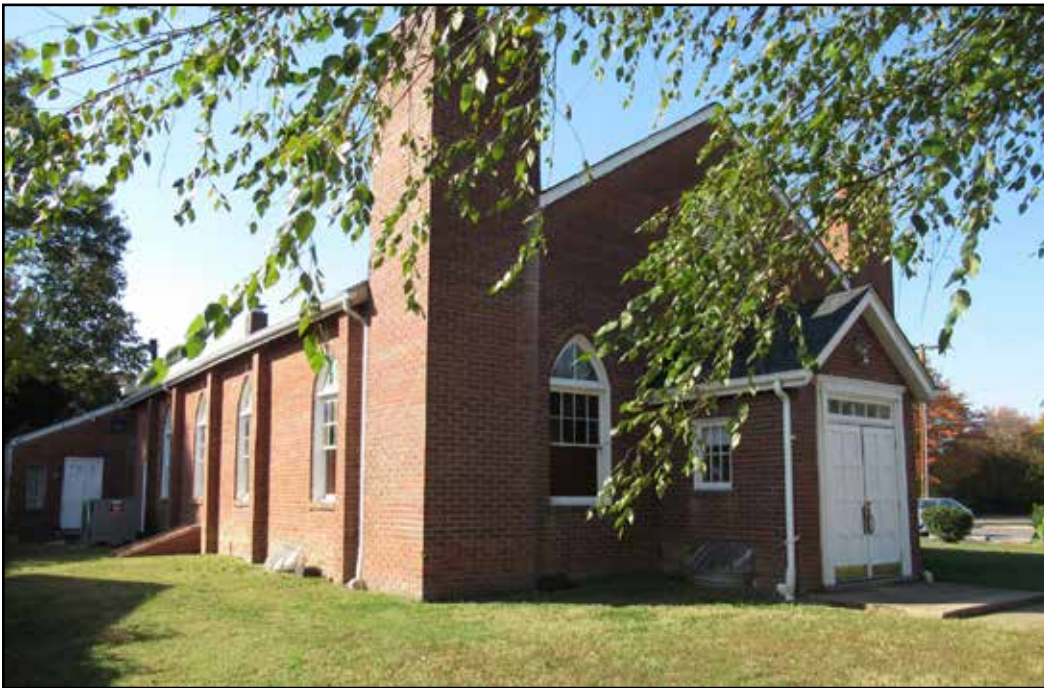
Figure 3.141. Woodlawn Methodist Church (029-6045), southeast corner.
