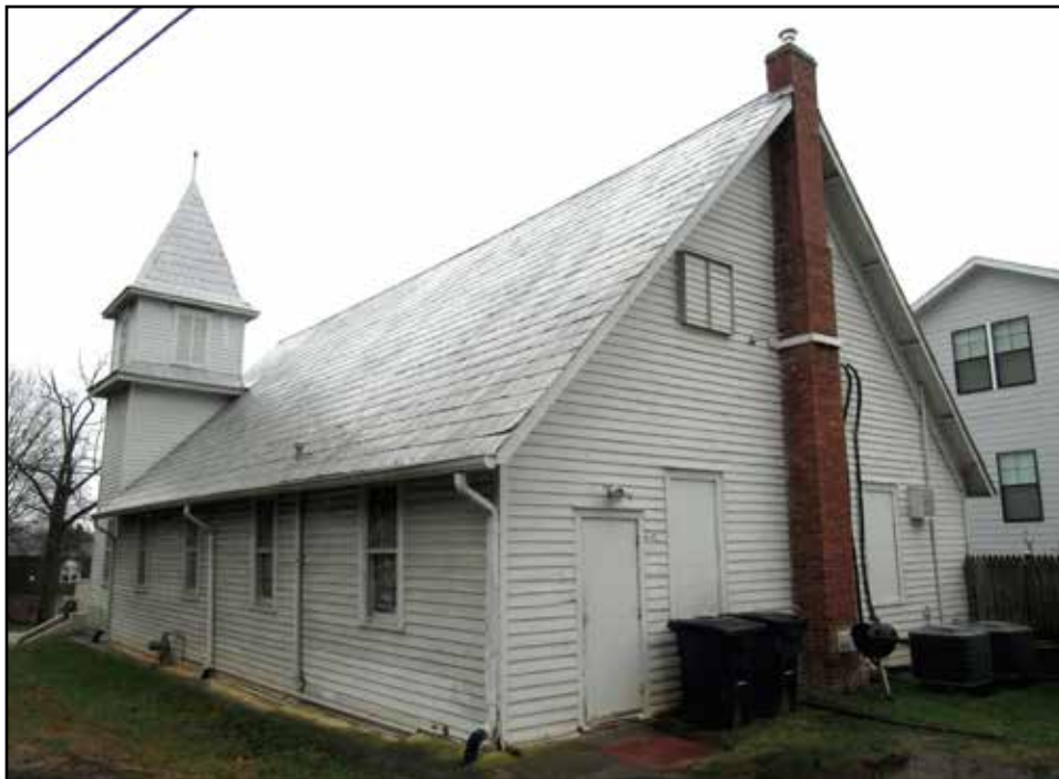
Figure 3.46. First Baptist Church of Vienna (153-5017), west corner.
