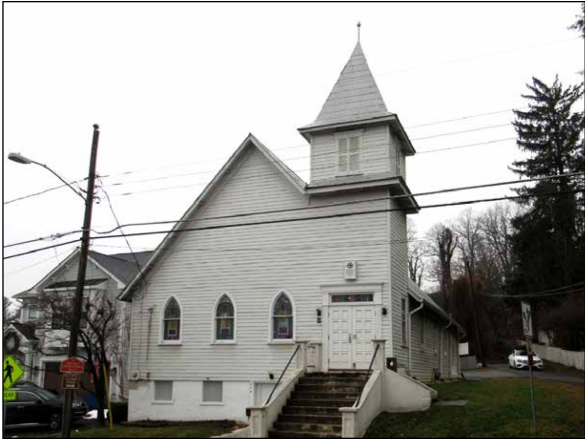
Figure 3.45. First Baptist Church of Vienna (153-5017), north corner.
