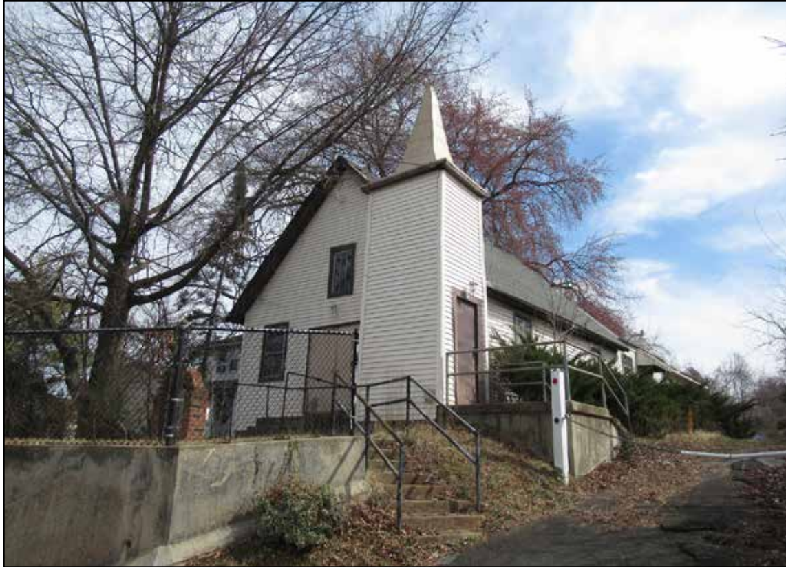
Figure 3.131. Third Baptist Church (029-6935), southwest corner.
