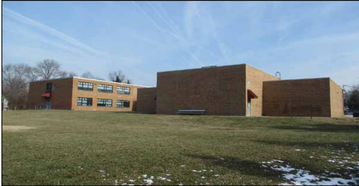
Figure 3.104. Quander Road School (029-6908), southwest corner.
