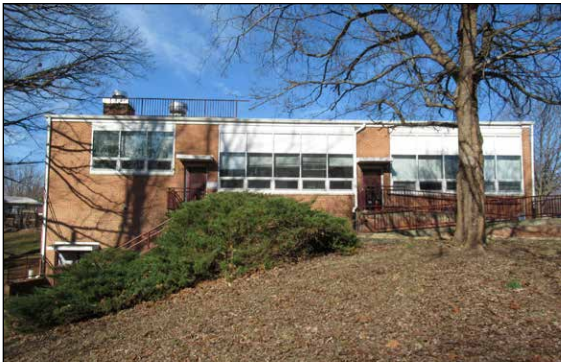
Figure 3.71. Lillian Carey Elementary School (029-6910), First Phase, south elevation.
