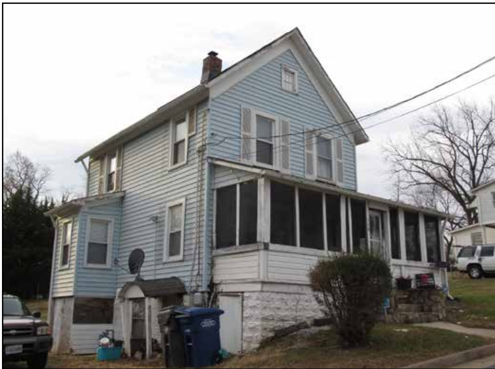
Figure 3.59. House, 114 Tinner Hill Road (029-6915), southeast corner.
