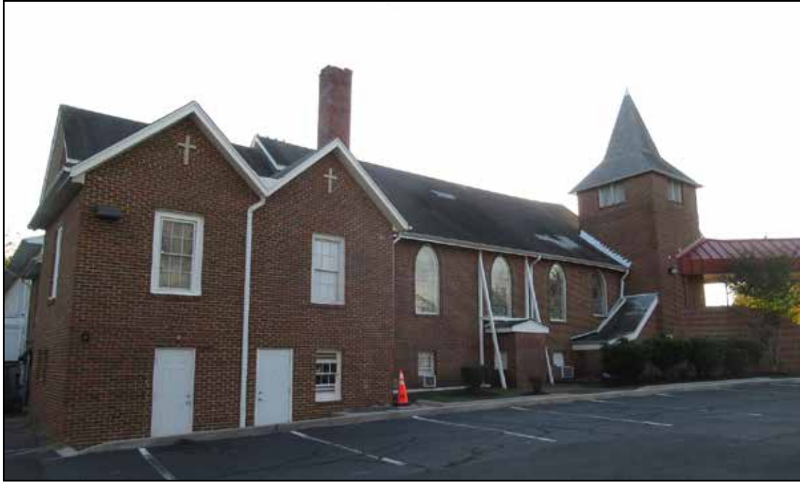
Figure 3.107. Second Baptist Church (029-6034), north elevation
