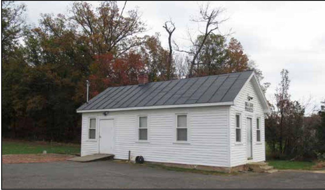
Figure 3.19. Chantilly Baptist Church (029-0307), Belle Cook building, southwest corner.
