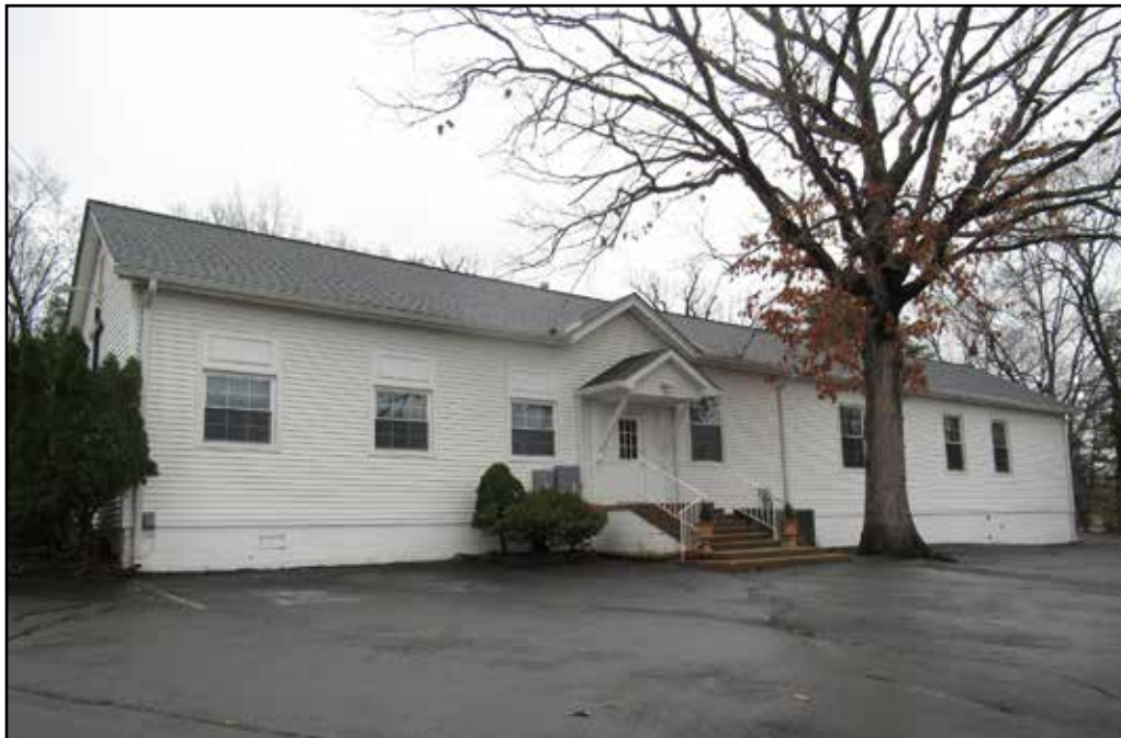
Figure 3.39. Cub Run Colored School/Centreville Assembly of God (029-6930), northwest elevation.
