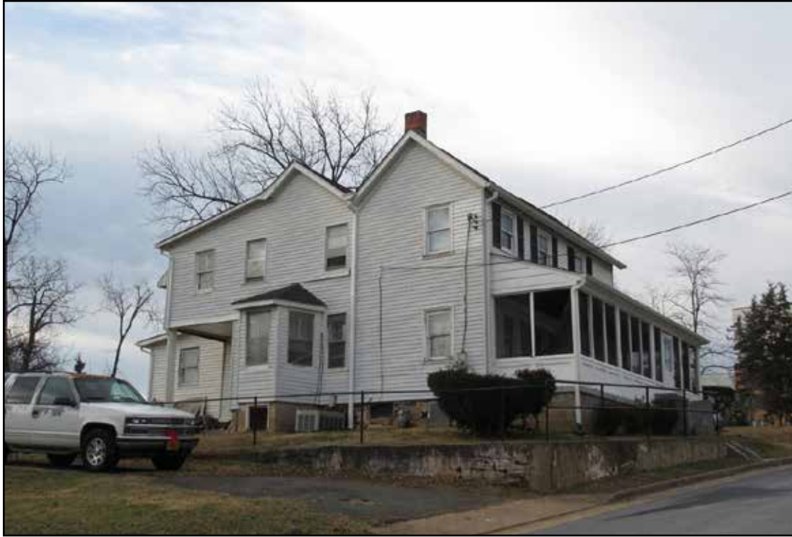
Figure 3.61. House, 110 Tinner Hill Road (029-6916), southeast corner.
