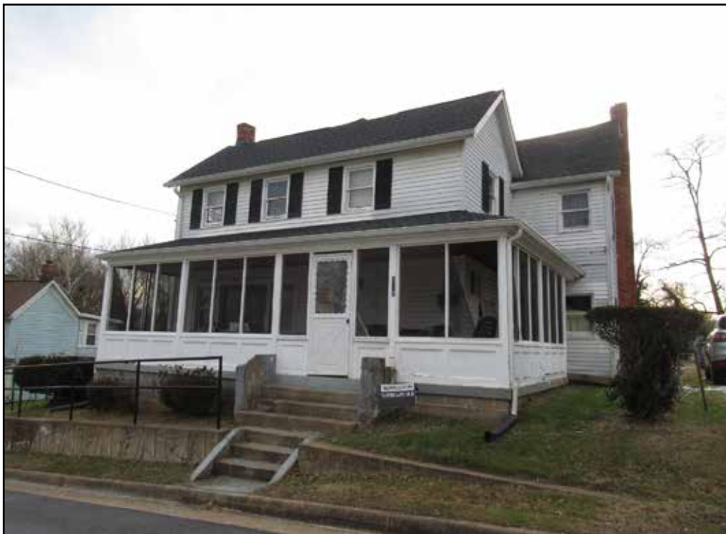
Figure 3.60. House, 110 Tinner Hill Road (029-6916), facade.
