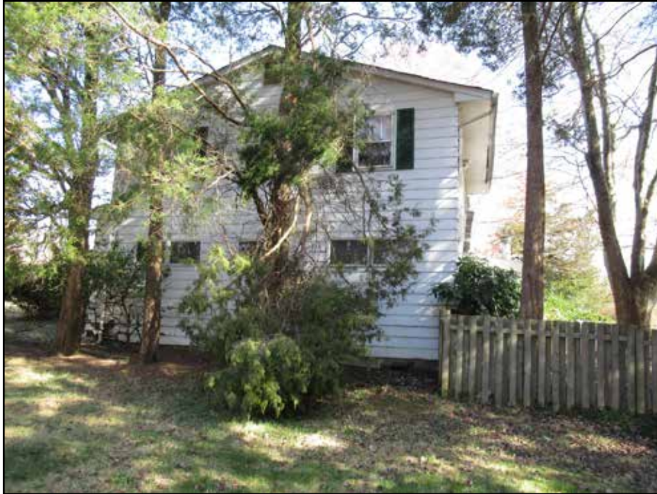
Figure 3.11. Bushrod House (029-6929), northwest elevation.
