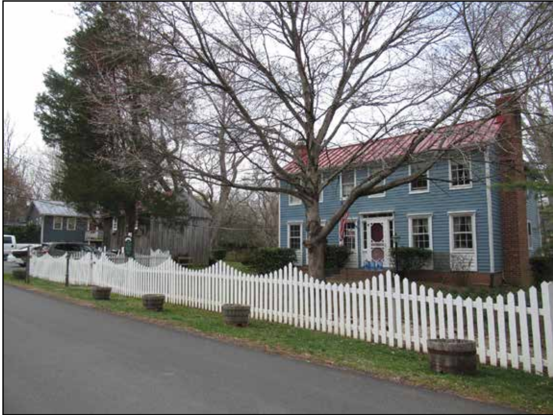
Figure 3.26. Clifton Historic District (194-0003), Chapel Street.
