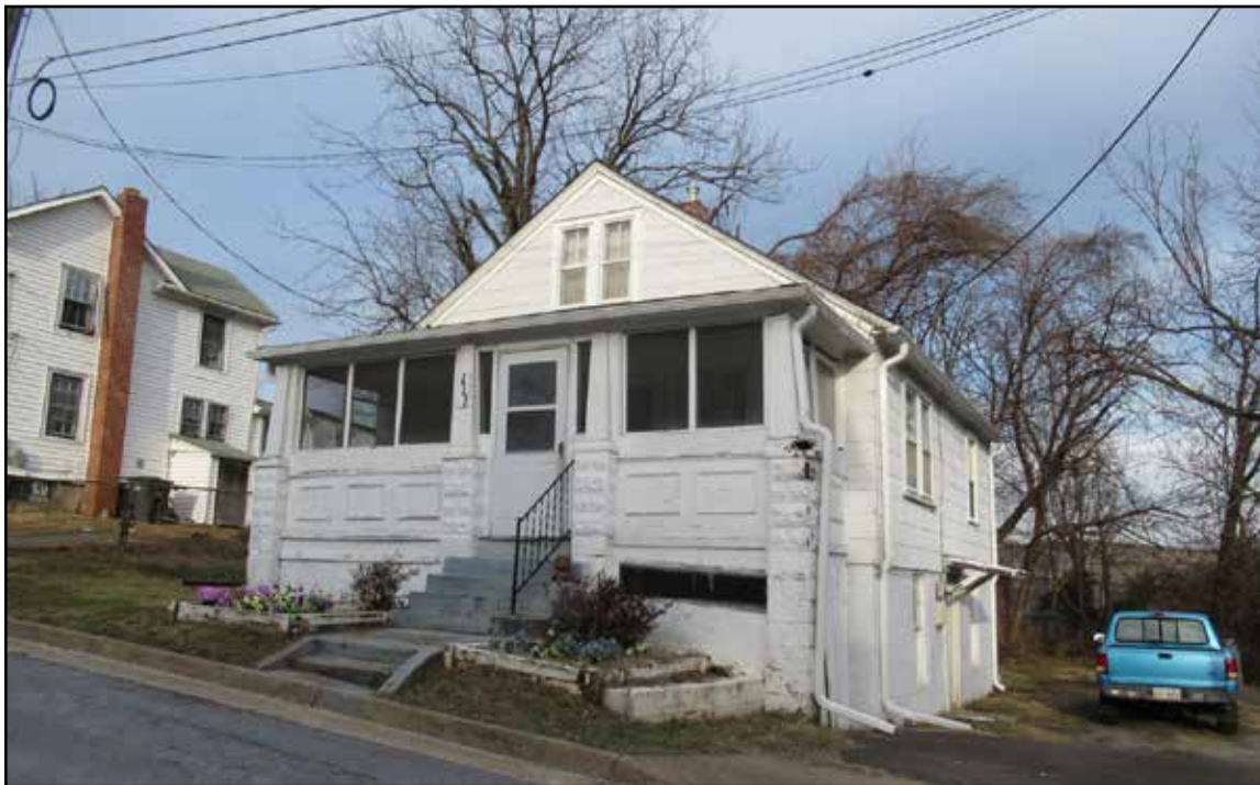
Figure 3.56. House, 111 Tinner Hill Road (029-6912), southwest corner.
