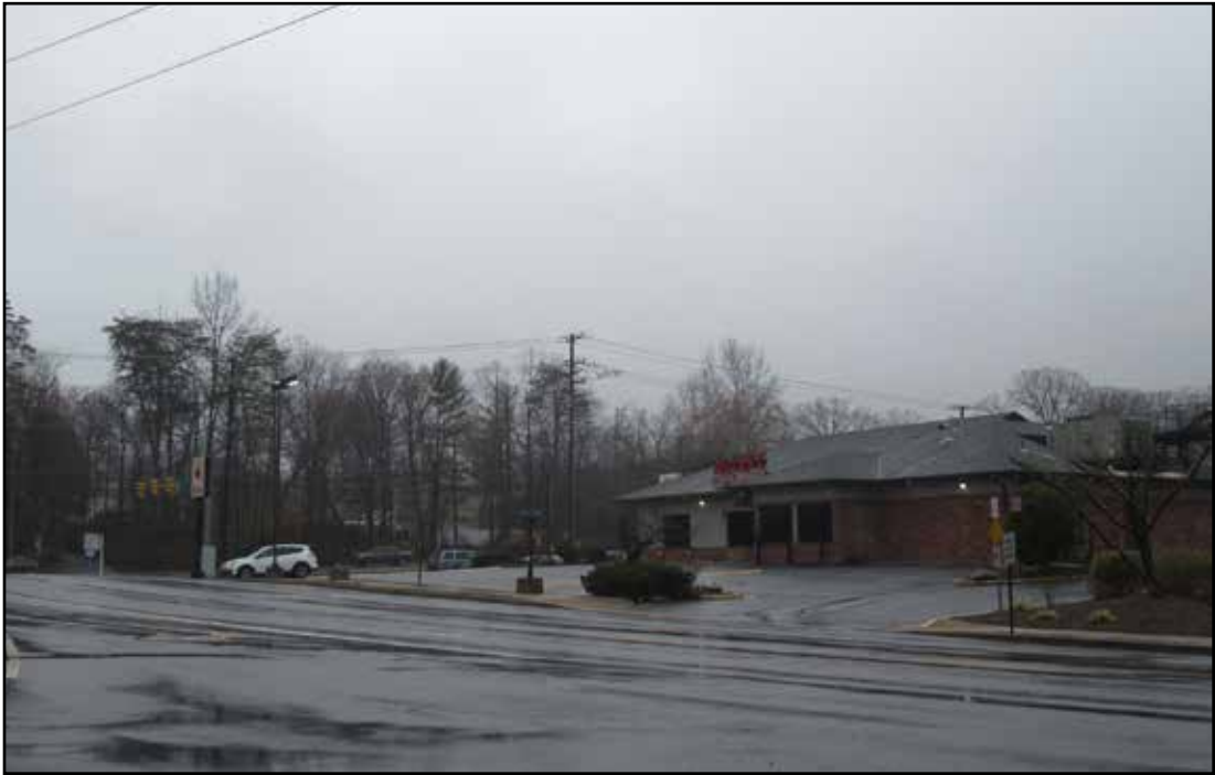
Figure 3.63. Ilda area (029-6932), Little River Turnpike at Prosperity Avenue, view to northwest.
