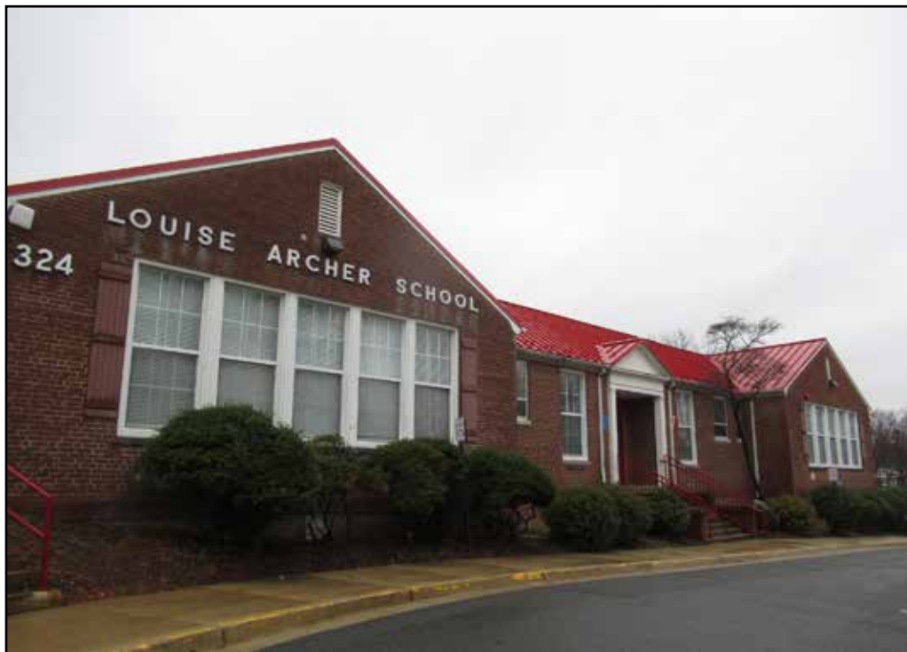
Figure 3.79. Louise Archer School (153-5021), facade.
