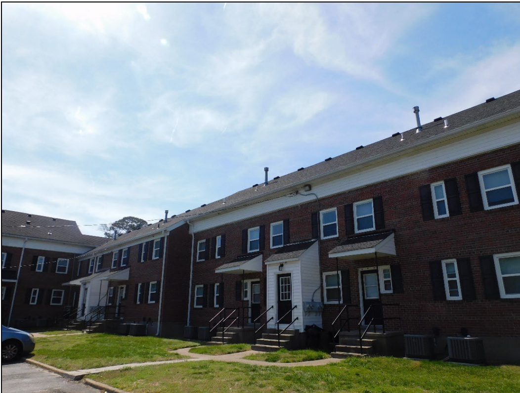
Figure 22. Representative Apartment Buildings at Sussex-at-Norfolk (Image Source: Commonwealth Preservation Group, 2024)
