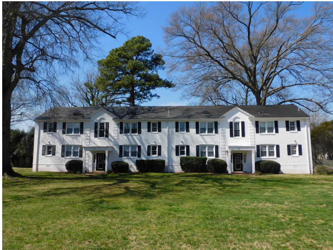
Figure 16. Representative Apartment Buildings at Bondale Apartments (Image Source: Commonwealth Preservation Group, 2024)
