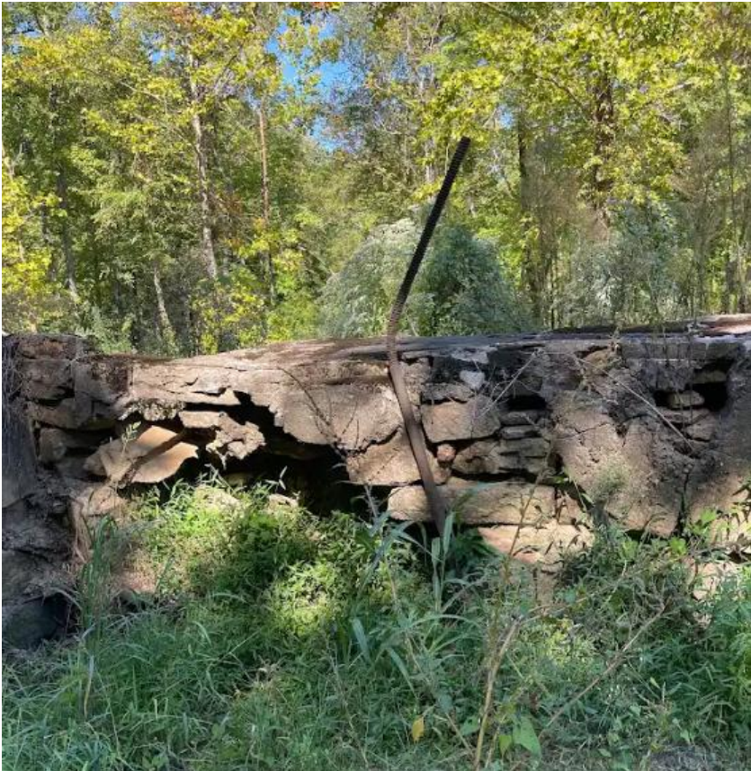
East end of milldam showing stonework with concrete lining and iron bar.
