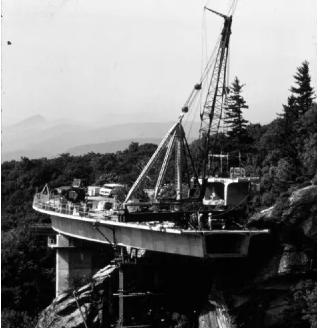
Figure 28. Construction of the Linn Cove Viaduct, ca. 1980. The completion of the technologically advanced precast concrete viaduct in 1983 allowed for the construction of the final section of the Parkway and its opening to its full length in 1987 (source: Blue Ridge Parkway Archives).
