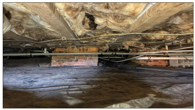
Crawlspace beneath the two-story section, looking towards the rear of the house at brick piers supporting the rear sill. October 2024.
