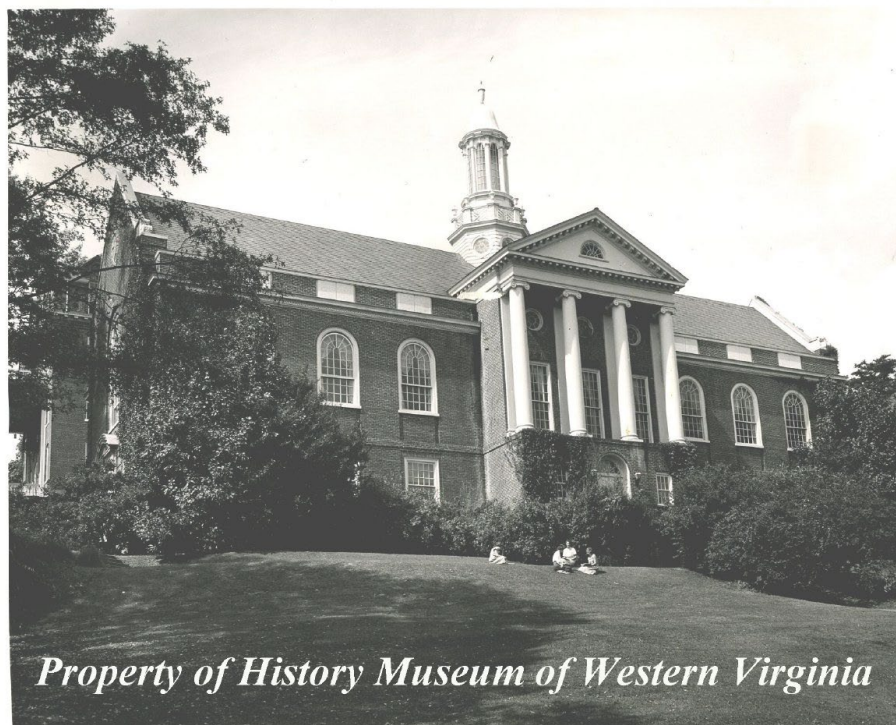
Figure 5: 1954 photo of Lipscomb Hall's Front (East) Elevation. Courtesy of the History Museum of Western Virginia.
