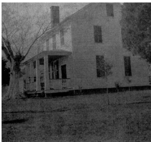
Figure 6: The north elevation pre-1900. Note that the first-floor west window has not yet been replaced. Note, too, the Victorian-era pattern-sawn porch pickets (seen also in Figure 4). Photo courtesy of the owner.
