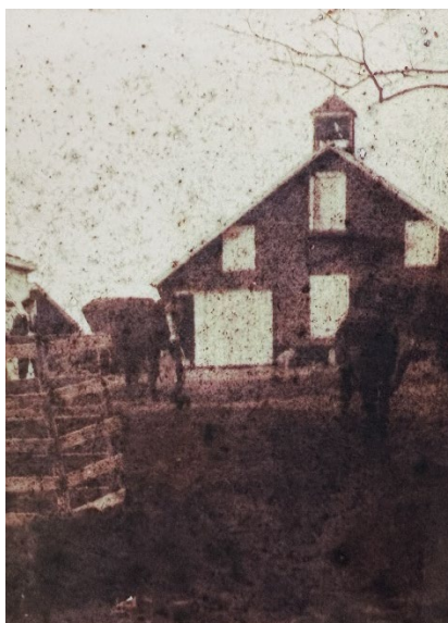
Figure 6: The barn pre-1900. Note that the additions have not yet been constructed and the fenestration has since been altered. Photo courtesy of the owner.
