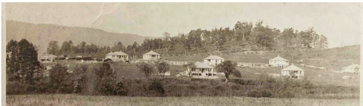
Figure 6 – Bacova employee housing under construction in 1920 looking roughly north from the current location of Lake Bacova. Lumber is stacked on the left side of the image waiting to be assembled. Courtesy Bath County Historical Society.
