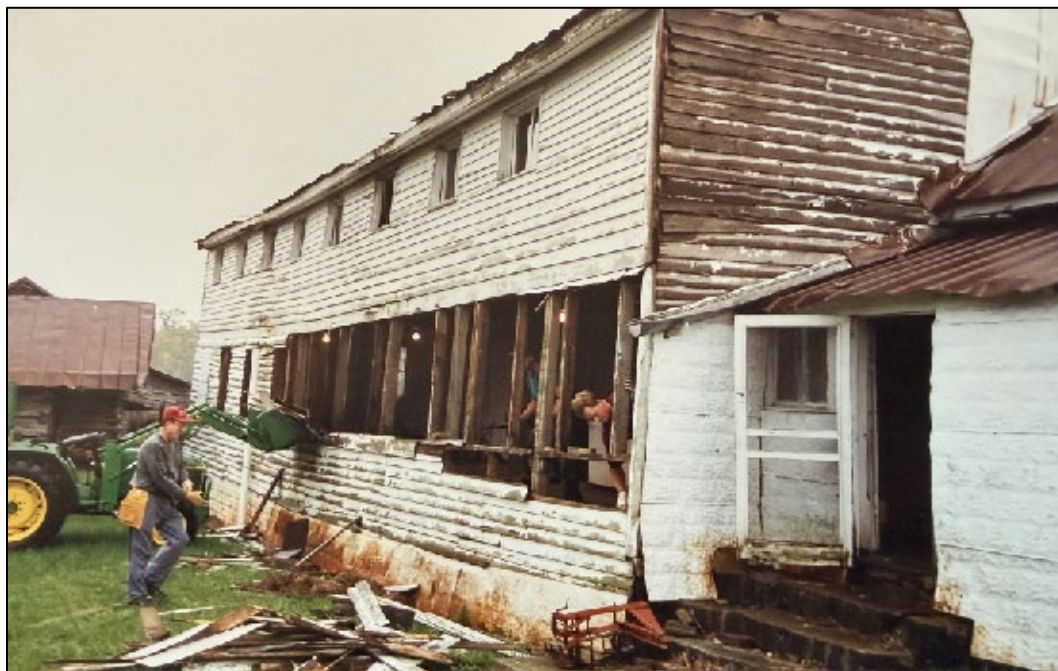
Fig. 3 Rear porch being dismantled, circa 1991.
