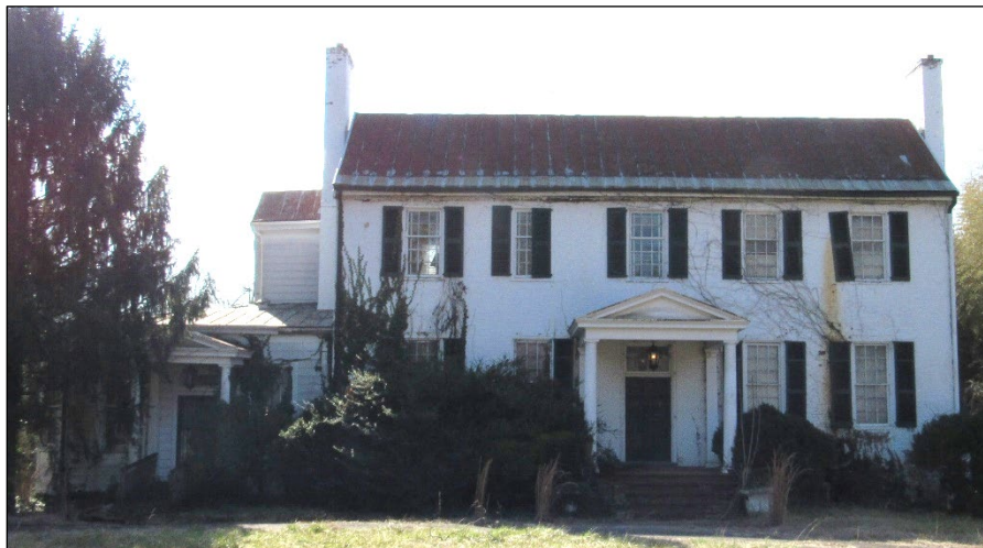
Photo 1: Brookbury, North Elevation (Gordineer 2024).
