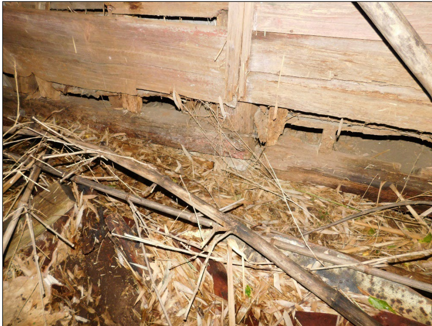
Photo 12: View of Sill Plates of East and West Portions of Quarter (Wagner and McDonald 2020).
