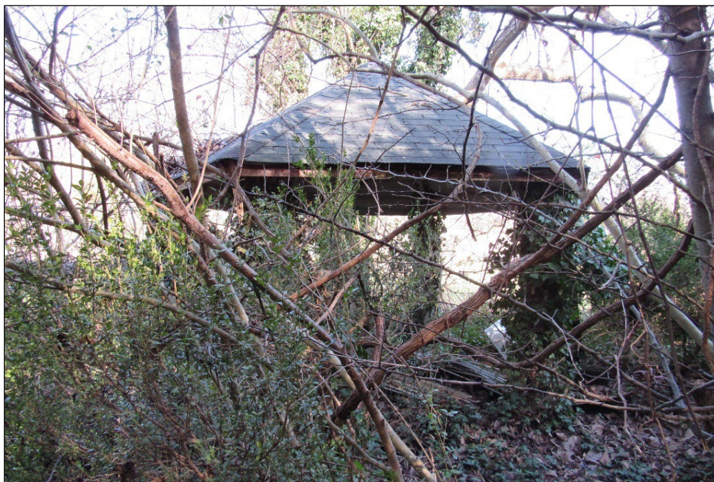
Photo 15: Early Twentieth-Century Gazebo/Tearoom, Looking North (Gordineer 2024).
